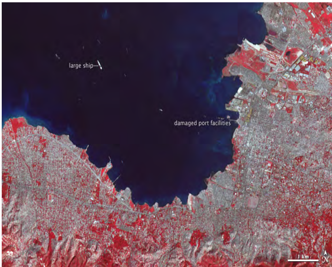
Figure 6. Damaged Transportation Infrastructure
