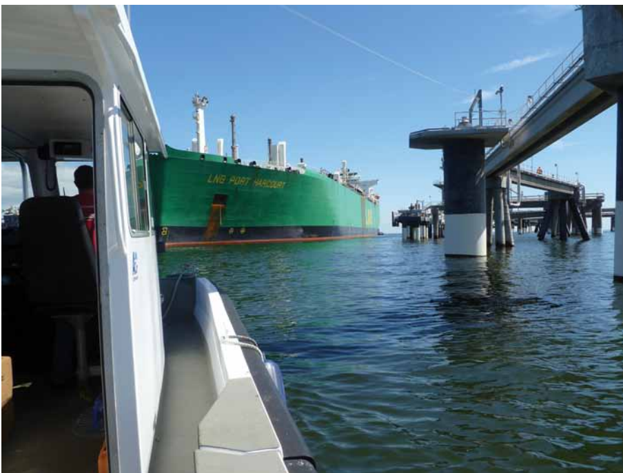
Berthing operations at the Cove Point LNG terminal in the Chesapeake Bay near Lusby, Maryland. Photo courtesy of Mr. Michael Gardner, Dominion Cove Point LNG.
