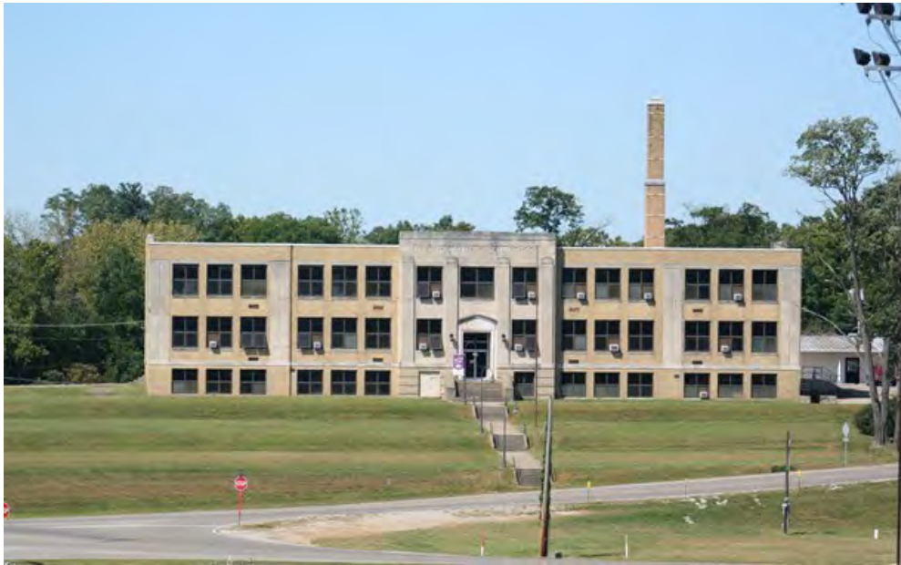
Figure 52. Union-Scioto Rural School, now the school district's administrative offices ( http://www.unioto.org/schools.aspx ).
