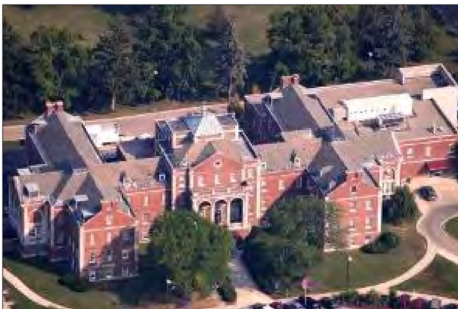
Figure 48. Chillicothe VA Medical Center, undated (Chillicothe VA Medical Center).
