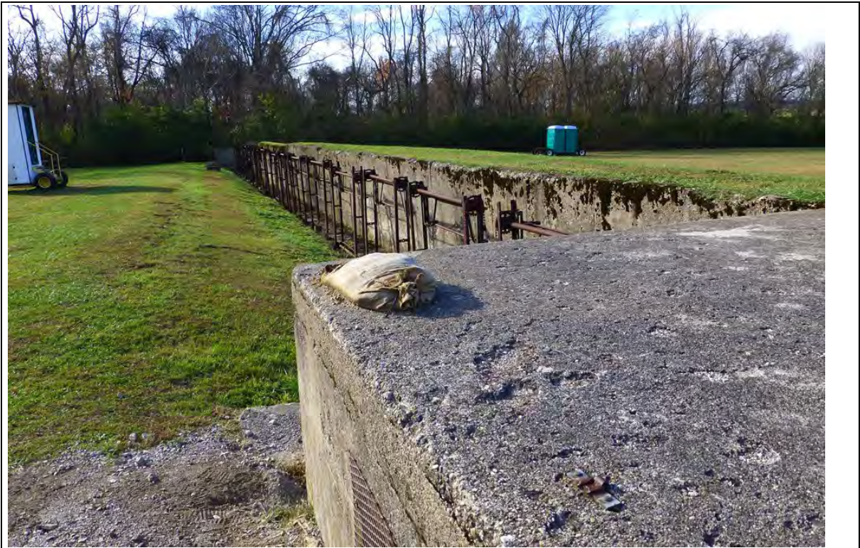
Photo 9. Former target butt (circa 1940), looking south (ERDC-CERL, 2015).
