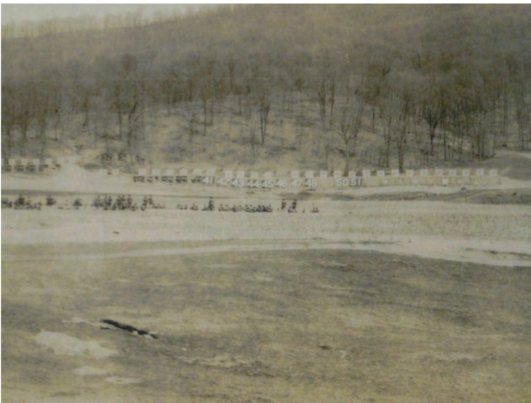
Portion of a panoramic view of the Camp Sherman Rifle Range, circa 1918 (courtesy of the Ross County Historical Society).
