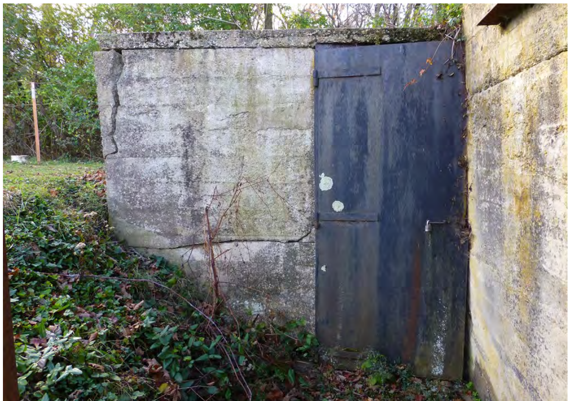
Photo 14. South target house storage door (circa 1940) (ERDC-CERL, 2015).
