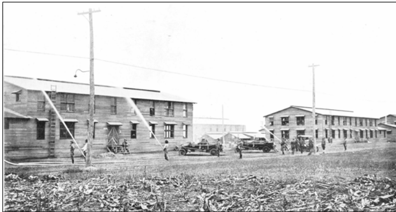
Figure 3. Example of two-story enlisted barracks at Camp Sherman ( National Army Cantonments 1918 ).
