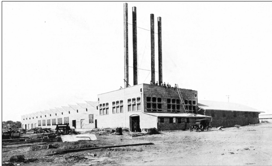
Figure 9. Camp Sherman laundry facility, 1918 ( National Army Cantonments ). The saw-tooth roof design is visible at the left side of this photo.
