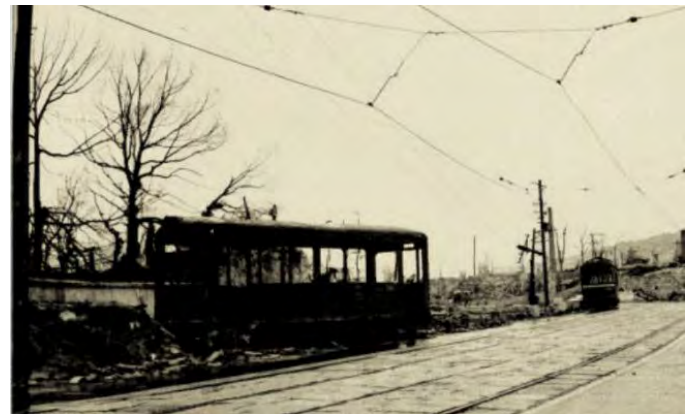
Fig. 9. Photo from Nov. 14, 1945 showing damage to the streetcar system, taken 3000 feet northeast of the hypocenter.
