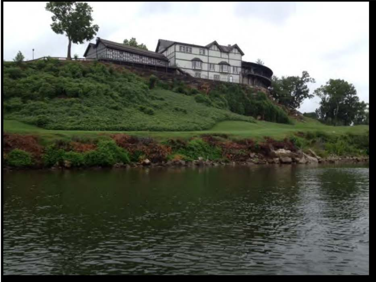
Figure 7 – Riverbank at Approximate TRM 466
