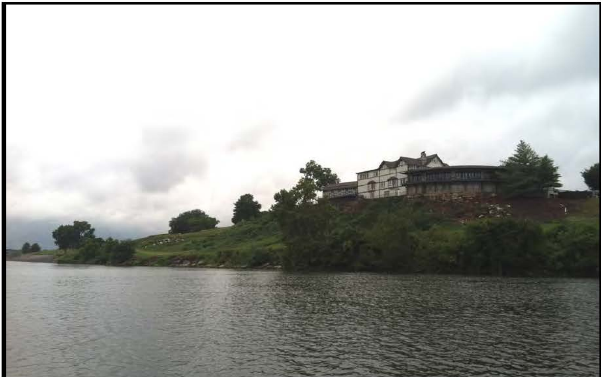
Figure 6 – Riverbank at Approximate TRM 466
