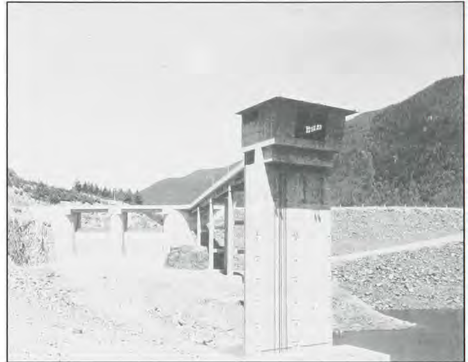
Howard Hanson Dam Construction
