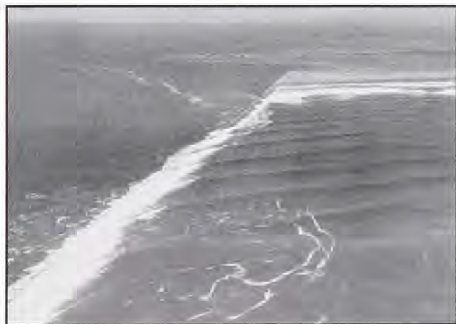
Grays Harbor, South Jetty Deterioration 30 January 1962
