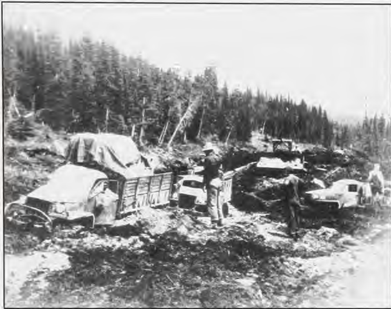
Alaska Canada Highway Construction, 1942
