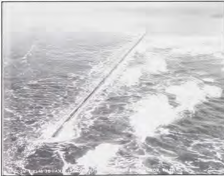
Grays Harbor, South Jetty
