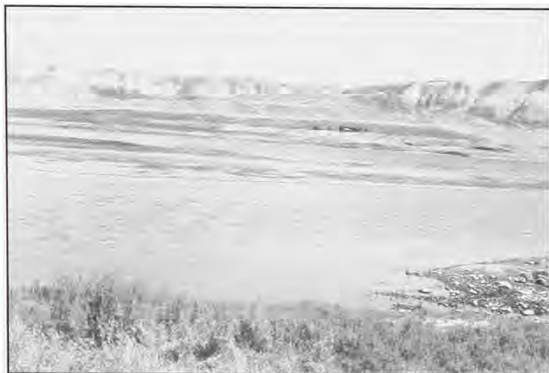
Ben Franklin Dam Site, Columbia River 6 Aug 1968
