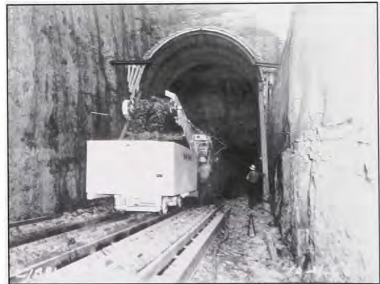
Great Northern Railway Tunnel Construction
