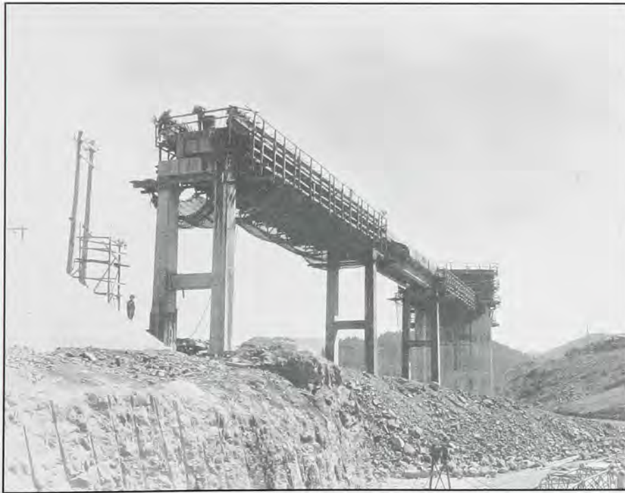
Howard Hanson Dam Construction
