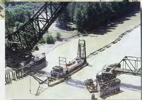
Pipeline dredges working on the Cowlitz River
