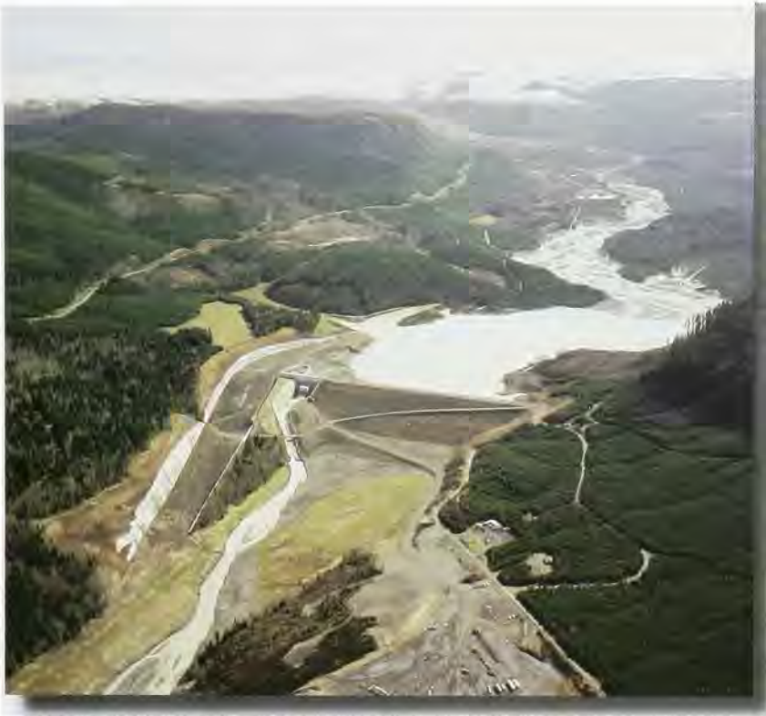
Completed Sediment Retention Structure (SRS)
