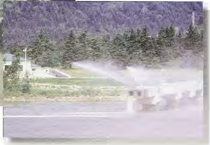
Bonneville Juvenile Transport System and monitoring facility. The outfalls have spray jets of water to deter gulls, terns, and other birds from feeding on the salmonids.
