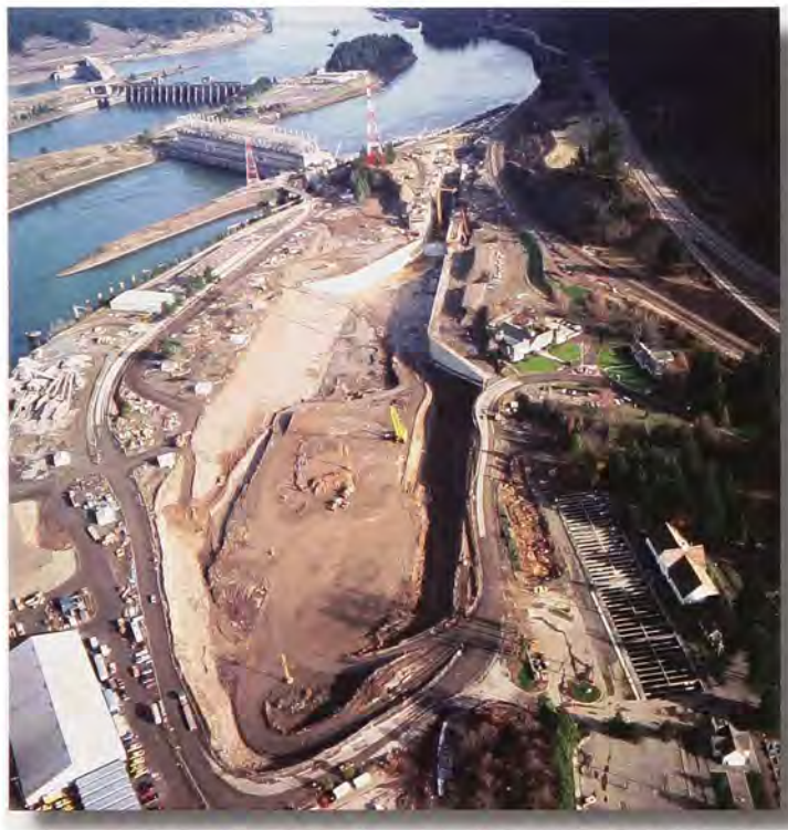
Using RCC application on the downstream guide wall decreased the construction time on the navigation lock. These photos show working on the tunnels for filling and emptying conduits and designing the concrete swing bridge.
