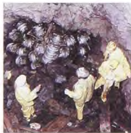
TBM BREAKING THROUGH THE SPIRIT LAKE TUNNEL
