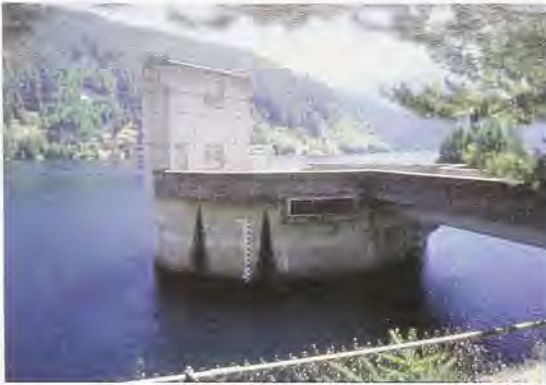
Cougar Dam reservoir water temperatures will be regulated through a temperature control tower.
