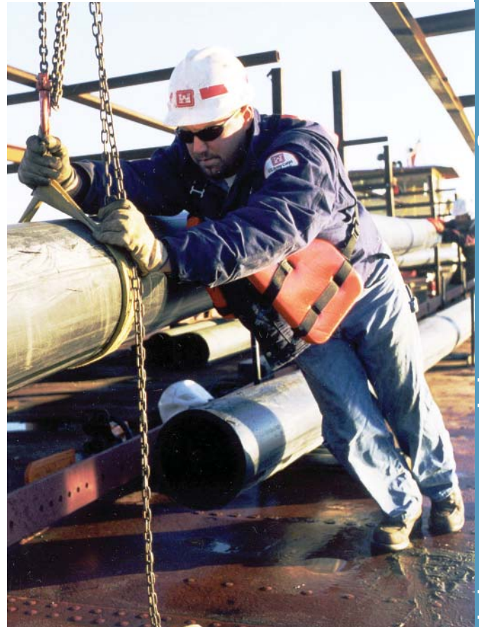
Dredging the Mississippi River: J. Skrede, a member of the crew on the Dredge Dubuque, positions pipe that will carry dredge material. (Photo courtesy of, St. Paul District, Corps of Engineers)
