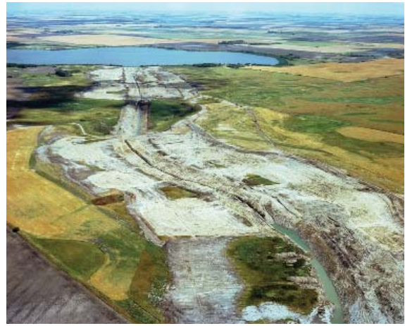
Devils Lake: A flood control diversion channel constructed by the North Dakota State Water Commission in the northeastern part of the Devils Lake watershed. (Photo by Lyle Nickly, courtesy of St. Paul District, Corps of Engineers)
