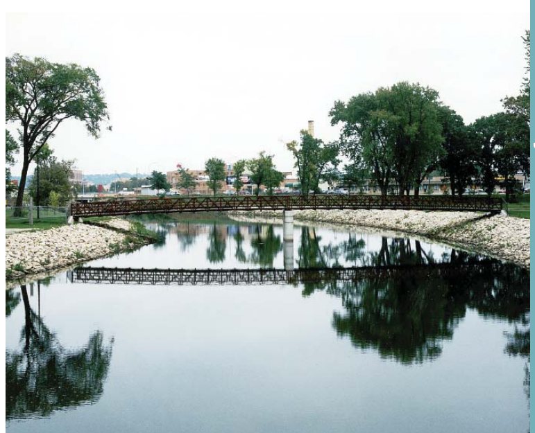
Zumbra River: Channel modifications on the South Fork Zumbro River in Rochester, Minnesota, showing the pedestrian bridge and riprap implemented by the St. Paul District, 1995. (Photo courtesy of St. Paul District, Corps of Engineers)
