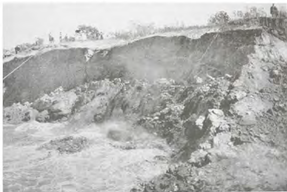
Caving bank on the Mississippi River.
