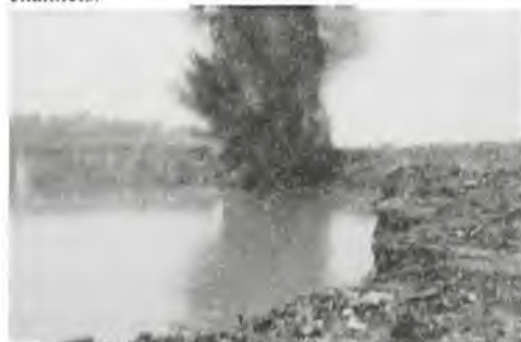
Dynamite removes the plug and opens the cutoff.
