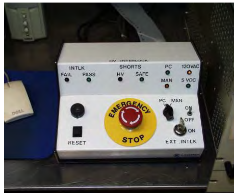
Figure A.46. Safety Interlock System
