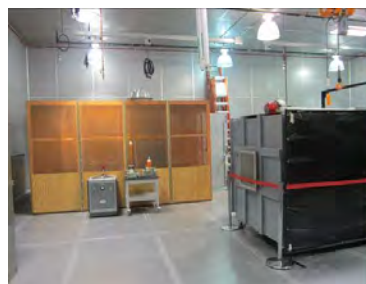
Figure A.66. High Bay (View B)
