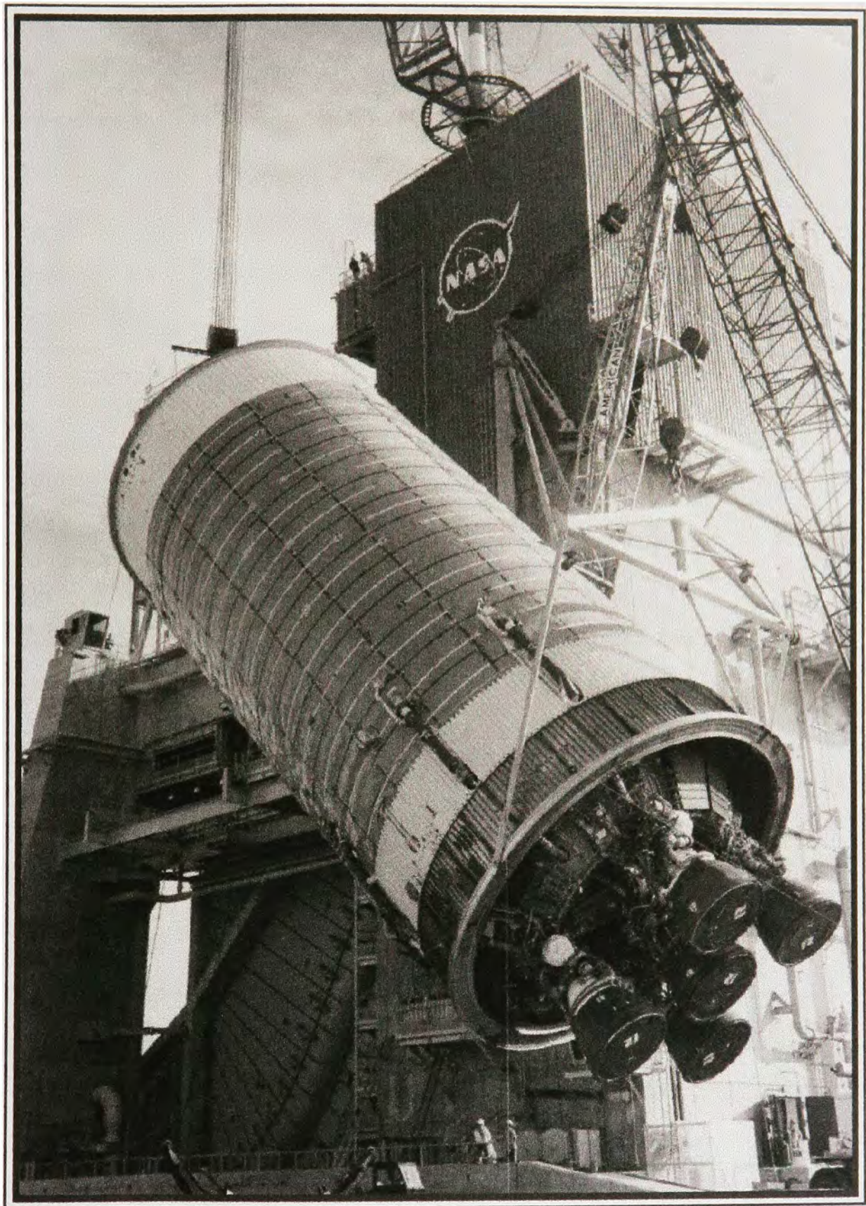
Figure 13-10. Cranes lifting the Saturn rocket booster for placement in the test stand at MTF (Public Affairs, MDO).
