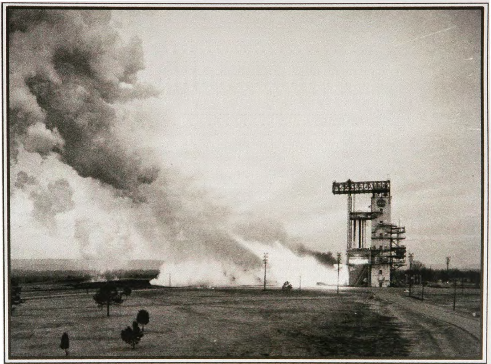
Figure 13-3. Test firing the first stage of the Saturn V rocket, Marshall Space Flight Center, Huntsville, Alabama (Public Affairs, MDO).
