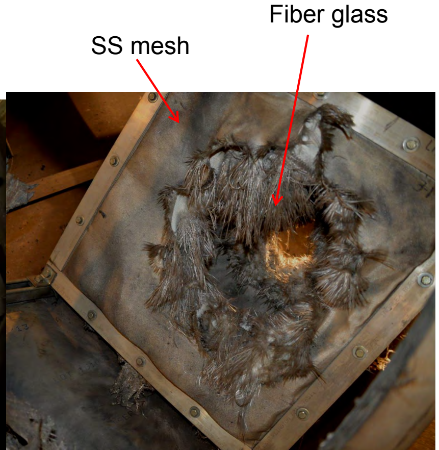
Back side of 3 rd bumper. Note that fiberglass protrudes through SS.
