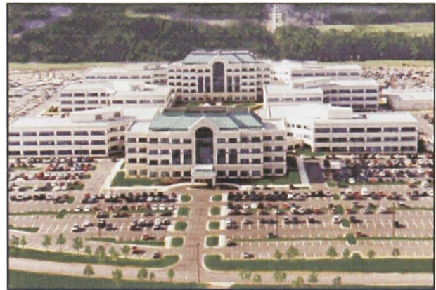
Completed Sparkman Center at Redstone Arsenal.
