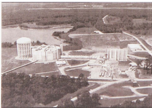
Overview of the completed J-6 facility.
