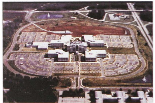
The Sparkman Center at Redstone Arsenal, Alabama.
