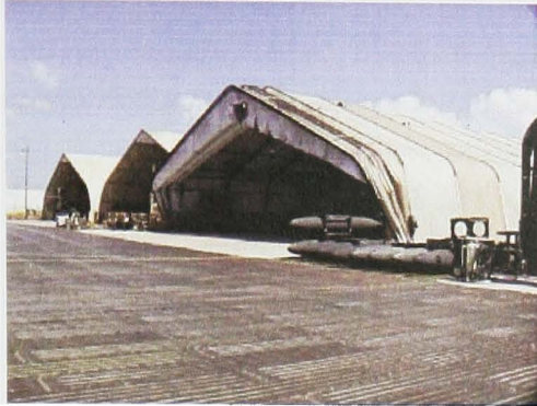
The District work at Soto Cano Air Base, Honduras.
