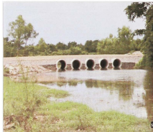
Water control bridge for a USAID bridge project in Honduras.
