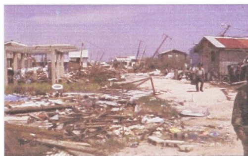
Damage done by 1986 earthquake in El Salvador.
