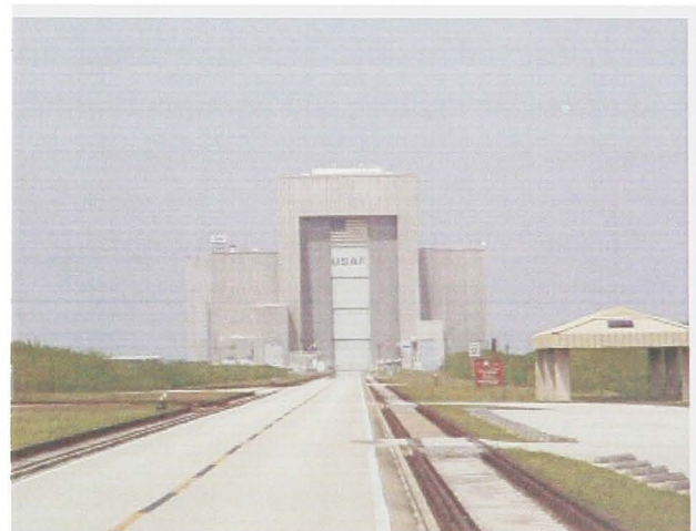
Solid Motor Assembly Building at Cape Canaveral.
