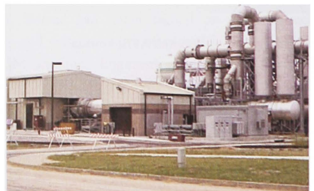
View of the Navy Large Engine Test Facility (photo courtesy of Arnold Engineering and Development Center).
