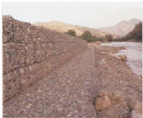
Erosion control in Bolivia.
