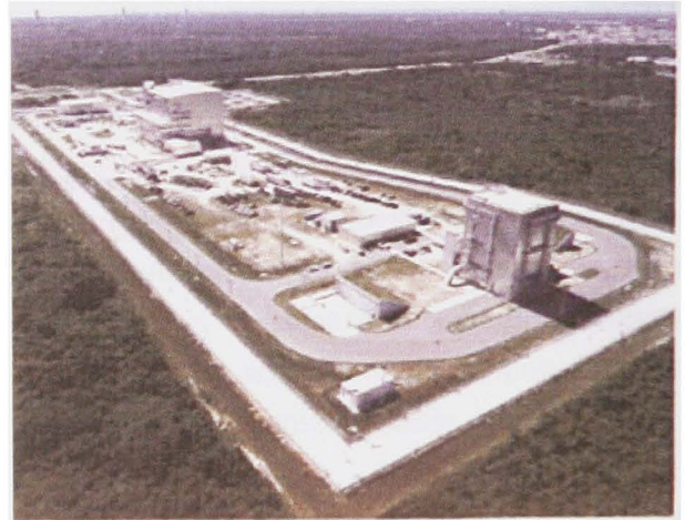
The Centaur Tanking and Processing Facility.
