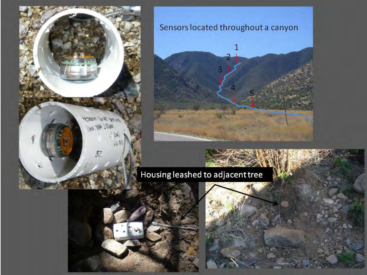
Plate 1.2. Illustration of electrical resistance sensor installation. Sensors are shallowly buried in the streambed along a gradient of hydrologic flow regimes (perennial, intermittent, ephemeral) within a canyon.
