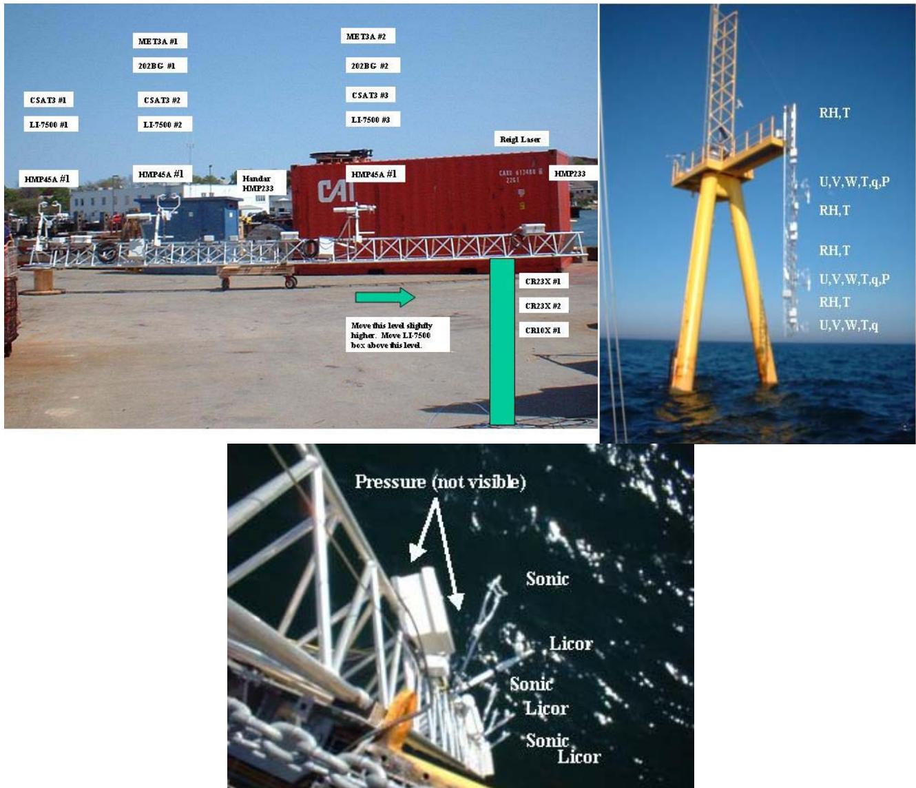
Figure 1. The CBLAST instrument mast partially assembled with four pressure sensors at the Woods Hole Oceanographic Institution (upper left photo) and the mast installed at WHOI's Air-Sea Interaction Tower (upper right and lower photo). Photographs courtesy of Dr. Jim Edson.
