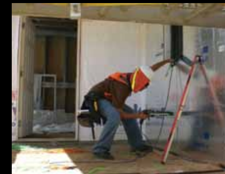
Demonstrated at Aliamanu Military Reservation, radiant barriers are an alternative to conventional insulation used in houses. These barriers reduce summer heat gain and winter heat loss, making military houses more energy efficient.
