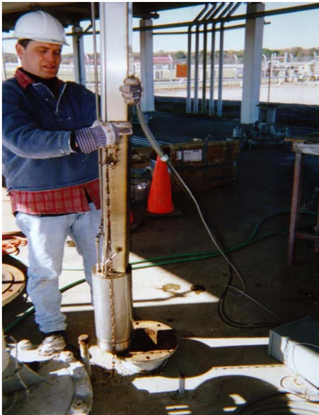
Figure 17. Installation of the LRDP in the 50,000-gal UST.
