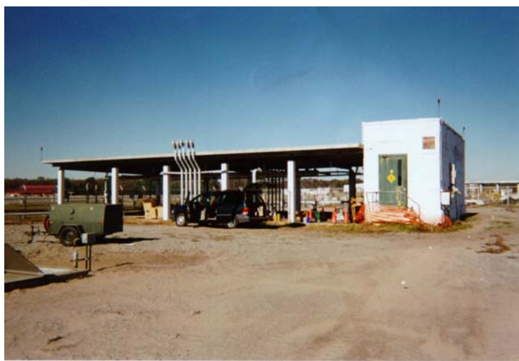
Figure 14. Tank 45 at the Hunter Army Airfield.
