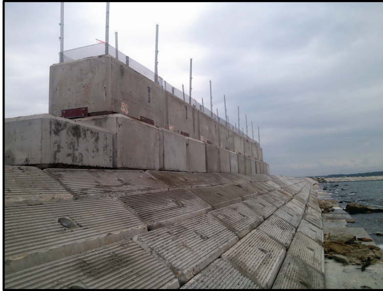
Figure 2. Nesting habitat blocks installed on the Ashtabula breakwater. Toe blocks are at the far right of the breakwater at water level.
