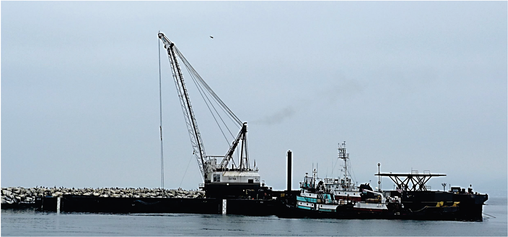
Figure 12. Dredge Barge, Scow (foreground left) and Tugboat, Marina del Rey, April 30, 2012.
