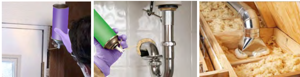
Figure 7. One-component spray polyurethane foam application options (from American Chemistry Council Inc., 2015d).
