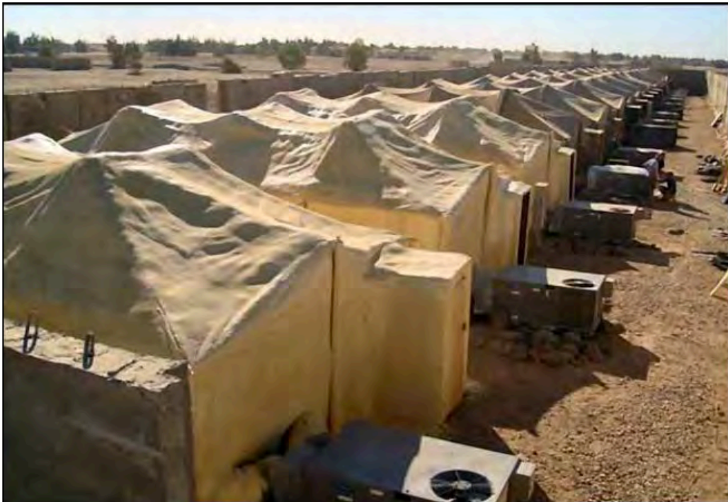
Figure 11. Foam insulation applied to tents in Kuwait (from AFCESA, 2010).
