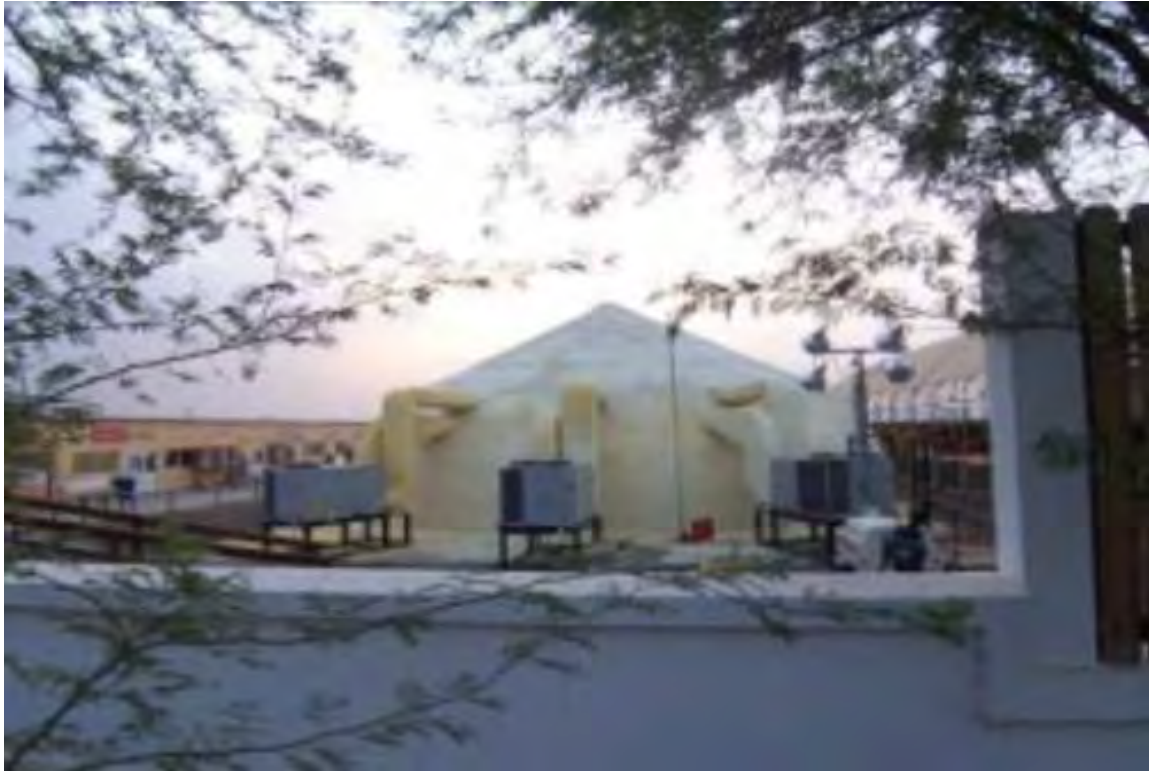
Figure 12. Exterior foam application to Camp Lemonnier Gym, Djibouti (from Nolan, 2015).
