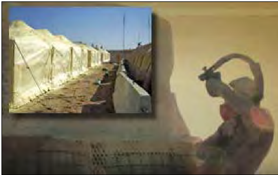
Figure 13. Honeywell employee applies terra strong foam to structures in Iraq (from Urethanes Technology International, 2009).
