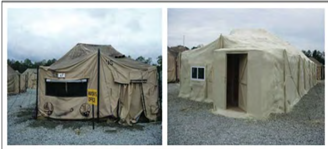
Figure 10. GP-L tent before and after external application of spray foam insulation, Fort Benning, Georgia, 2007 (from GAO, 2009).
