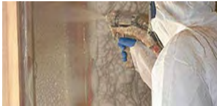
Figure 8. Open-Cell Spray Foam (from EPA, 2015a).
