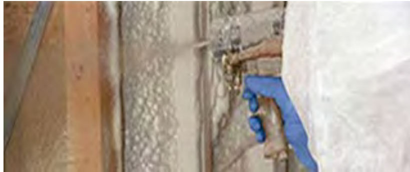
Figure 9. CCSF two-component, professional, high-pressured system foam application (from EPA, 2015a).
