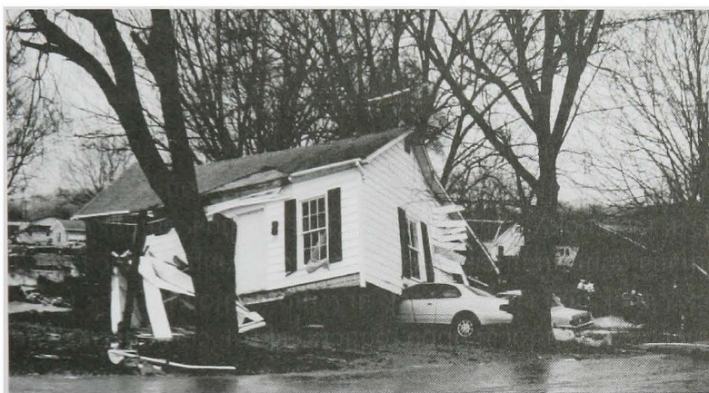
Flood damages, Falmouth, KY 1997
