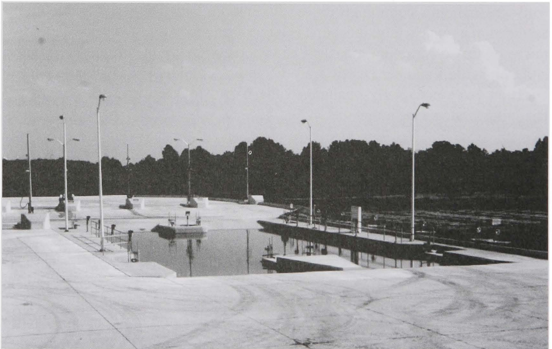
Vehicle Wash Rack, Fort Campbell, KY
