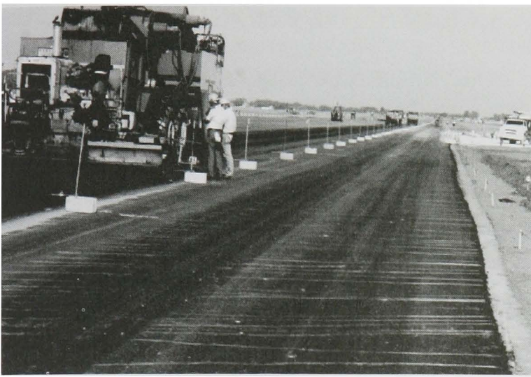
Airfield Paving, Fort Campbell, KY
