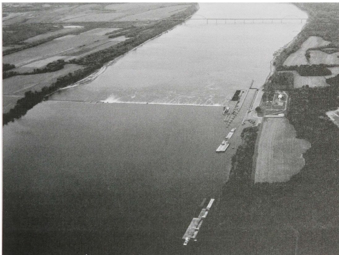
Locks and Dam 52, Ohio River Mile 938.9
