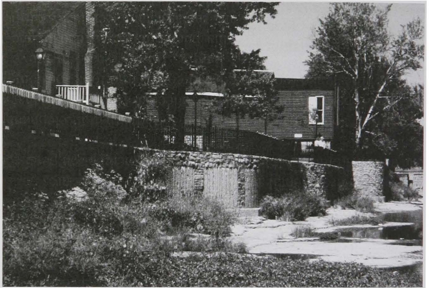
Perryville, Kentucky, Local Protection Project
