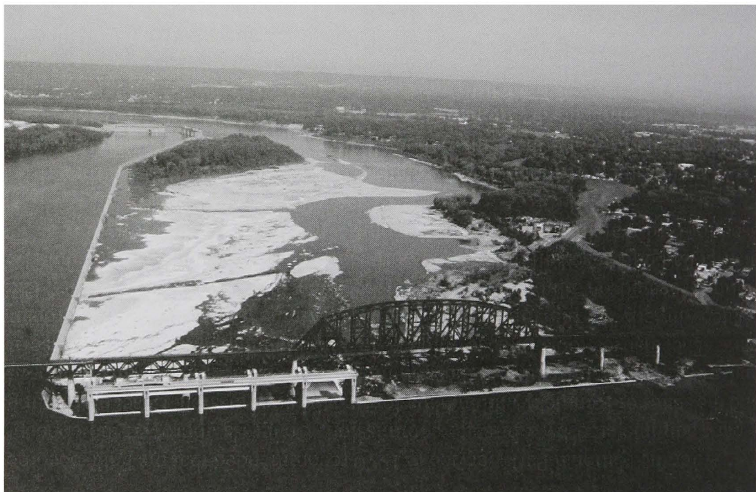
Falls of the Ohio, below upper gates, McAlpine Locks & Dam
