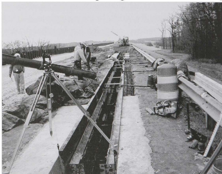
Mississinewa Dam repair
