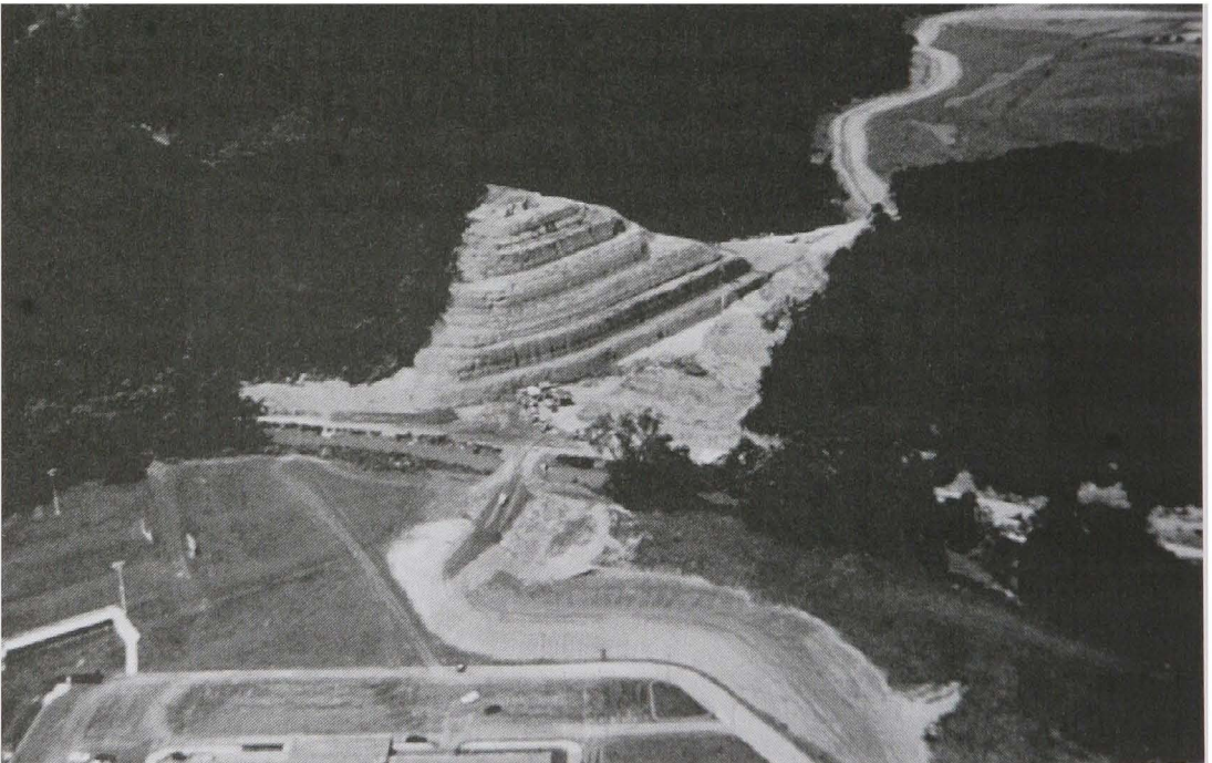
Salyersville, KY, Flood Protection Project
