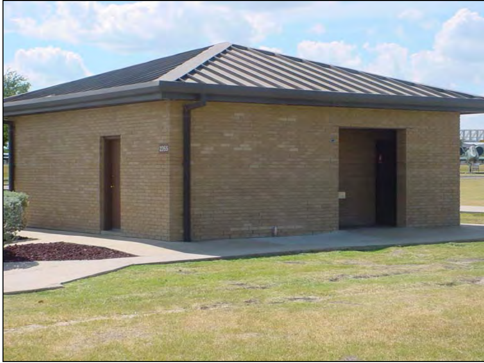
Photograph 7: Example of the Restrooms
