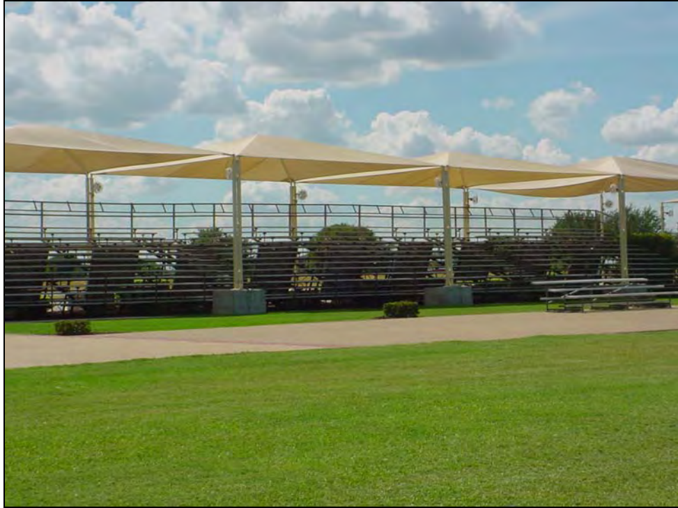
Photograph 5: Example of Front View of Bleachers
