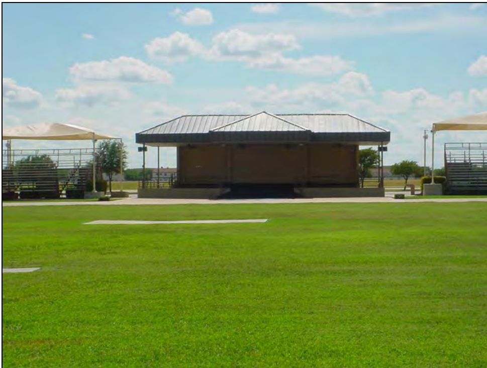
Photograph 4: Example of Front view of the Reviewing Stand
