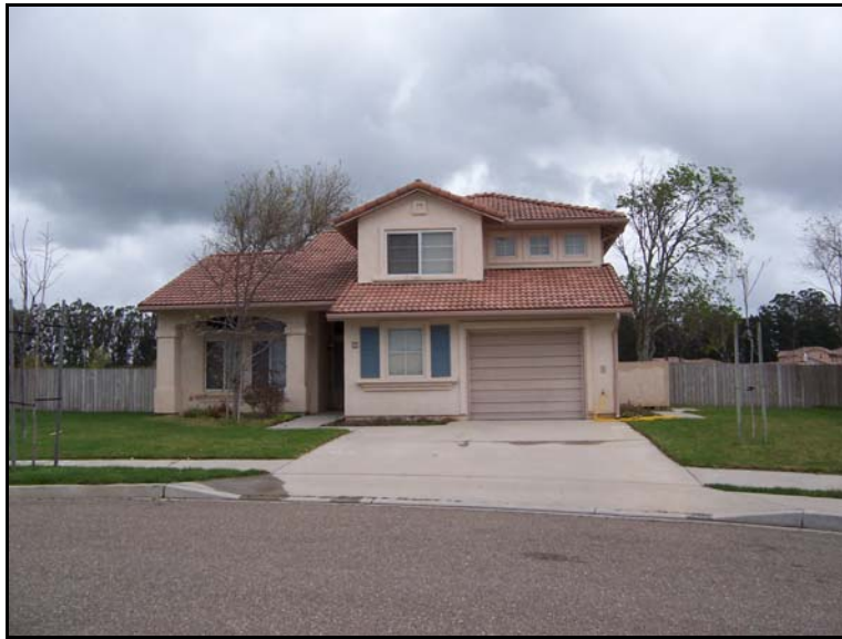
Figure 1-5 Example of a 3- to 4-Bedroom MILCON Replacement Unit in the West Housing Area
