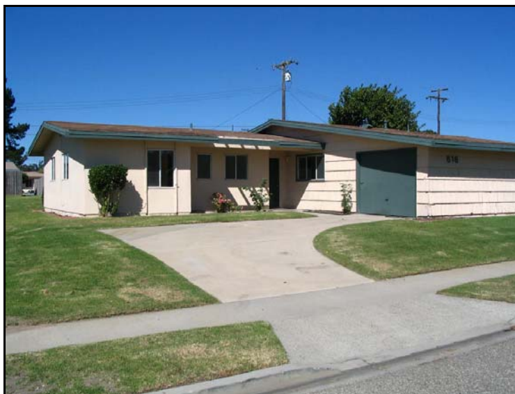
Figure 1-3 Example of a 3-Bedroom Capehart Housing Unit in the West Housing Area
