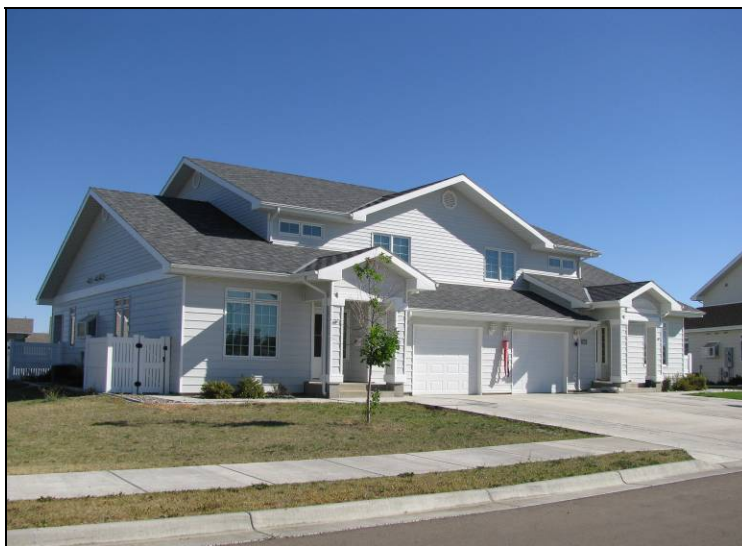
Figure 2-3. New Housing Constructed via MILCON
