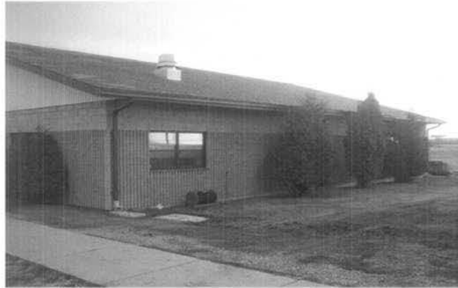
Existing CATM Building Figure 1-2
