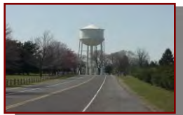
Water Tower Replacement
