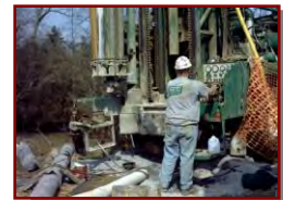
Refurbishment to lift stations
