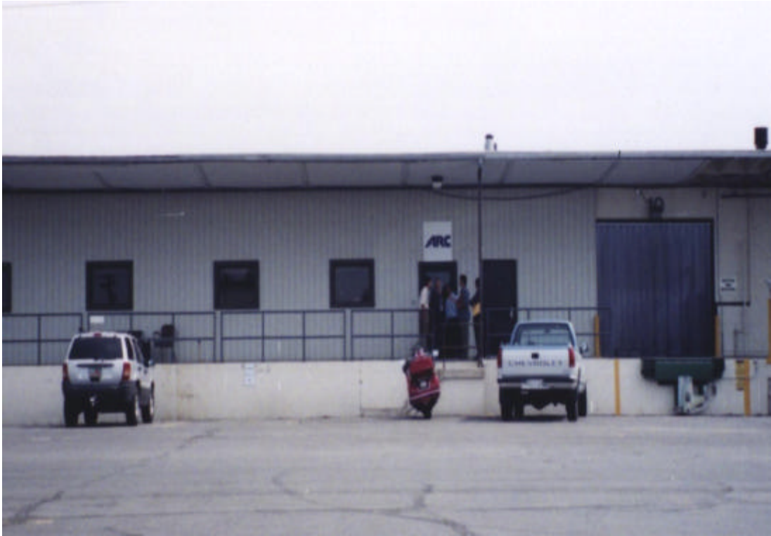
Photo 7: Contractor Facilities at Freeport Center.
