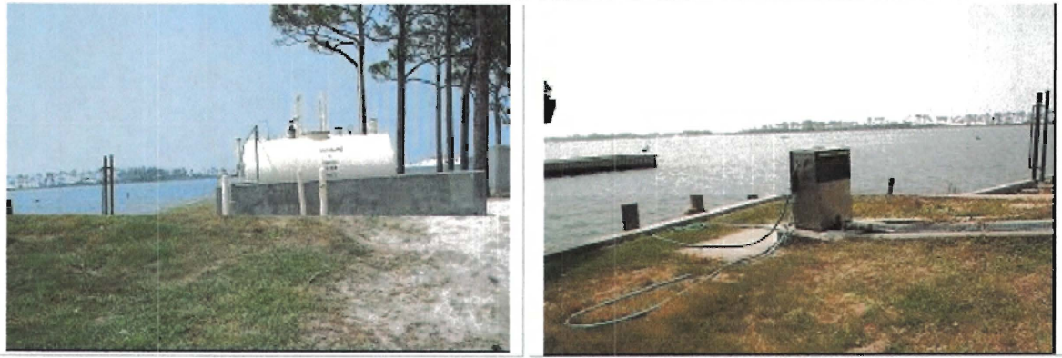
Figure 1-2. Existing fuel storage and dispensing system.
