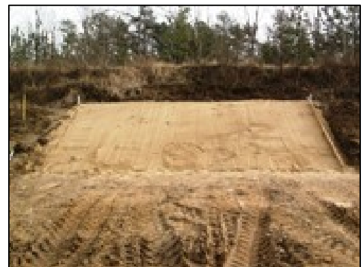
3. Berm Grading Complete
