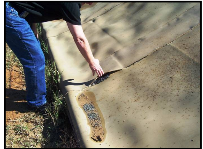
Loose top rubber cover seam
