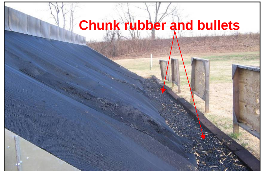
Degradation of the bullet trap, including the forward kick out of rubber and bullets
