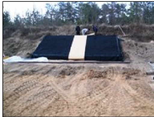
5. Applying Top Cover
