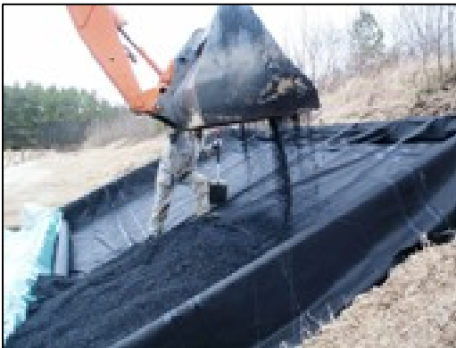
4. Adding Granular Rubber
