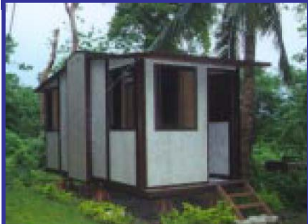
Storage Sheds and Emergency Shelters
