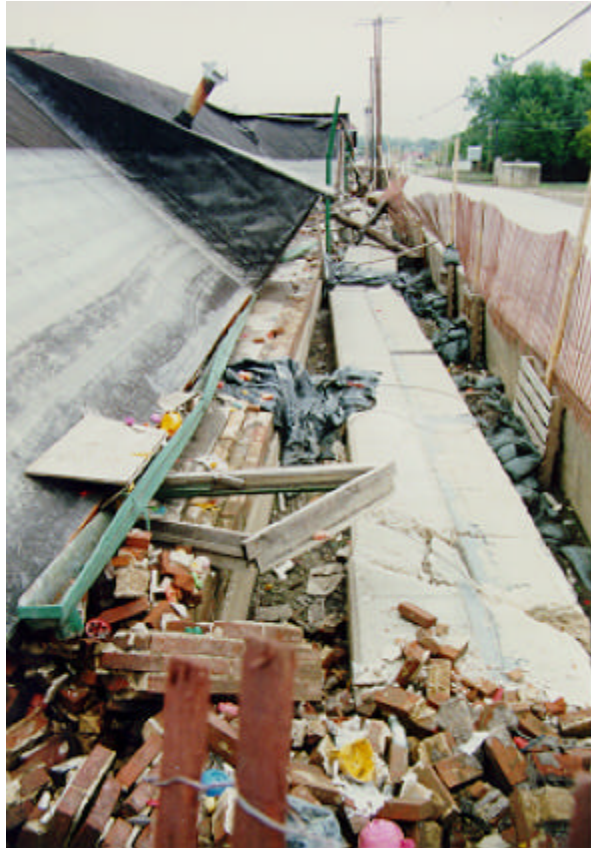
Looking at the collapsed floodwall additions. Note these two additions are still tied together with rebar.
