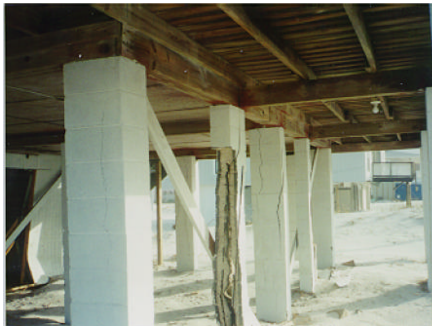
Looking at the column support that was nearing failure.
