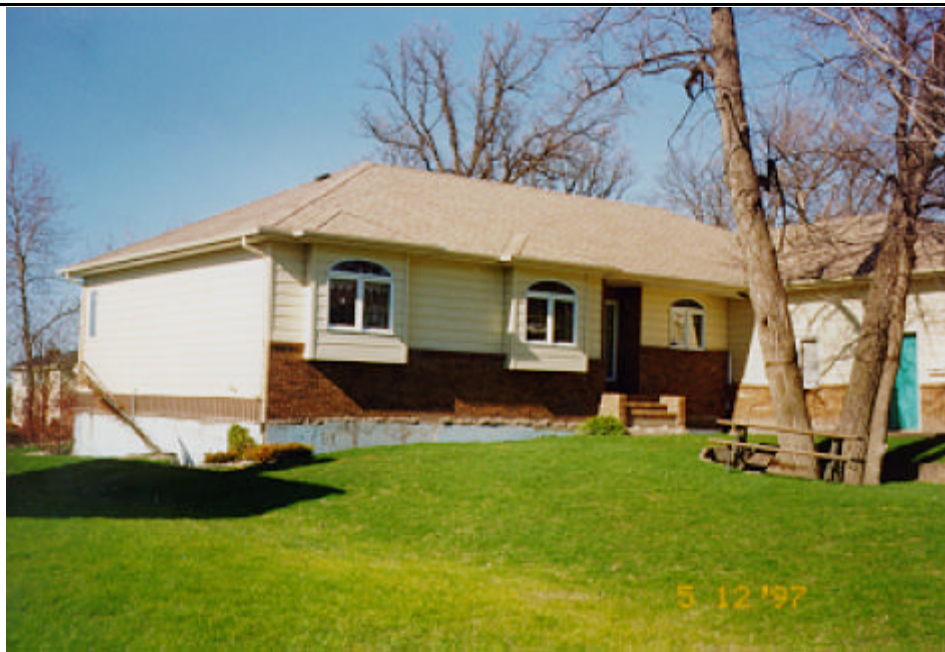
Looking at the structure. Note the garage on the right that held that part of the structure down and the exposed basement wall on the left indicating the amount of lifting that occurred on the west side.
