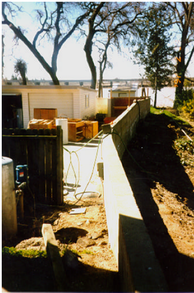
Looking along a portion of the floodwall. The failure under the wall occurred in the immediate foreground. Note the largest closure at the right of the structure. Also note the Sacramento River in the background.
