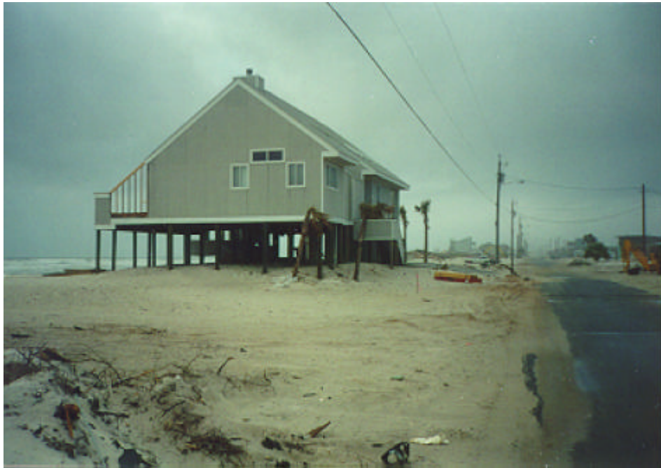
Looking at the structure. Note the beach at the left. Note also the absence of adjacent structures, which had been destroyed and removed.
