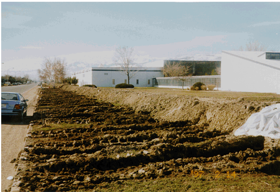
Looking at the recently constructed earthen embankment protecting Structure 95. Note the plastic sheeting at the far right that was placed over the embankment's unprotected side and held in place with sandbags to provide impermeability to the embankment.
