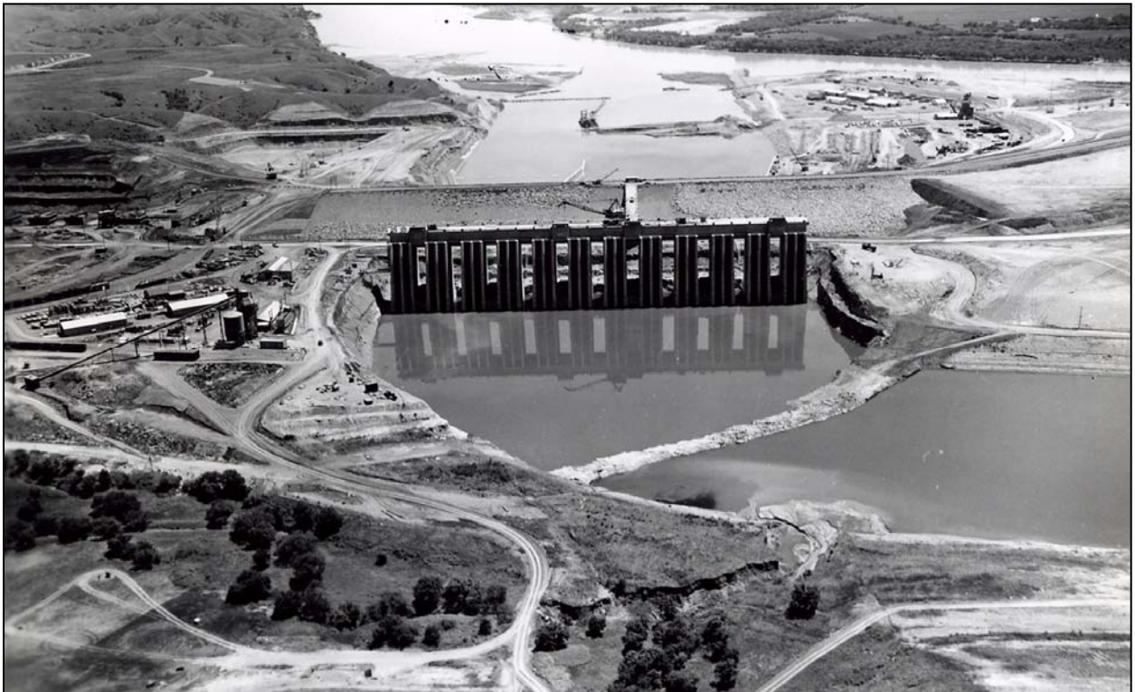
Photo 1.4. Aerial view of intake structure at Fort Randall Dam after initial release of water through river plugs in the coffer dam ( Photo Date: 5-Jun-1952 ). It is believed the coffer dam was later removed.
