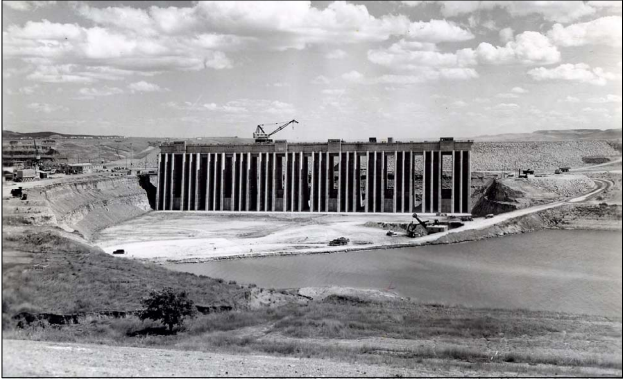
Photo 1.3. General view of upstream face of intake structure at Fort Randall Dam, after final cleanup of approach area, and before release of water through river plugs in the coffer dam ( Photo Date: 27-May-1952 ).
