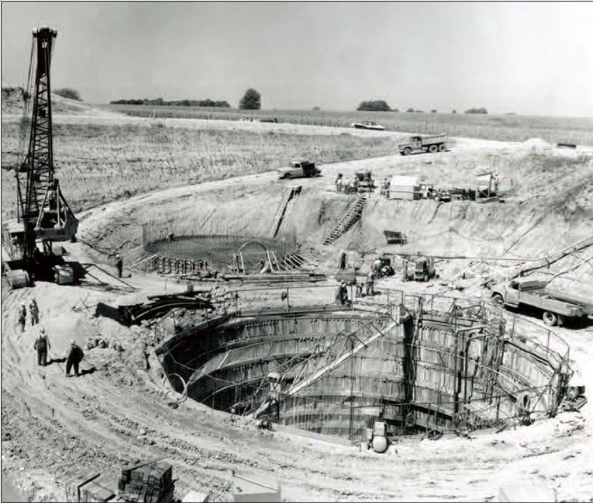
Construction of silos for the Atlas ICBM missiles took place on the prairies and high plains of the Midwest and West. The Omaha District built the nation's first operational Atlas launch facilities in silos surrounding F. E. Warren Air Force Base near Cheyenne, Wyo.
