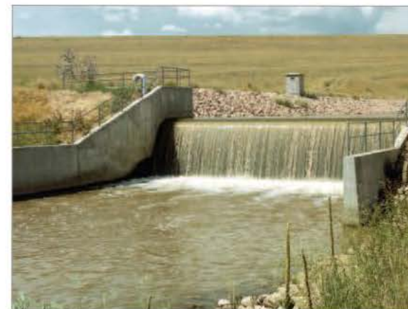
Bear Creek Spillway
