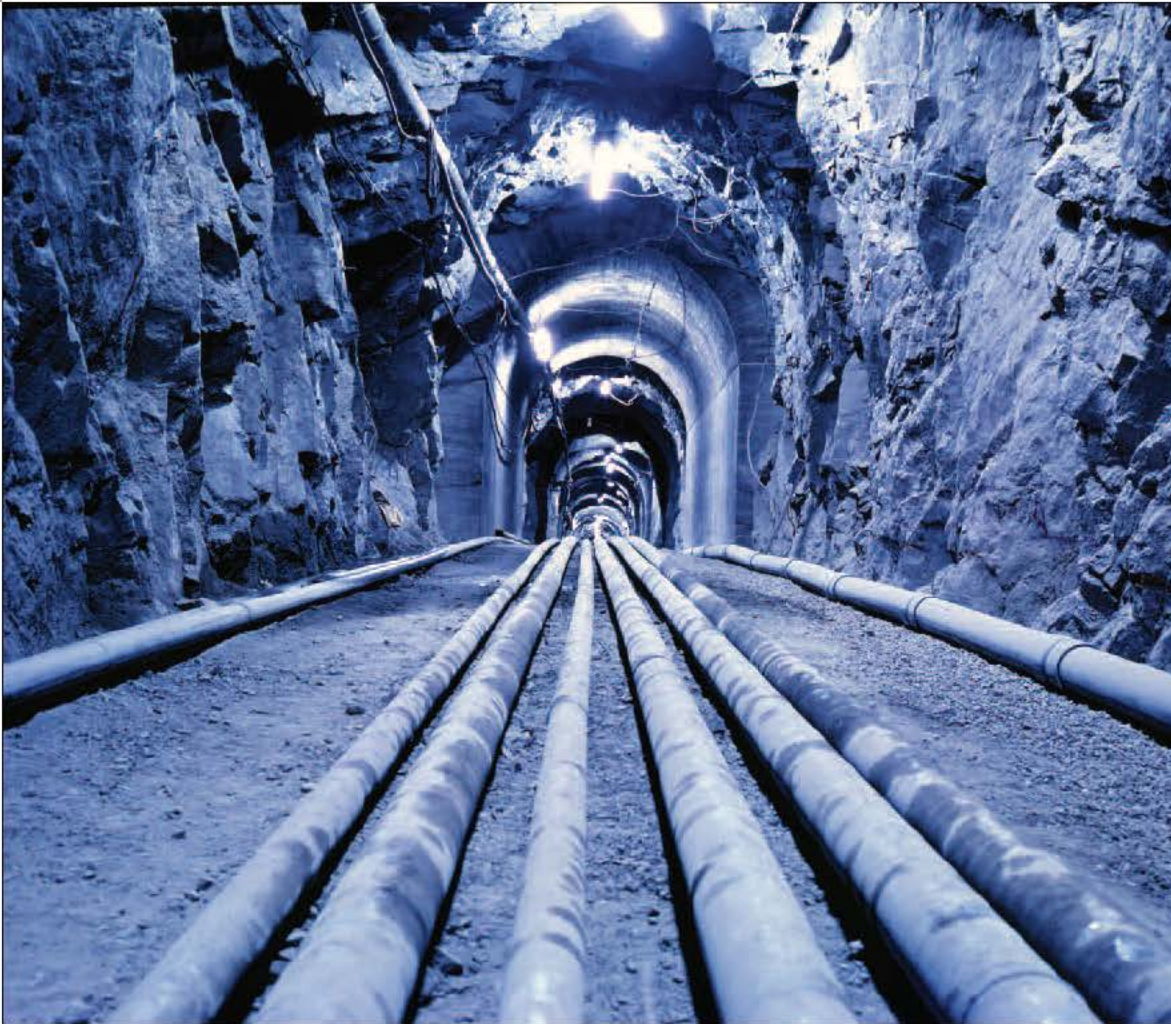
Truck-size tunnels and building-size chambers were blasted from granite for NORAD in one of the district's great engineering and construction project achievements. The district continues to perform engineering work for NORAD.
