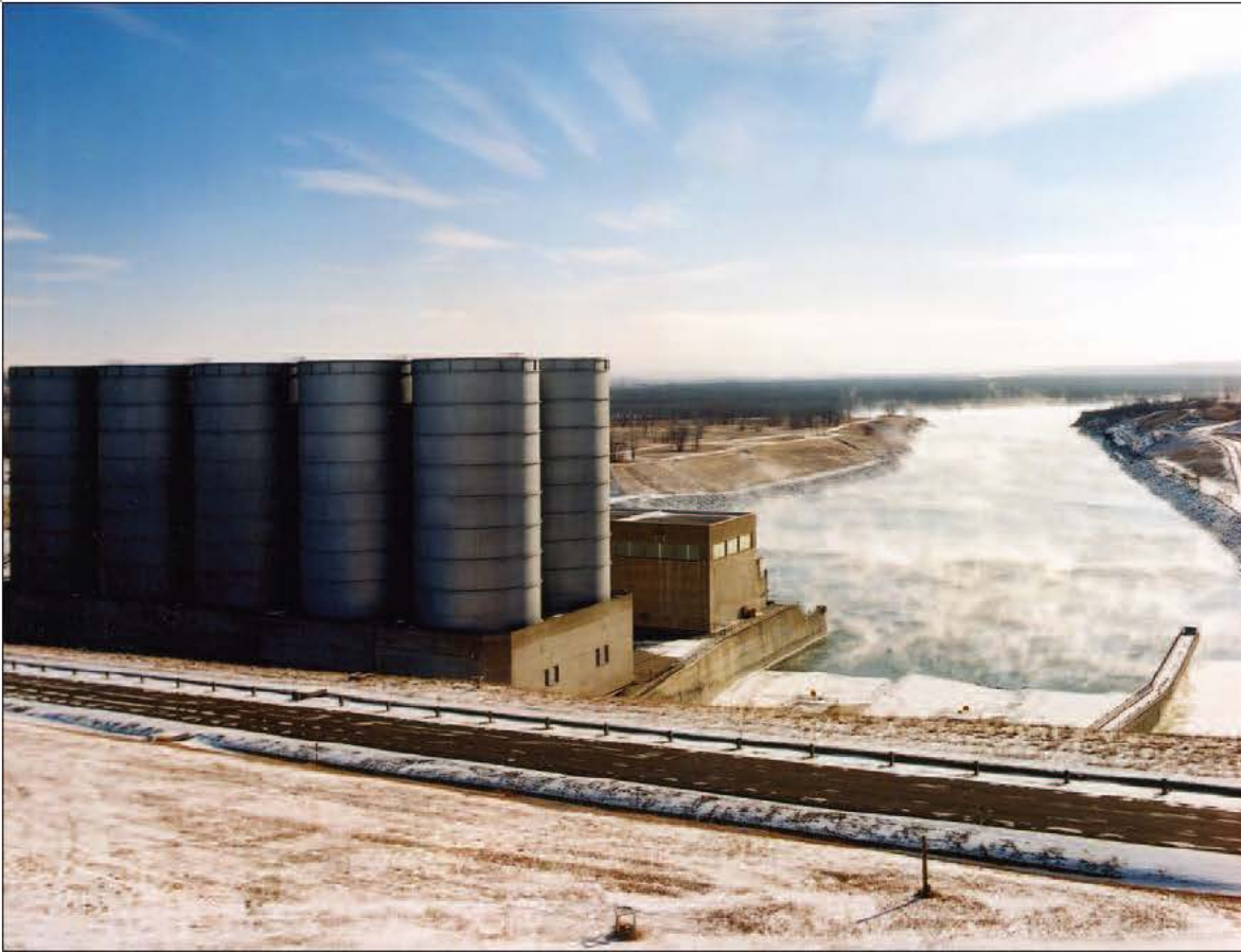
The Garrison Dam Powerhouse houses five generating units that produce an annual average 2.6 million mega-watt hours of electricity. This translates into a value in excess of $25 million in revenue.
