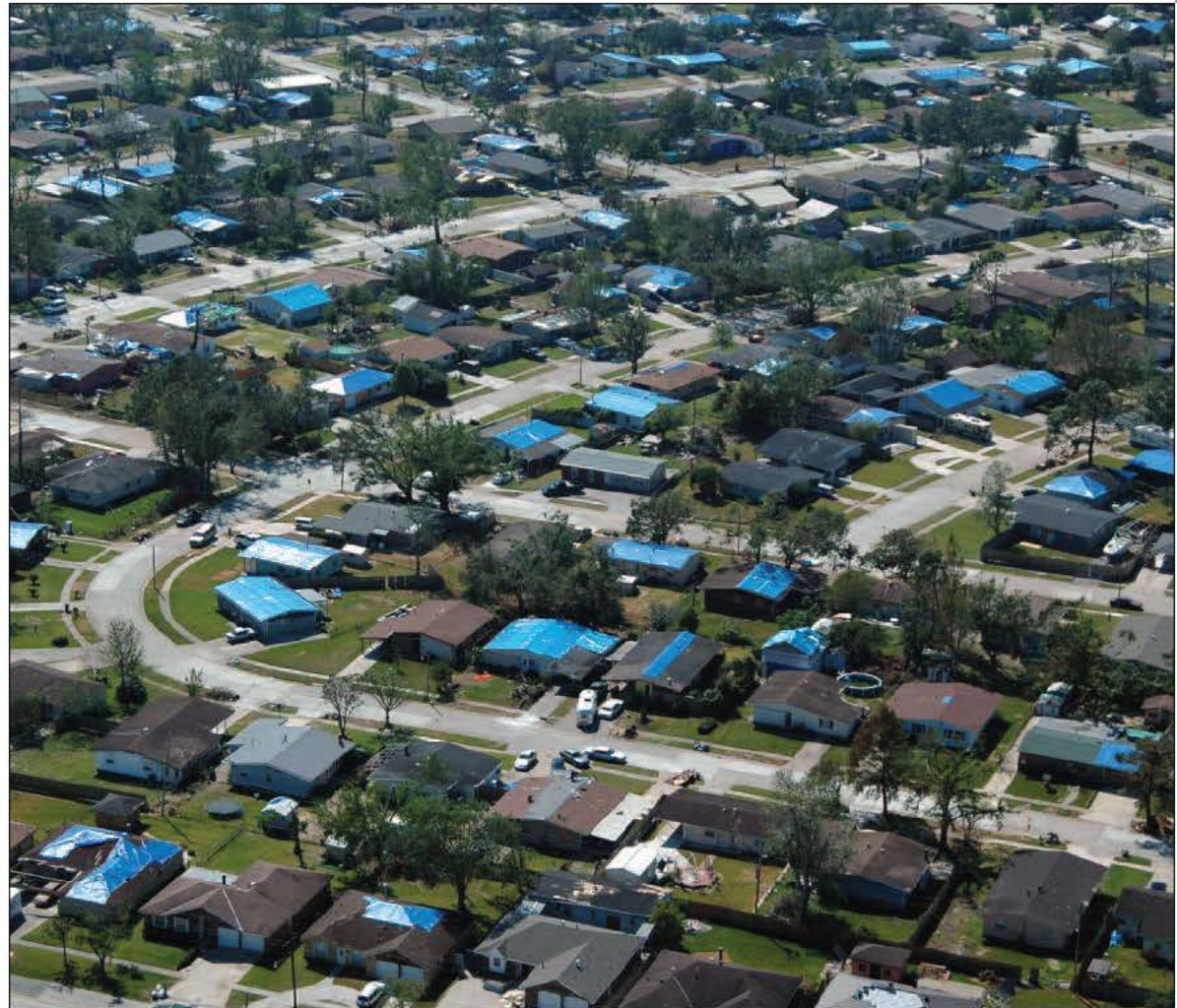
In the aftermath of major natural and man-made events, response teams such as the "Blue Roof" teams are a part of the Federal Emergency Management Agency mission to respond to local communities devastated by such storms. (Photo provided.)
