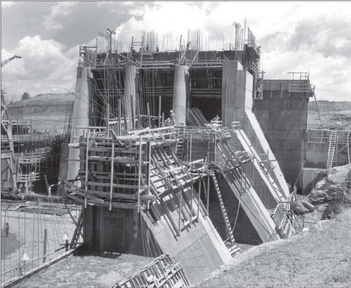
Many workers who built the Big Bend Dam spillway came from missile jobs in Nebraska. Work on the powerhouse substructure alone involved as many as 1,300 workers, including up to 600 carpenters.
