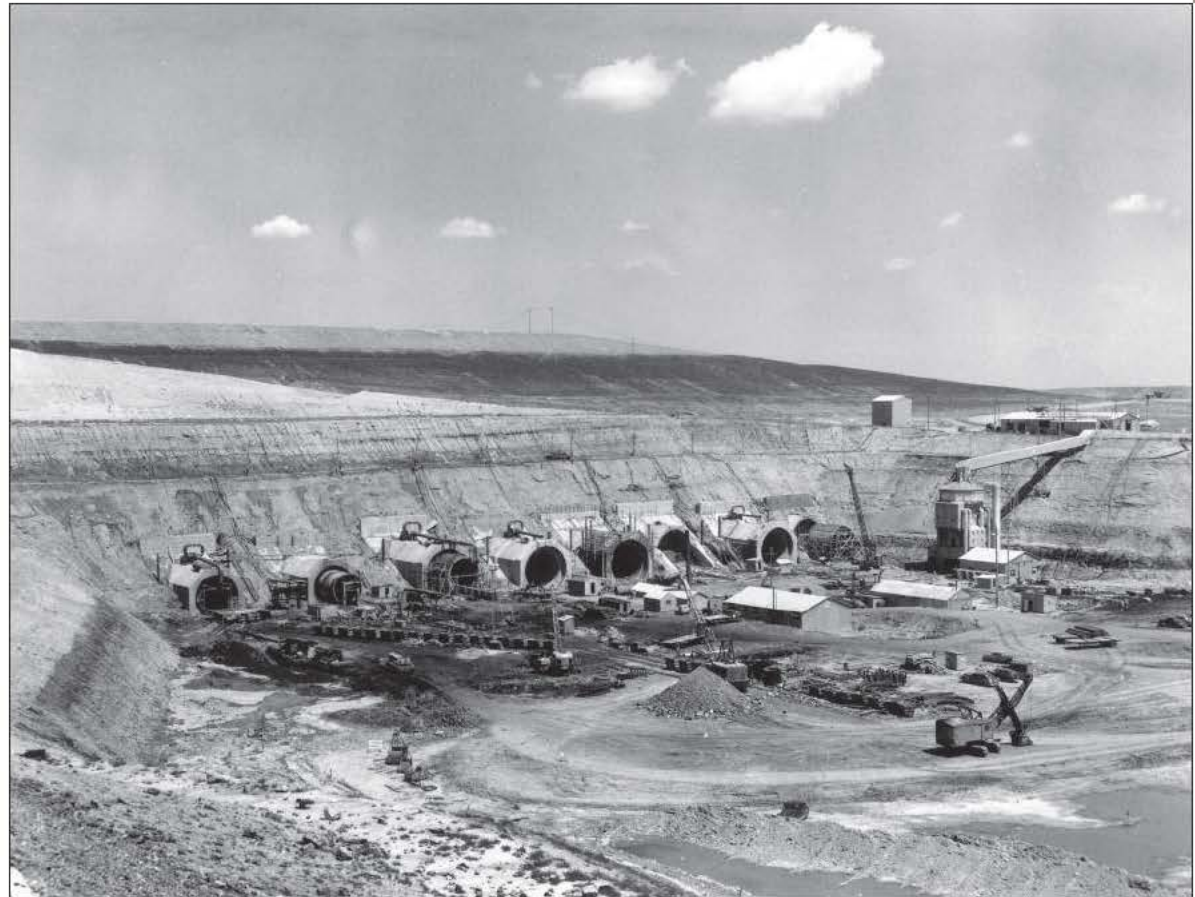
Work on the Garrison Dam involved new drilling techniques, specially made equipment and innovative approaches to construction. (File photos.)
