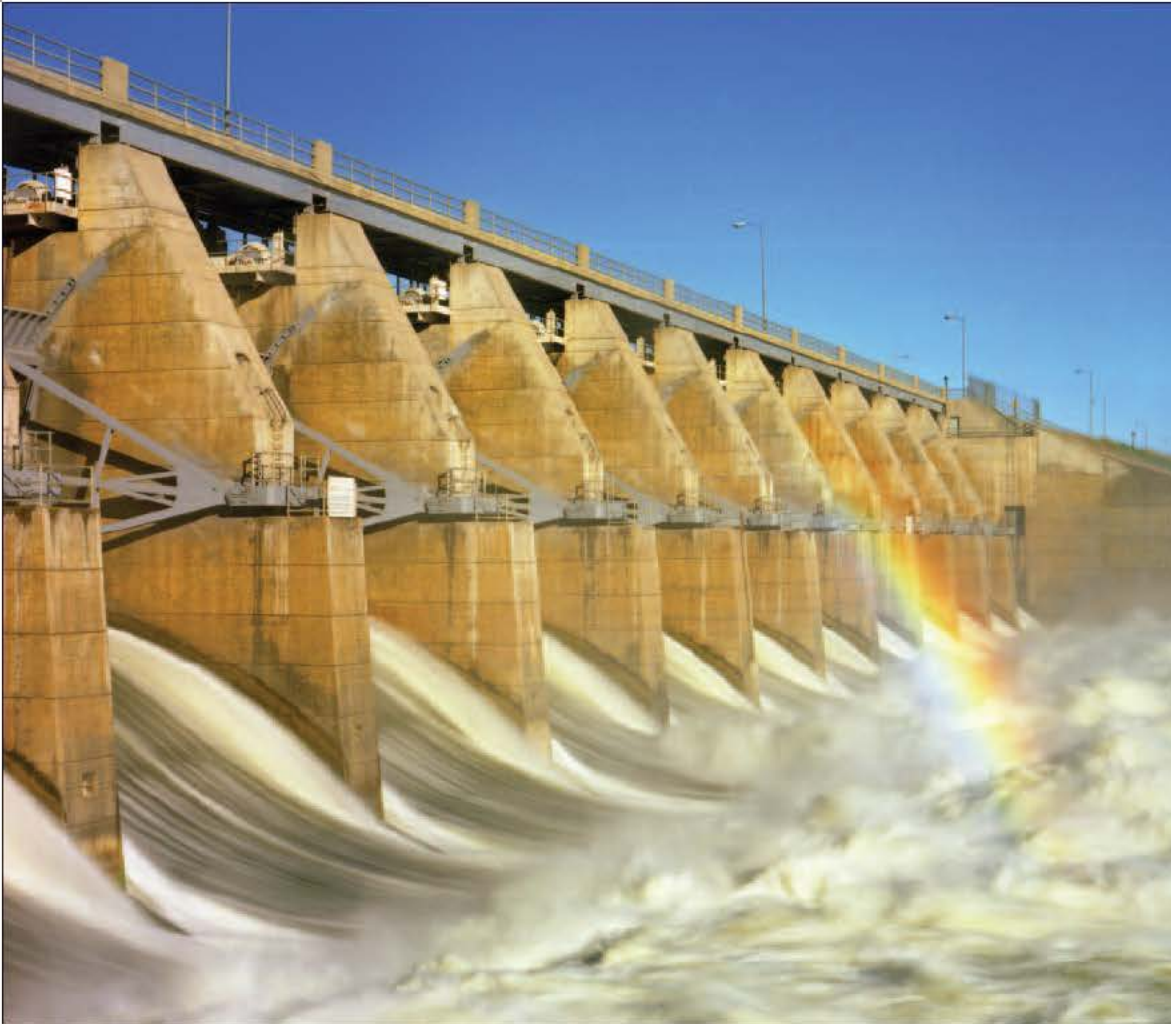
Water released from the five upstream dams is used at Gavins Point for producing hydroelectric power. Controlled releases from the dam enhance navigation and minimize erosion on the Missouri River to St. Louis, Mo.
