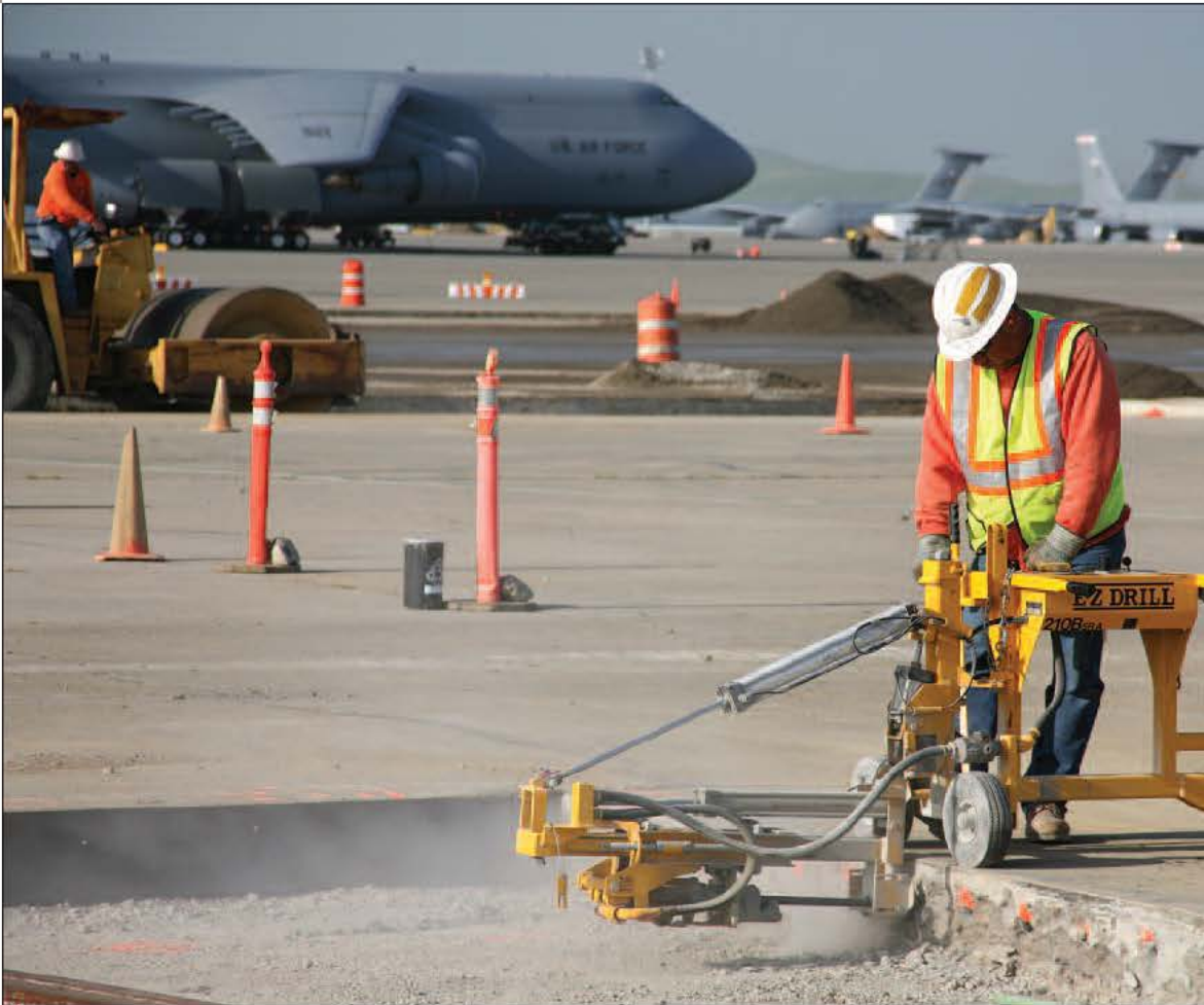
One of the Centers of Expertise in the Omaha District is the Transportation Systems Center. Other branches of the military tap the District to help with technical review, quality control and training for airfield, railroad and roadway projects.
