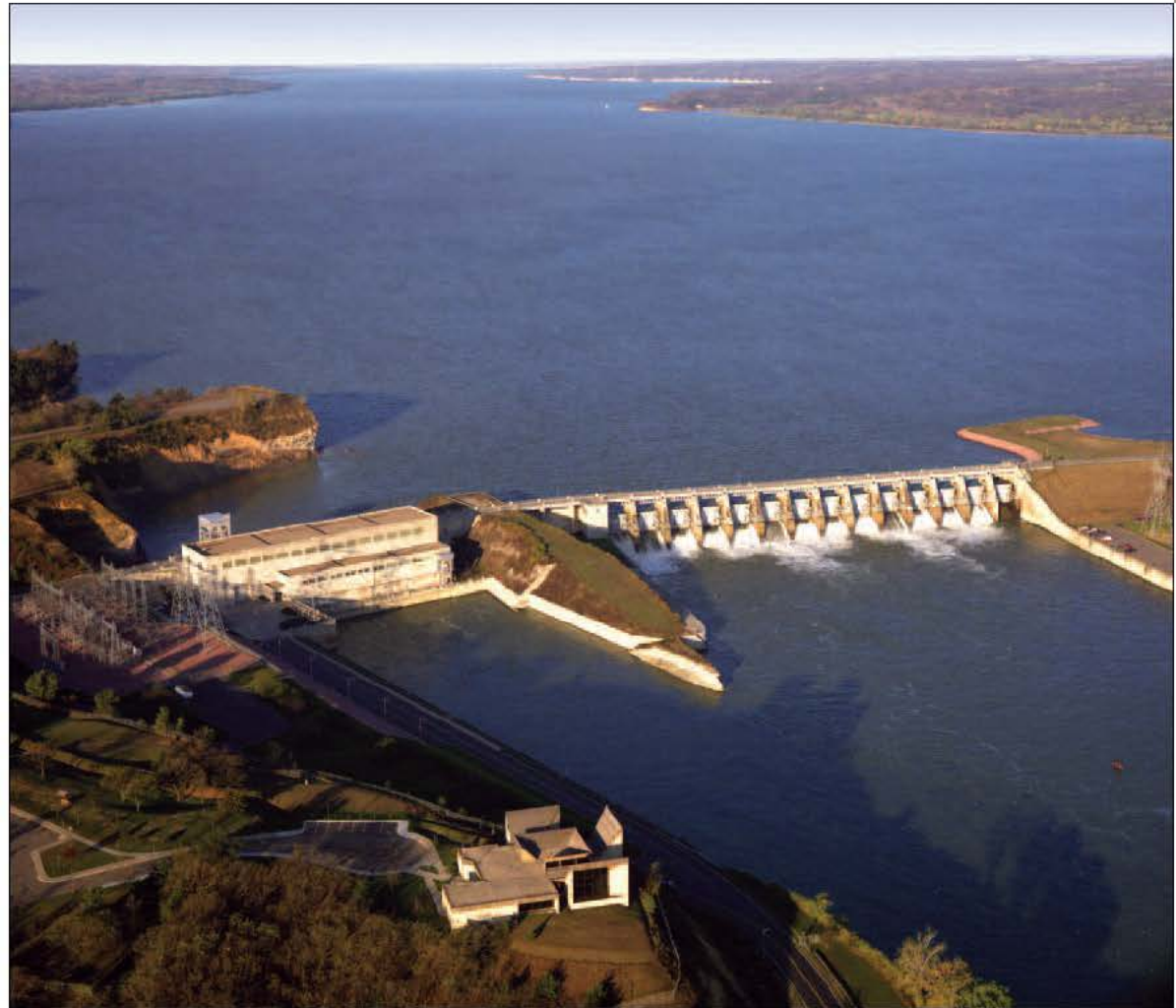
Gavins Point Dam lacks the flood control tunnels of the earlier main stem dams. Instead, it includes a spillway designed to handle water of any height.
