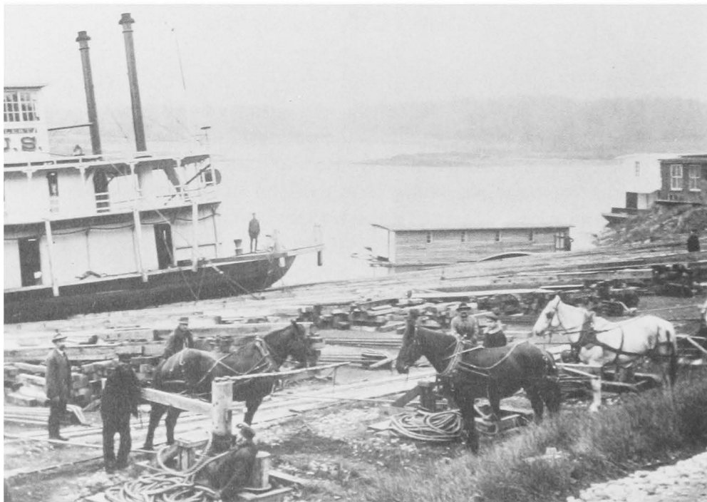
Horse-powered "Crabs" Were Used to Haul Boats Until 1948.
