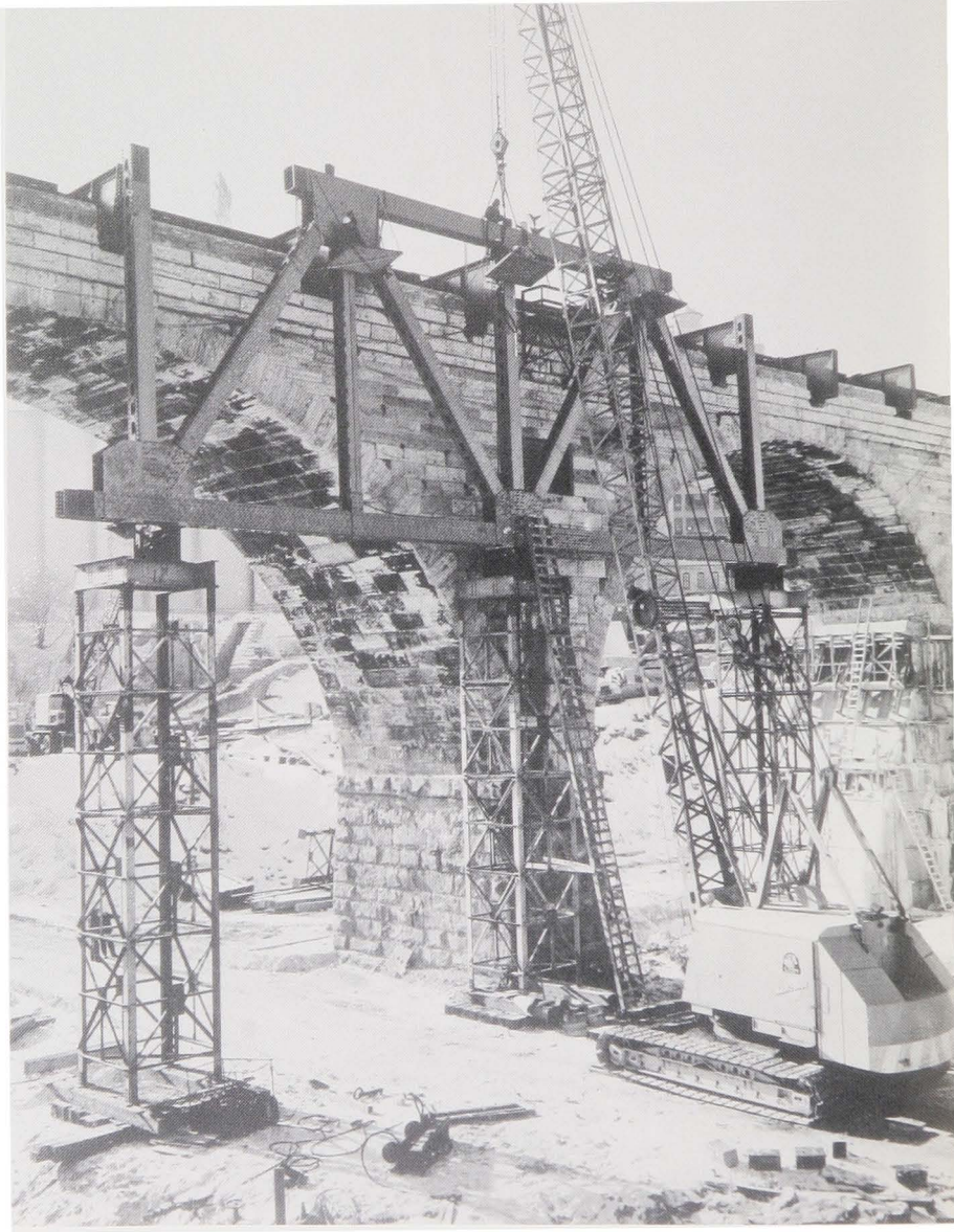
Building the trestle to replace two arches on the Great Northern Railway's Stone Arch Bridge. (St. Paul District)
