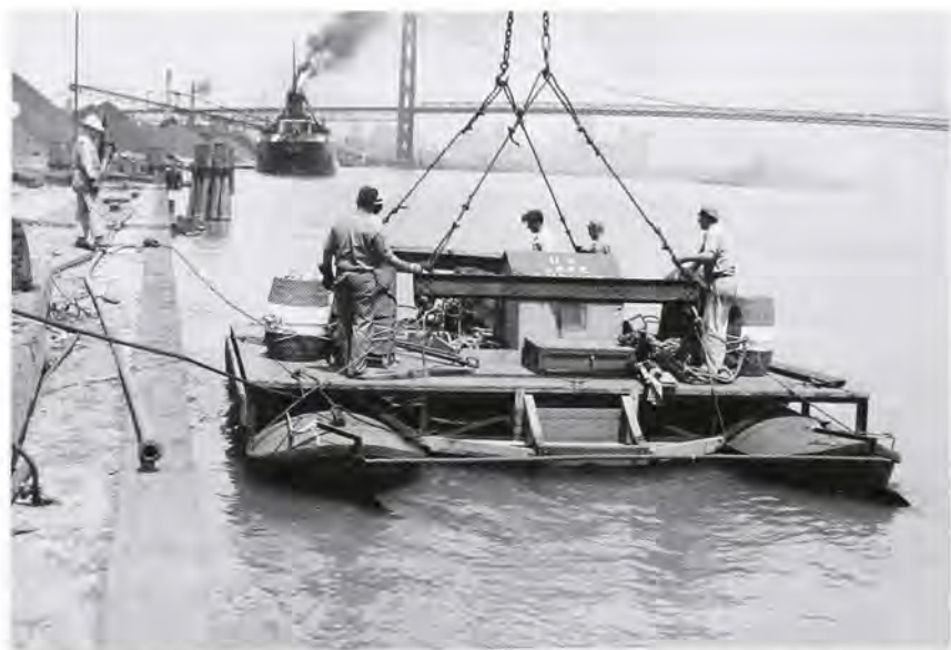
49. U.S. Lake Survey catamaran being lifted from the Detroit River for transport by truck to Ogdensburg, NY, for discharge measurements on the St. Lawrence River, 1945. Courtesy, U.S. Lake Survey Installation Historical Files, National Ocean Survey.
