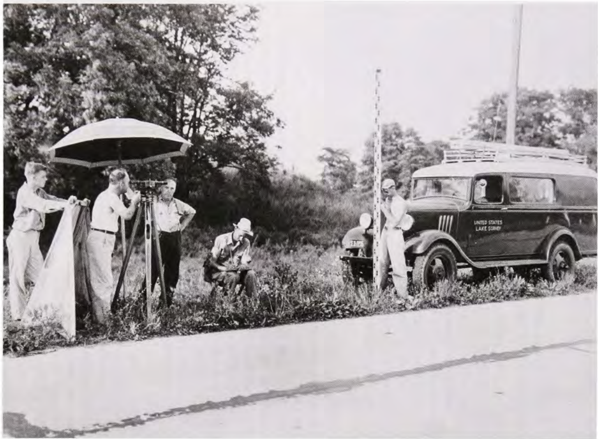
39. Members of a U.S. Lake Survey precise level party working in the vicinity of the Niagara River, 1937. Courtesy, U.S. Lake Survey Installation Historical Files, National Ocean Survey.
