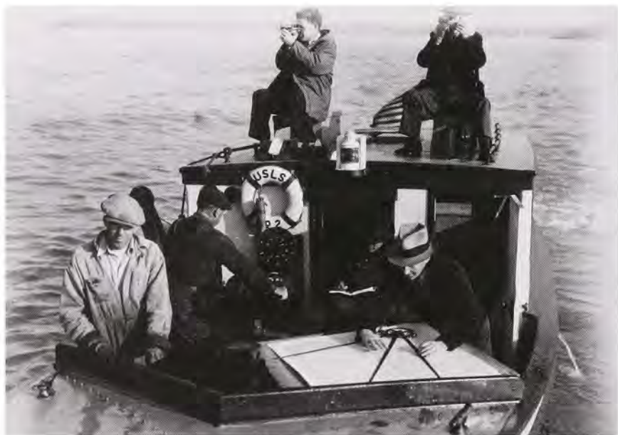
40. Taking soundings on board U.S. Lake Survey launch NO. 2 in the Detroit River, 1939. From left: wheelsman, J.S. Moore; sounding machine operator, E. Jewel; recorder (seated), E. Every; at the chart table, A.S. Purdy; sextant observers seated on the cabin roof, L.D. Kirshner (left) and G.E. Ropes. Courtesy, U.S. Lake Survey Installation Historical Files, National Ocean Survey.
