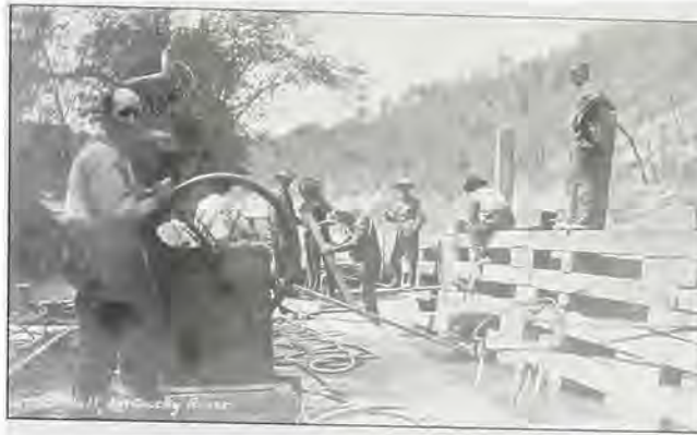
At Dam No. 11 in April 1906, a diver attaches lines to the last crib to be floated into position in the cofferdam around the dam site.
