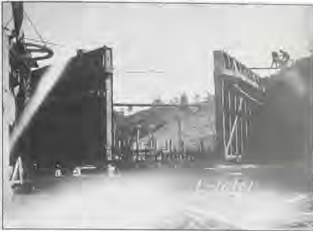
Test operation of the steel lockgates at Lock No. 10.
