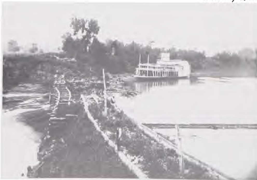
Deteriorated conditions at Dam No. 1 during the 1870's, with steamboat United States in the background.
