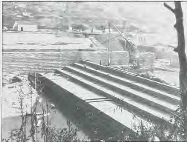
The completed timbercrib dam at No. 7.
