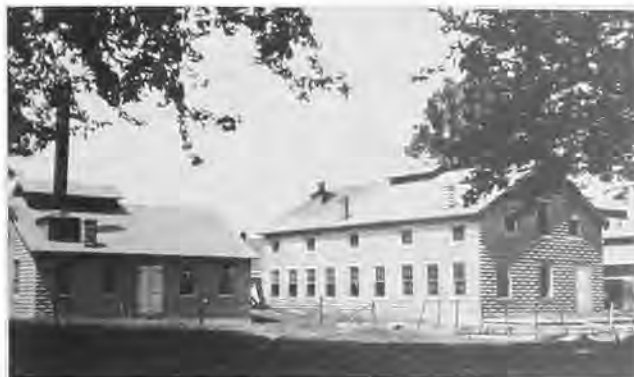
Powerhouse and machine shop at the Frankfort repair yard adjacent to Lock No. 4.
