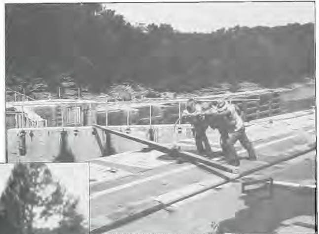
Lockmen turn the capstan to open the gates at Lock No. 8. In addition to turning the capstan in circles, they walked up and down the lockwalls to each capstan.
