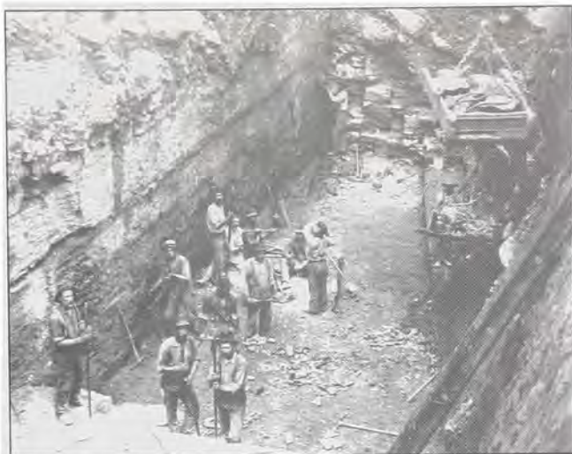
Excavation at Lock No. 7 in 1895 was still done with shovels and wheelbarrels.
