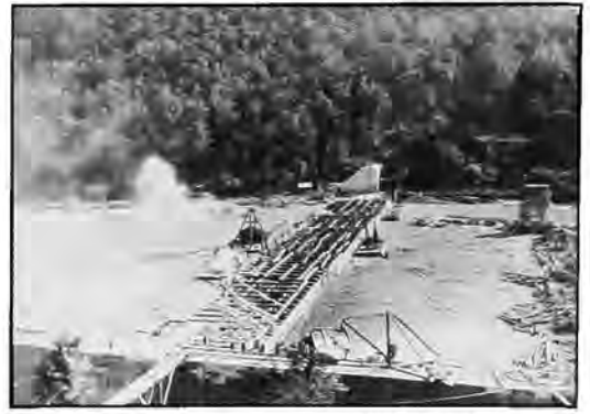
Timbercrib dam construction on the Kentucky River, 1885, at Lock No. 5.
