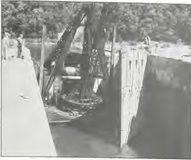
Corps repair crew and derrick replacing a lockgate at No. 5.
