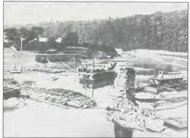
Rebuilding Dam No. 5 in 1885.
