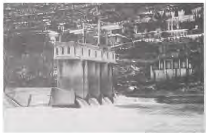
Kentucky Utilities powerhouse and transformer platform built at Lock and Dam No. 7 during the 1920s.
