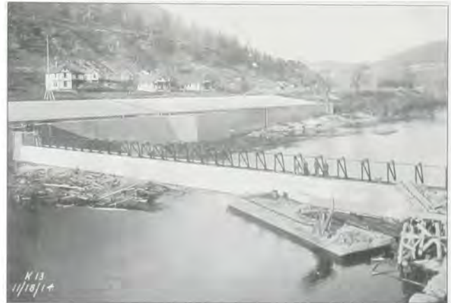
Metal trestles for the movable crest of Dam No. 13 are in place in Nov. 1914. A drift is at the left and a needle flat for maneuvering the trestles is at the right. Note the three lockhouses in the background.
