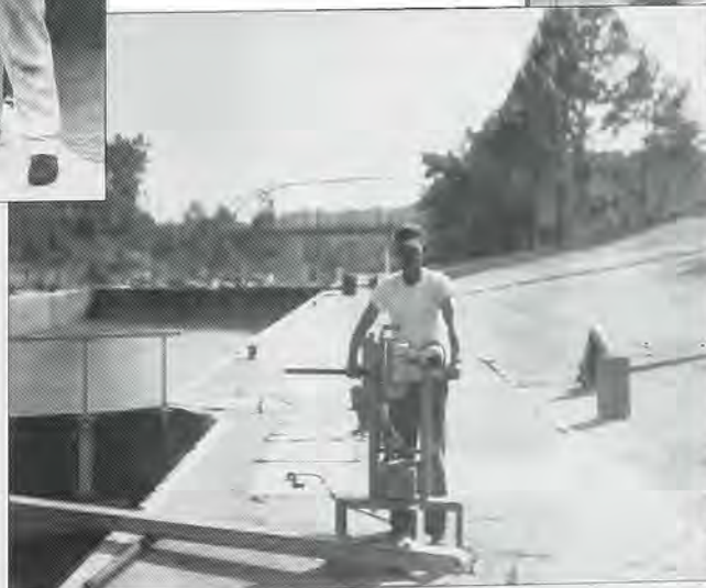
A 1958 view showing how electric drill motor coupled to a reduction gear made it possible for one lockman to operate lockgates.
