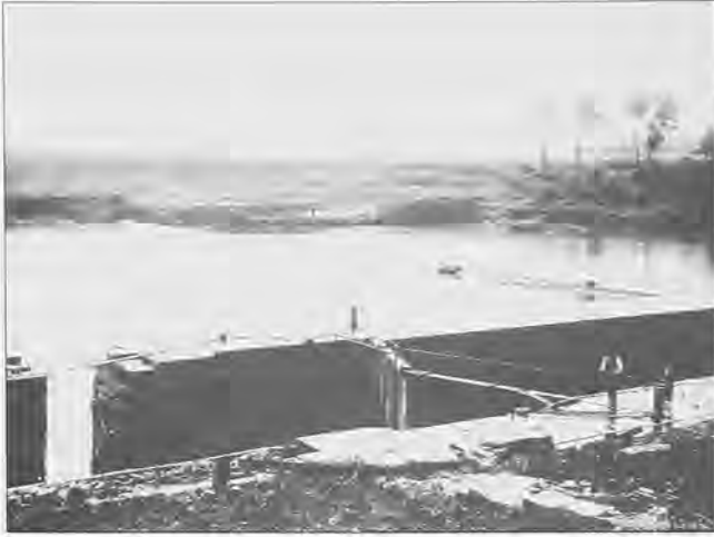
View of the manually operated lock mechanism at Lock No. 1
