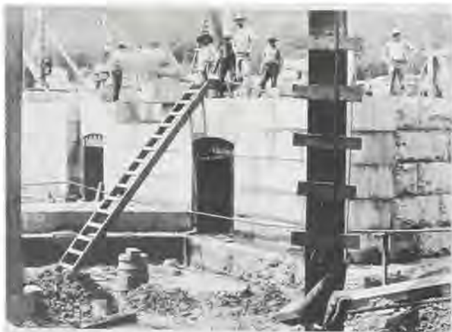
Workers building Lock No. 6, standing on the masonry emptying culverts.
