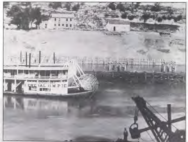
Snagboat General O. M. Poe and a dipper dredge working at Lock No. 7.
