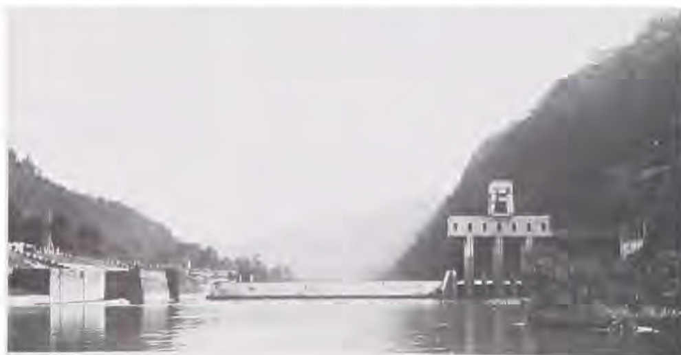
No water passed over Dam No. 7 during the 1930 drought. Structure on the right is the Kentucky Utilities powerhouse.
