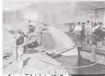
A ten-inch pump removes water from inside the bank cofferdam at Dam No. 14.
