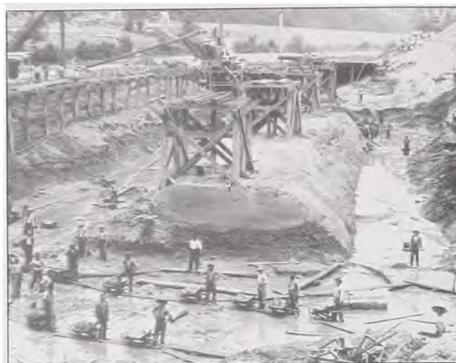
Workers excavating the abutment of Dam No. 7, loading stone on skips for hoisting and removal from the pit.
