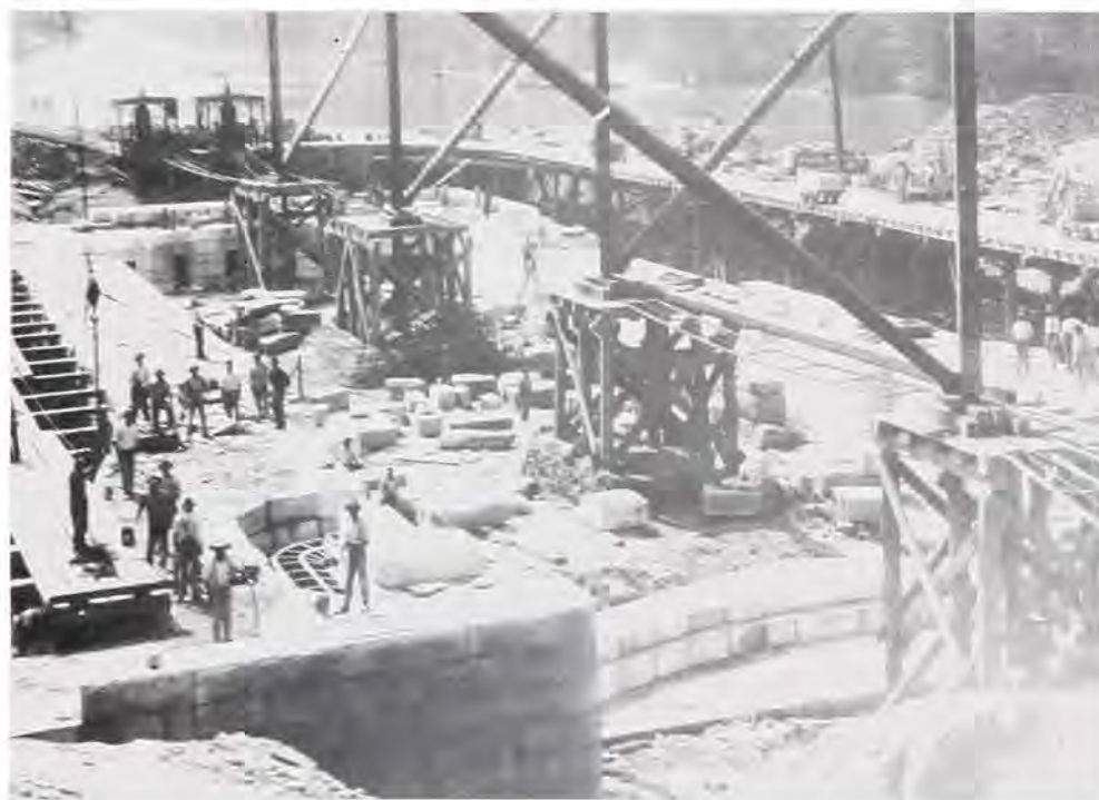
Finished stone was placed in the navigation lock walls
