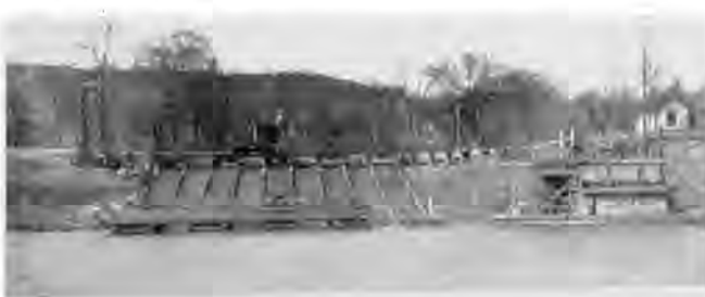
Launching a barge at marineway adjacent to the Frankfort repair yard at Lock No. 4 in 1923.
