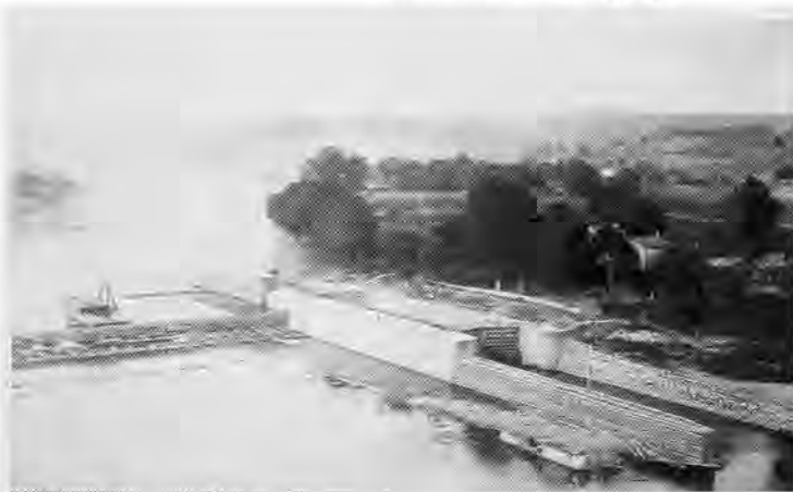
Plans for the Kentucky River project included navigation locks of stone masonry and dams built of timber cribs filled with stone.
