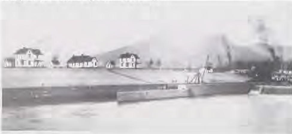
Lock and Dam No. 12 completed. Note the three lockhouses, provided because operating the movable dam crest required a crew of three men.
