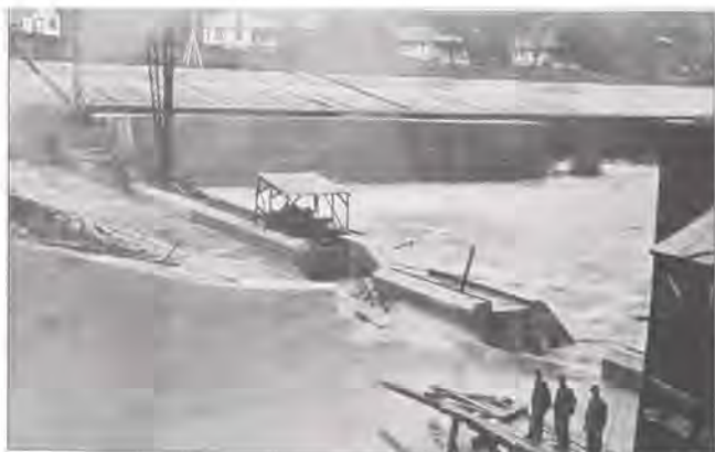
The concrete monoliths of Dam No. 13 were partly completed in Oct. 1914.
