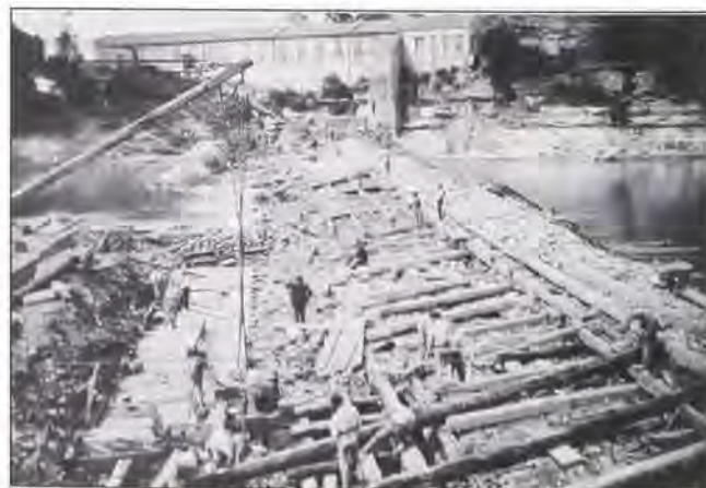
Rebuilding Dam No. 4 at Frankfort in 1885.
