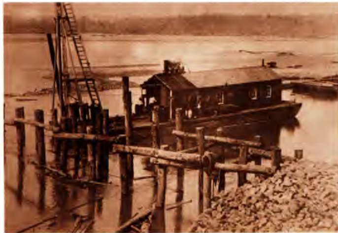
ILLUSTRATION 49. Little Rock District crew building pile and stone fill dikes to repair 1898 flood damage at Lower Greathouse Bend on the Arkansas River.
