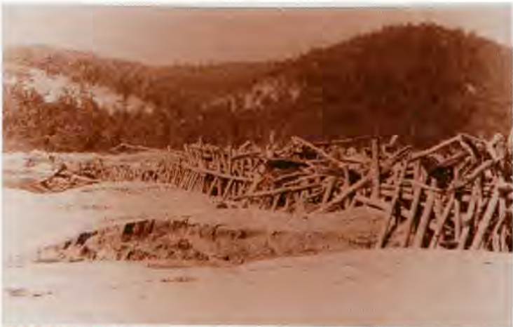
ILLUSTRATION 31. An effective permeable dike results in an accumulation of drift above the "dikebuilder" and a deposit of sand below.
