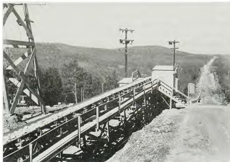
ILLUSTRATION 84. Conveyor belt at Bull Shoals Dam construction project.
