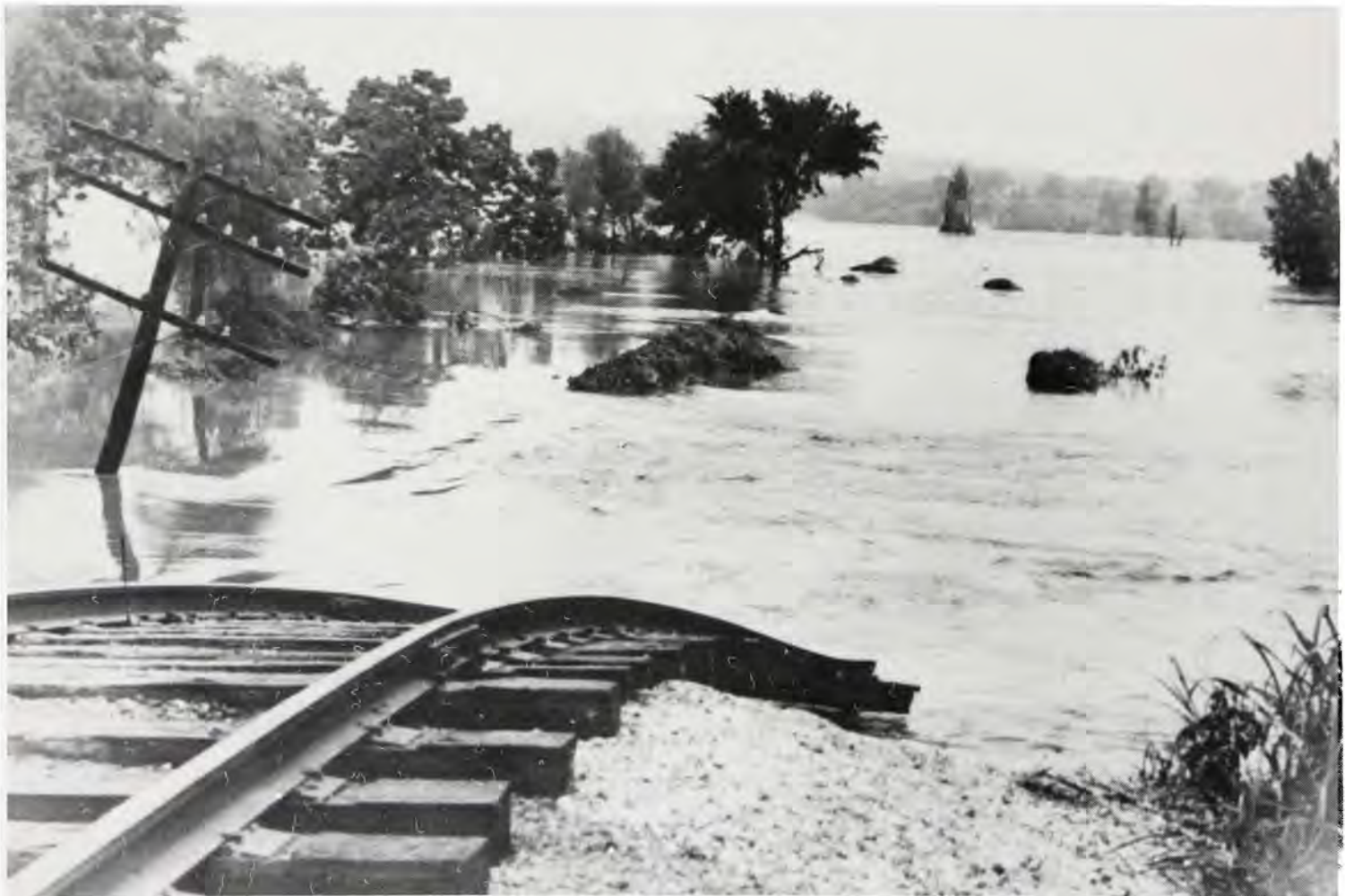
ILLUSTRATION 77. The Arkansas River washed out the Frisco Railroad in Van Buren, Arkansas in May 1943. (Courtesy of the U.S. Army Engineer District, Little Rock, AR)
