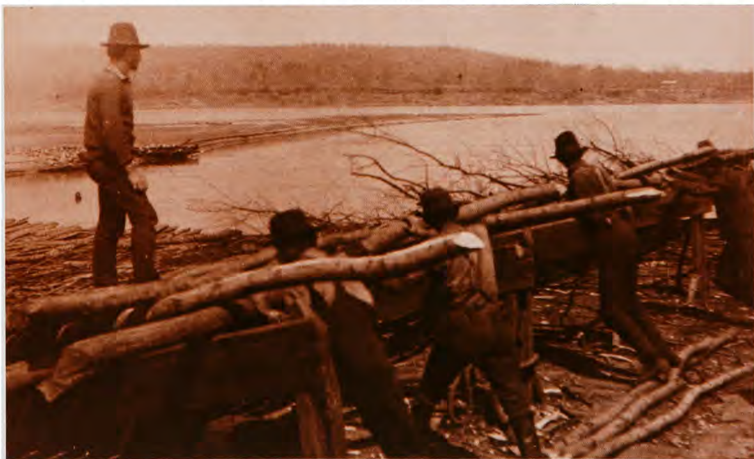
ILLUSTRATION 42. Workers building a willow mat. Willow mats were an essential part of brush and stone dams.
