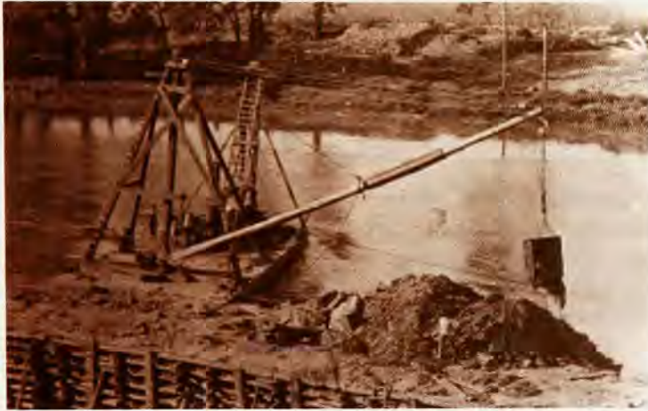
ILLUSTRATION 52. Removing spoil from Lock No. 1 pit.
