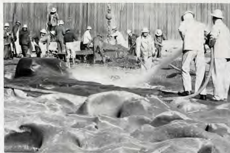
ILLUSTRATION 106. Workmen washing foundation rock at Dardanelle Lock and Dam complex, 2 December 1960.
