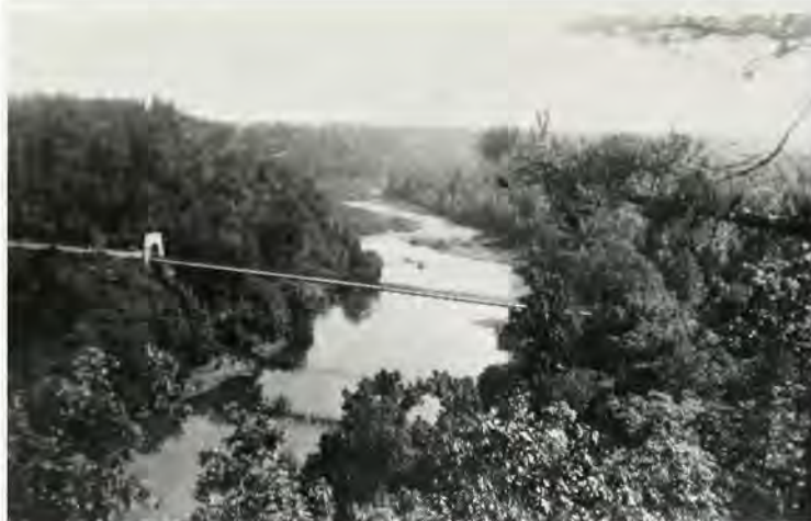
ILLUSTRATION 97. "Swinging" bridge over the Little Red River.
