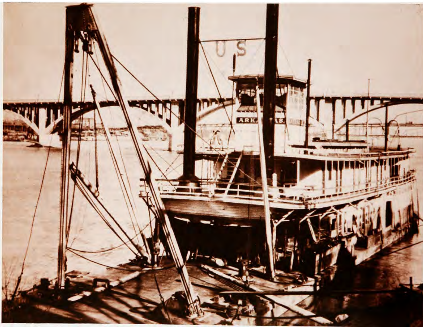
ILLUSTRATION 58. The steel hulled snag boat, the Arkansas , seen here along the Little Rock waterfront, was one of the District's prime maintenance tools in the 1920s.
