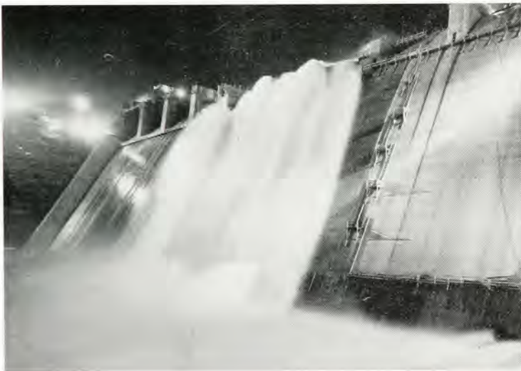
ILLUSTRATION 93. Flood water overtopping Table Rock Dam while still under construction in 1957.
