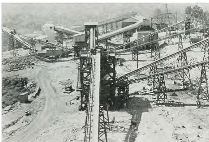
ILLUSTRATION 85. Aggregate plant at Bull Shoals Dam.
