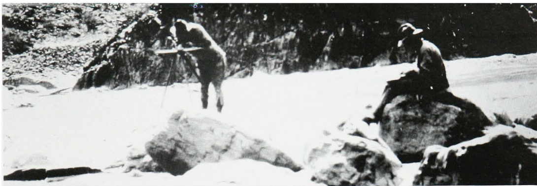
Section 308 survey crew at work in Arkansas
