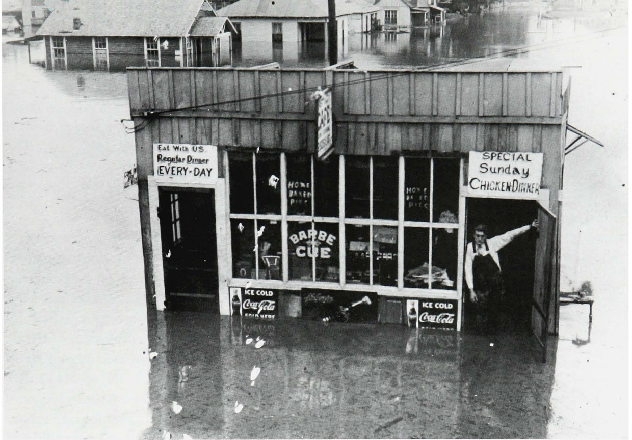
Flooded restaurant at North Little Rock, April 1927
