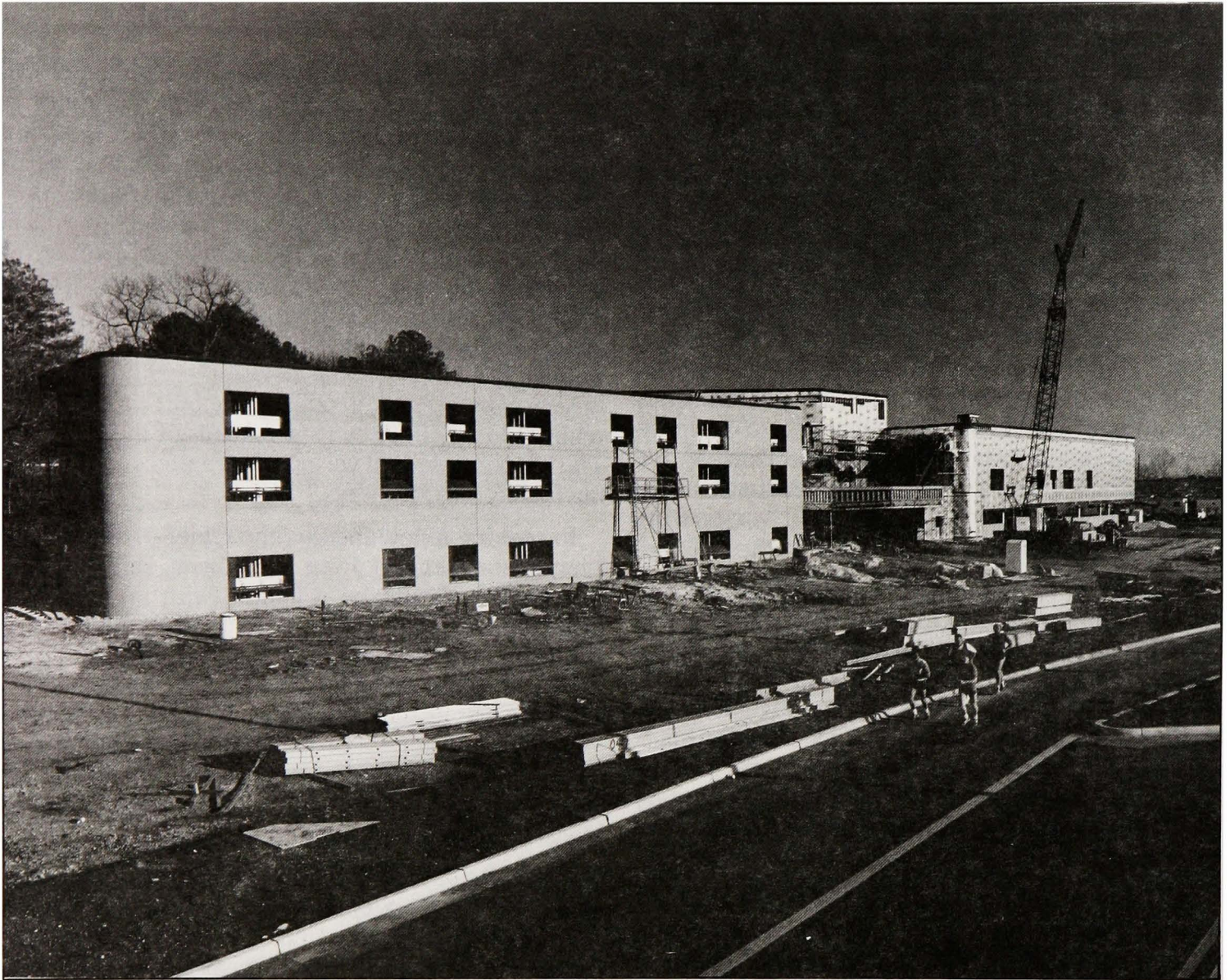
Fig. 10. New Training Center under construction, March 1987.
