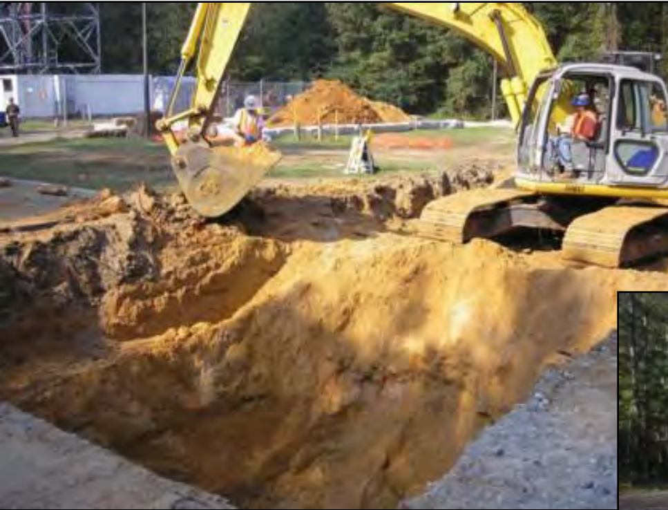
TCE Source Removal Adjacent to Radar Tower
