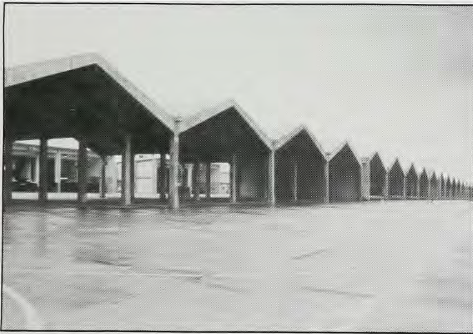
The concrete weather shelters replaced corroding metal shelters.
