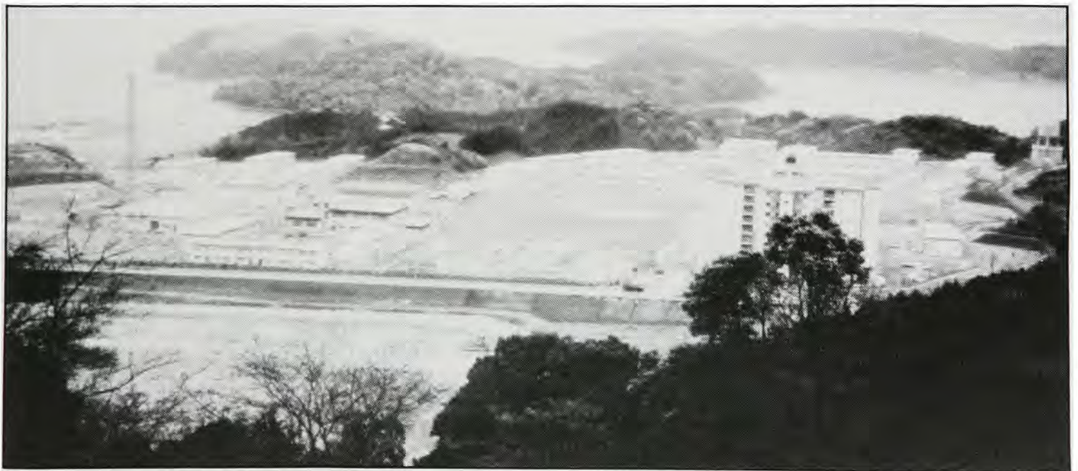
An overview of the new facilities at the Hario Housing Area.
