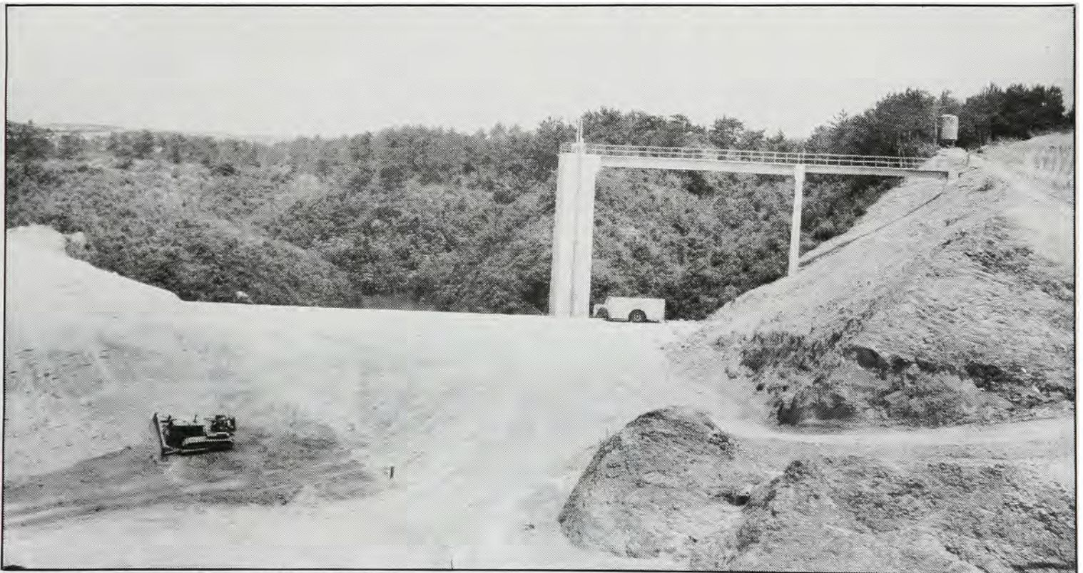
Construction of Tengan Dam and Reservoir.
