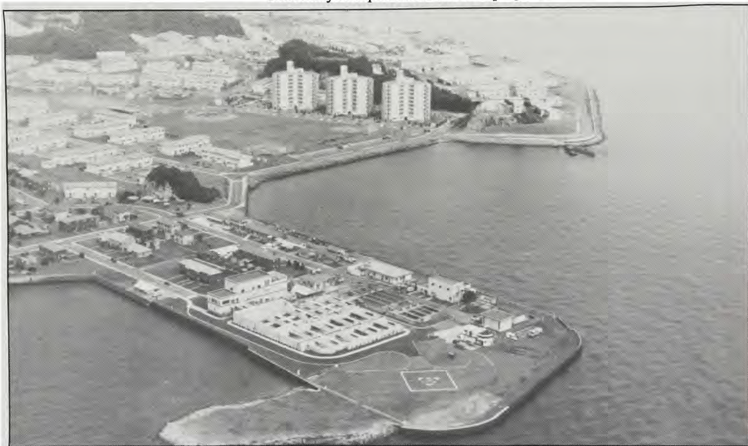
An aerial view of the sewage treatment plant as it appeared while under construction in 1983.
