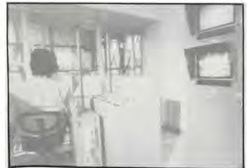
Interior of the trash incinerator at Yokosuka.
