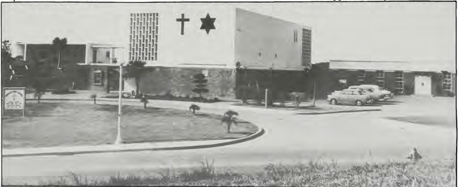
Sukiran Army Chapel. This typhoon resistant chapel provided seating for 300 people. This same design was used for a chapel at Kadena Air Base.
