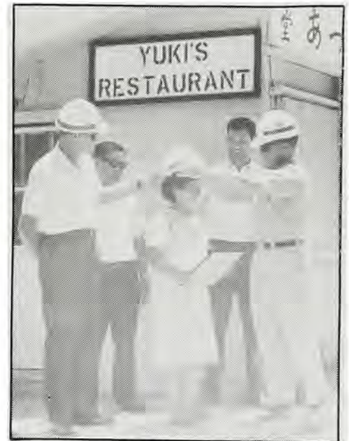
On July 16, 1969 Miss Yuki Nakamura was presented with a certificate of appreciation and a personalized hard hat by Lieutenant Colonel William S. Cutler, acting district engineer. For over two years, Miss Nakamura cooked and served OED construction representatives and acted as an unofficial vehicle dispatcher and welcoming committee to VIP's at the Fukuji dam site in Kawata Village. The certification included these words: "... from this day forward, Miss Yuki Nakamura will be tendered the honorary title of Inspector - Okinawa Engineer District, Corps of Engineers."
