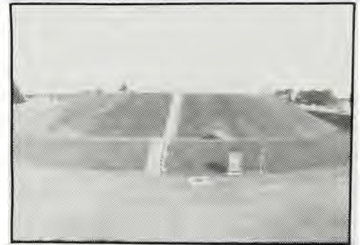
The hydrant fueling system included two temporary underground fuel storage tanks, pump house, filter separator facility and 15 hydrant fueling pits.
