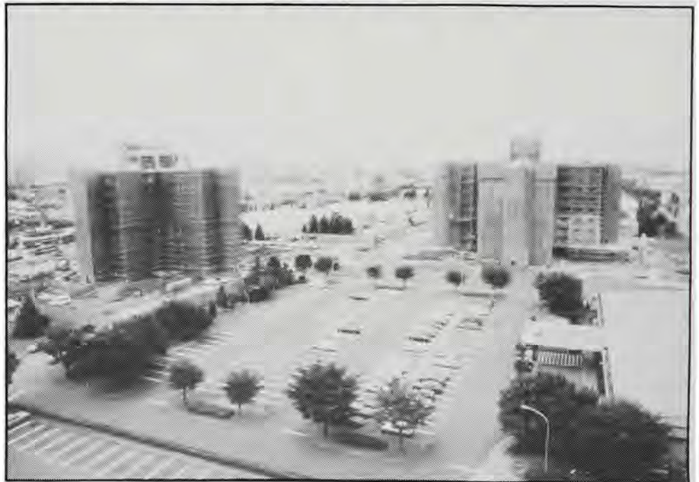
These new highrises provided the first new housing on Yokota in several years.
