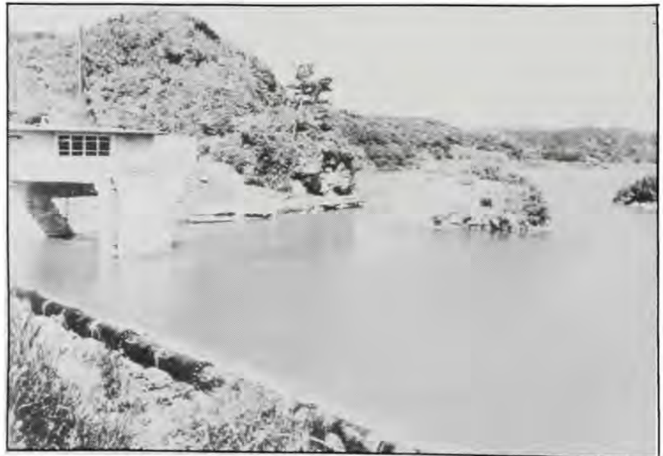
The Zukeyama dam and reservoir was an OED project for the Ryukyu Domestic Water Corporation.
