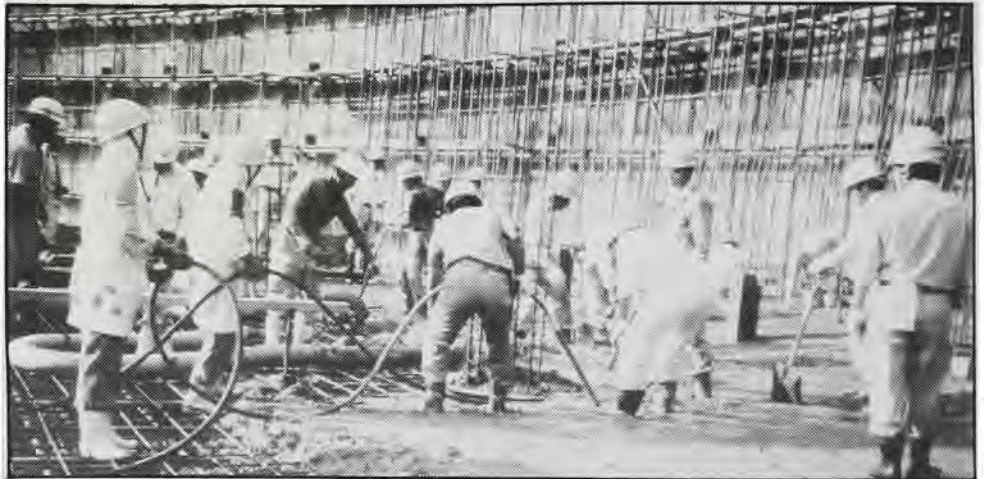
The workers in this photo show the scale of the tanks.
