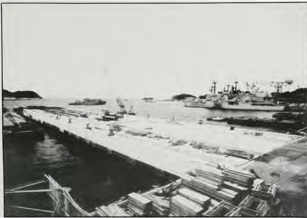
Harbor Master Pier under construction in September 1990.
