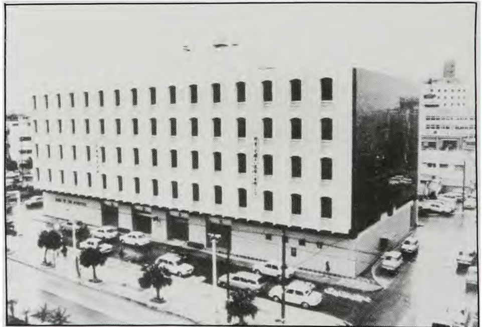
The Okinawa District constructed the Bank of the Ryukyus for USCAR.
