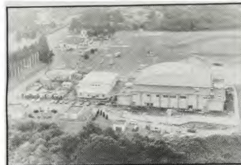
The new hangar (in the right of the above photo) dwarfs the hangar it replaced (left of the photo). The fuel storage tank, fire station, operations building and control tower surround the airfield. The new hangar could accommodate all the battalion's Blackhawks (left) greatly reducing the time required for maintenance.
