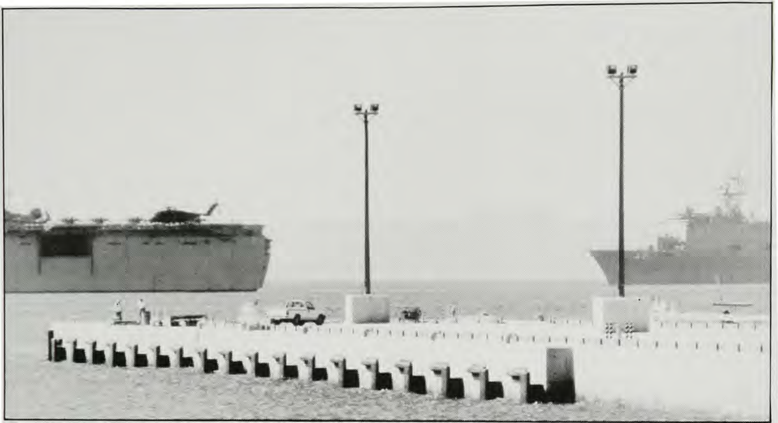
Pier Bravo after construction completion.
