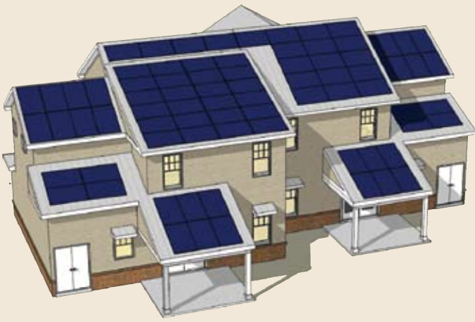
Applying ZEH design concepts that incorporate synergies between architecture and mechanical/electrical systems, the roof of this house was redesigned to provide additional space for photovoltaics.
