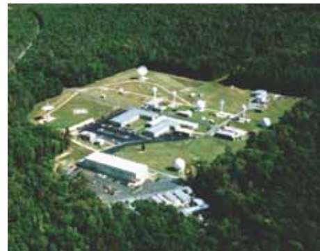
Blossom Point Satellite Tracking and Command Facility.
