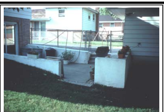
This floodwall was installed after the owner attended a local workshop on flood proofing. The community also helped pay for the project with a rebate. It has kept floodwaters out of the house three times since it was built in 1991 (South Holland, Illinois).
