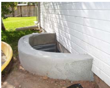
Some of Fort Collins' flood proofing projects to keep surface waters from entering basements
