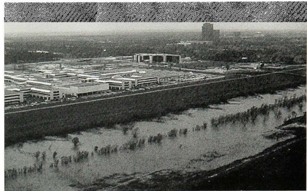
Right: Water collects behind Addicks Dam after heavy rains.
