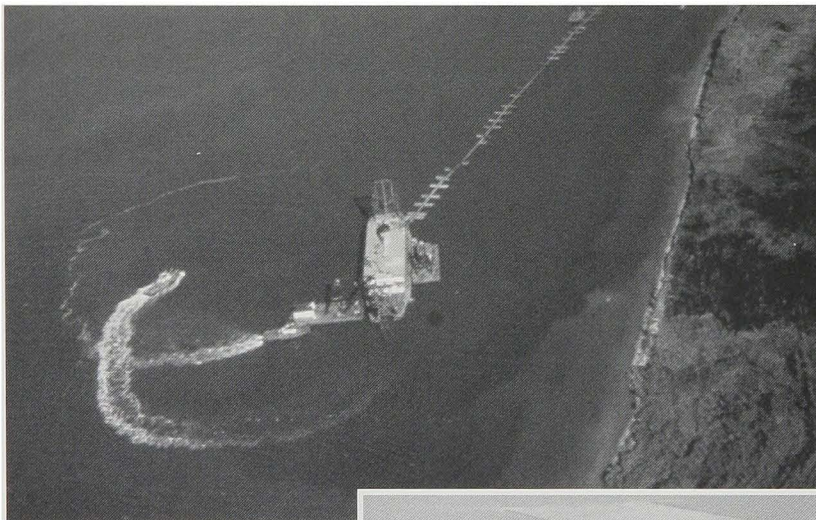
Above: Dredging activity on the GIWW keeps the waterway to its 12-foot depth.
