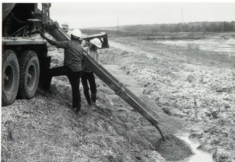
Reinforcing drilling “mud” flows into Addicks Dam slurry trench.
