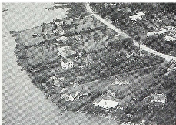
Subsidence allowed Alicia’s storm waters to wash in and flood these homes in the Baytown area.
