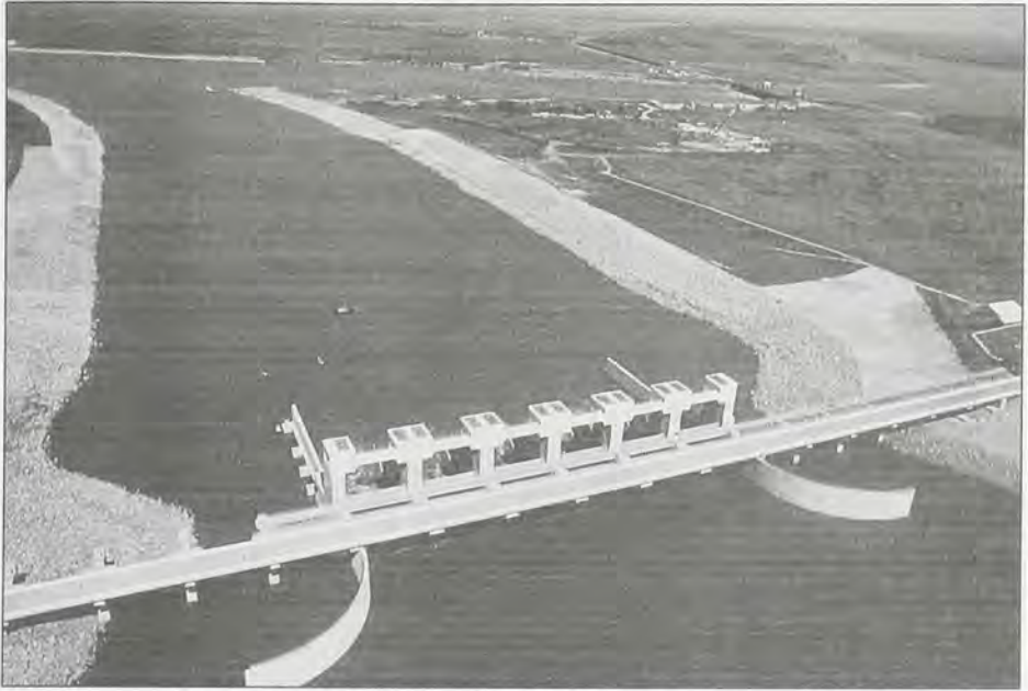
Old River Control. The auxiliary structure is in the foreground. The low sill and overbank structures are in the upper right (1987).
