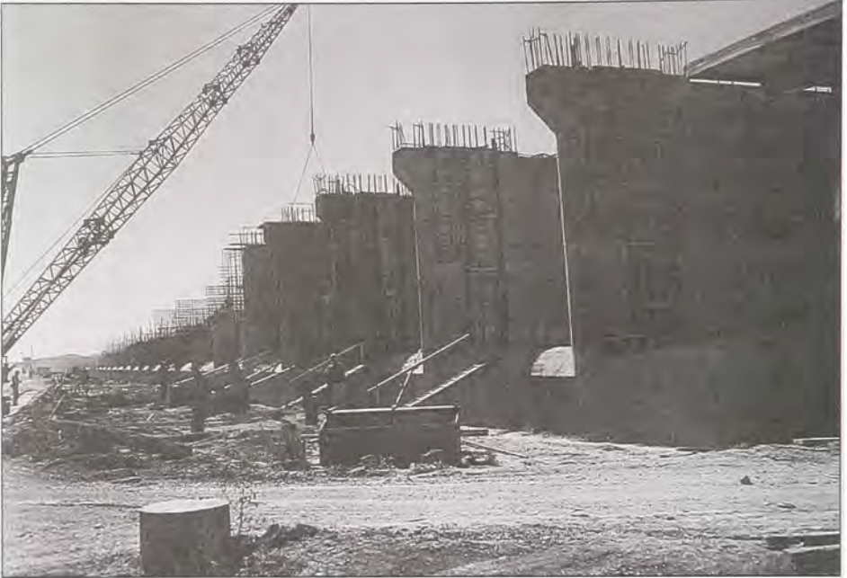
Morganza Floodway intake structure under construction, 1951.
