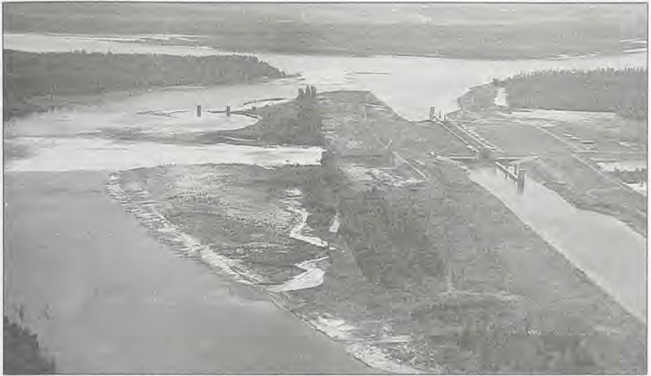
New navigation lock and channel at Old River, 1963. The large dam to the left permanently blocks the lower Old River.
