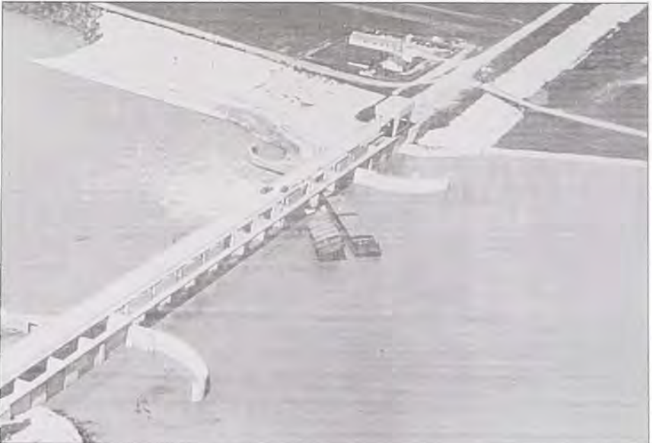
Barge collision at the low sill structure, 1965.
