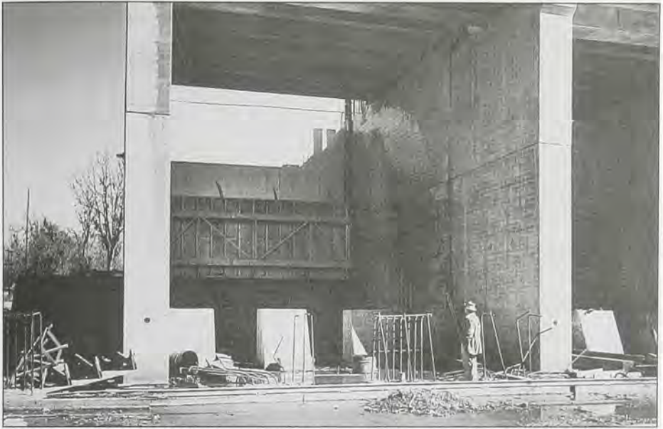
Morganza Floodway intake structure under construction, 1952.
