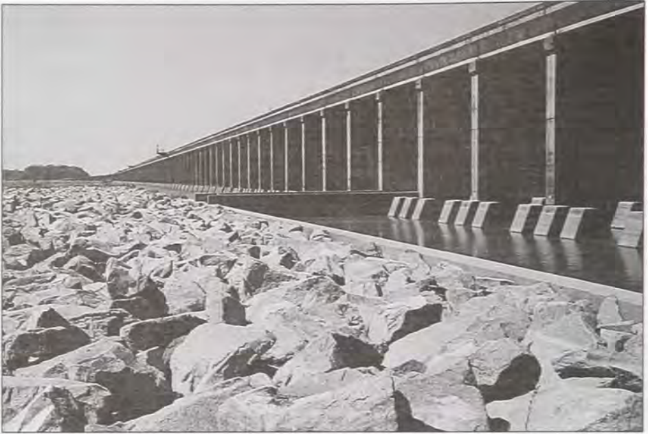
Completed Morganza Floodway intake structure (outflow side).
