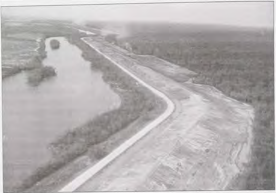
West Atchafalaya Basin Protection Levee, November 1987.
