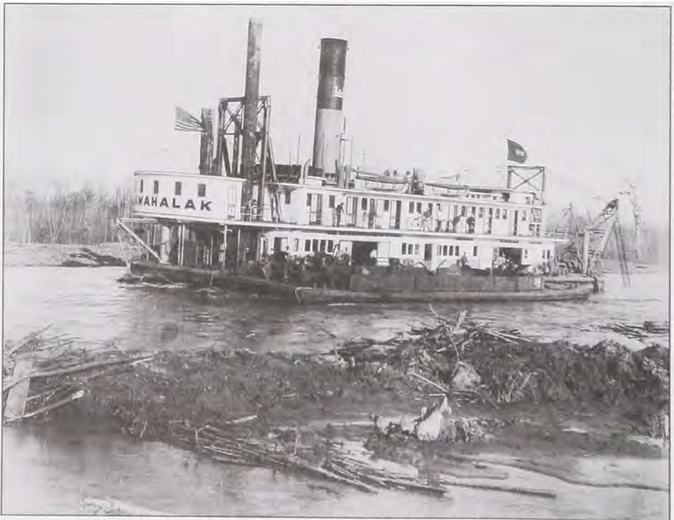
The Corps of Engineers' pipeline dredge Wahalak working in the Butte La Rose cutoff, Atchafalaya Basin, 1933.
