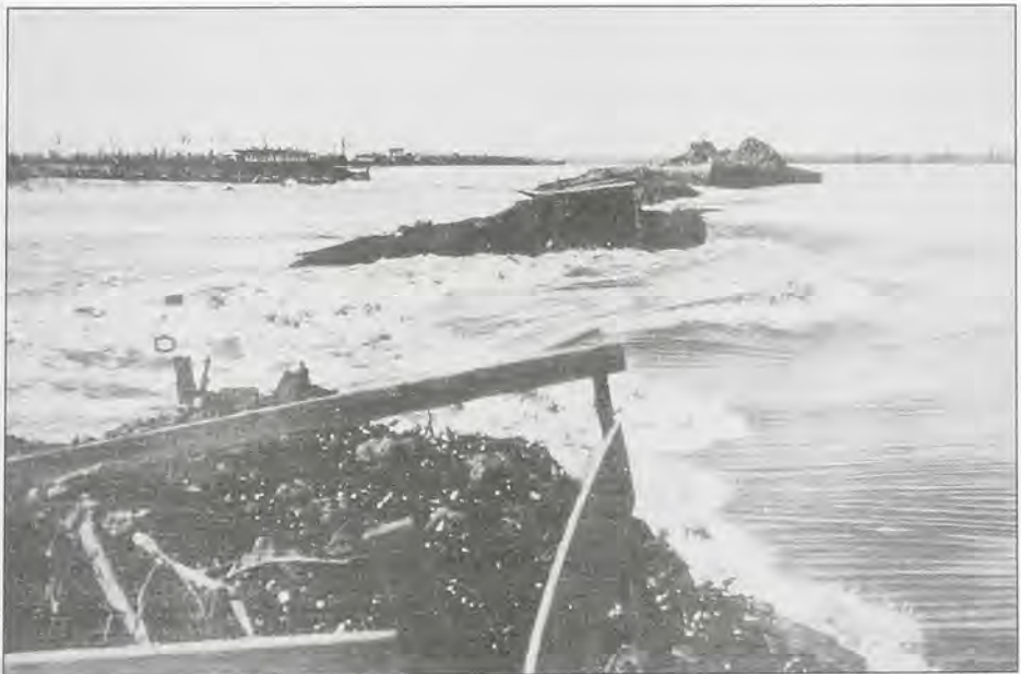
Three crevasses at Cypremort, Louisiana, during high water in the Atchafalaya Basin, 1932.
