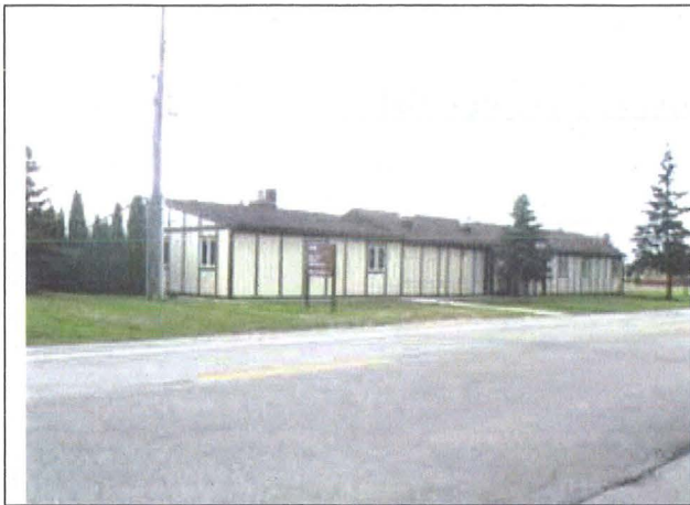
Project 7. Visitor's Quarters Phase IV
