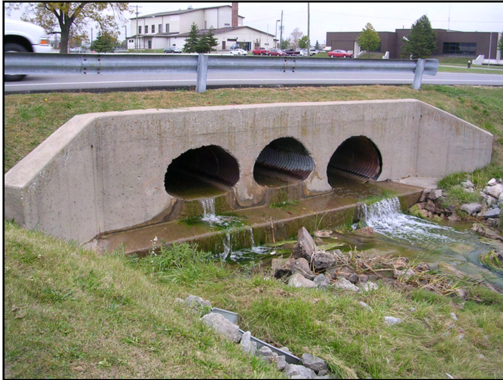
Figure 2-7. Existing Wagner Drive Culvert
