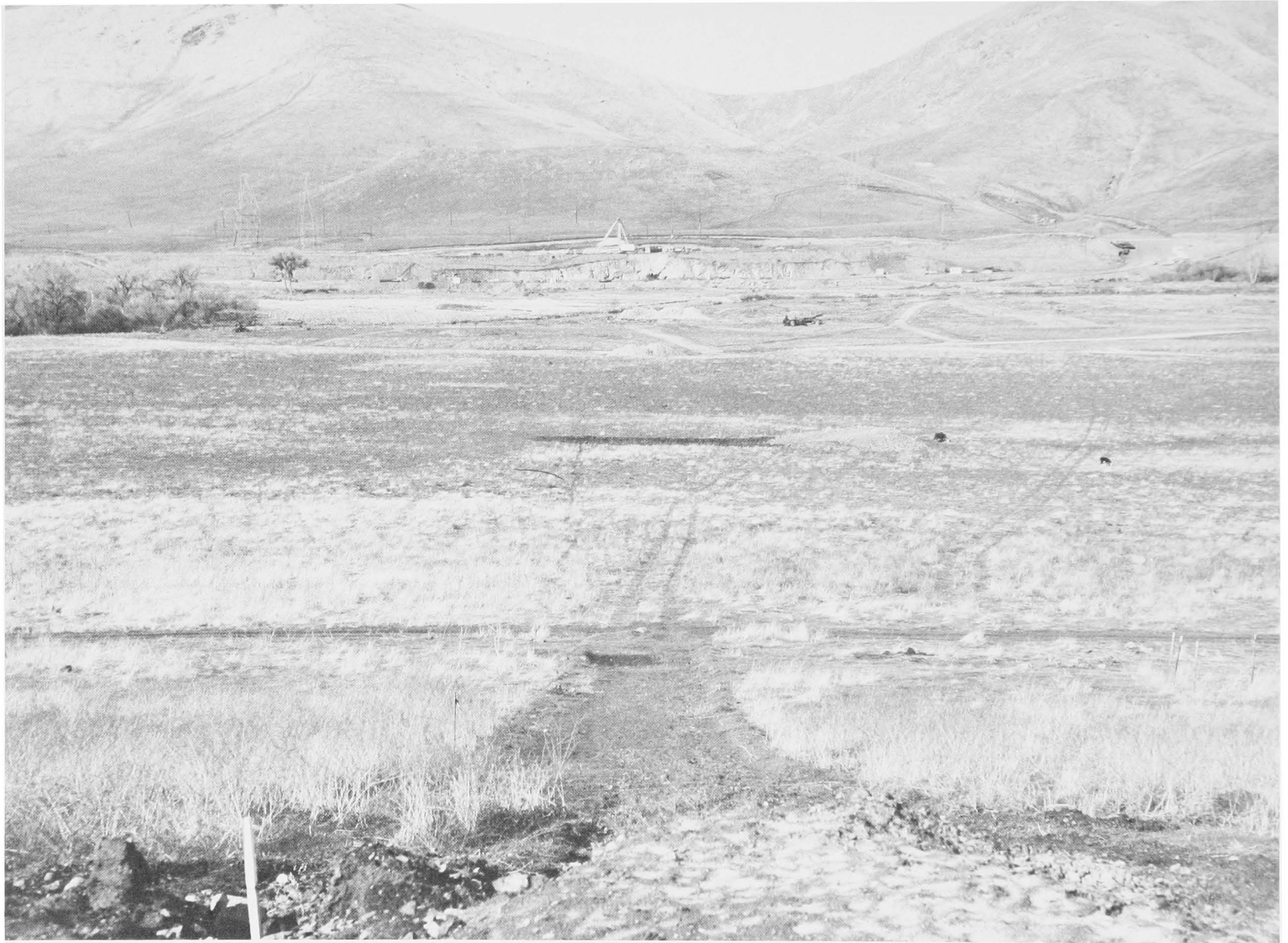
SITE OF SUCCESS DAM PRIOR TO CONSTRUCTION (TAKEN IN FEBRUARY 1959). THIS DAM IS ON THE TULE RIVER, IN TULARE COUNTY.
