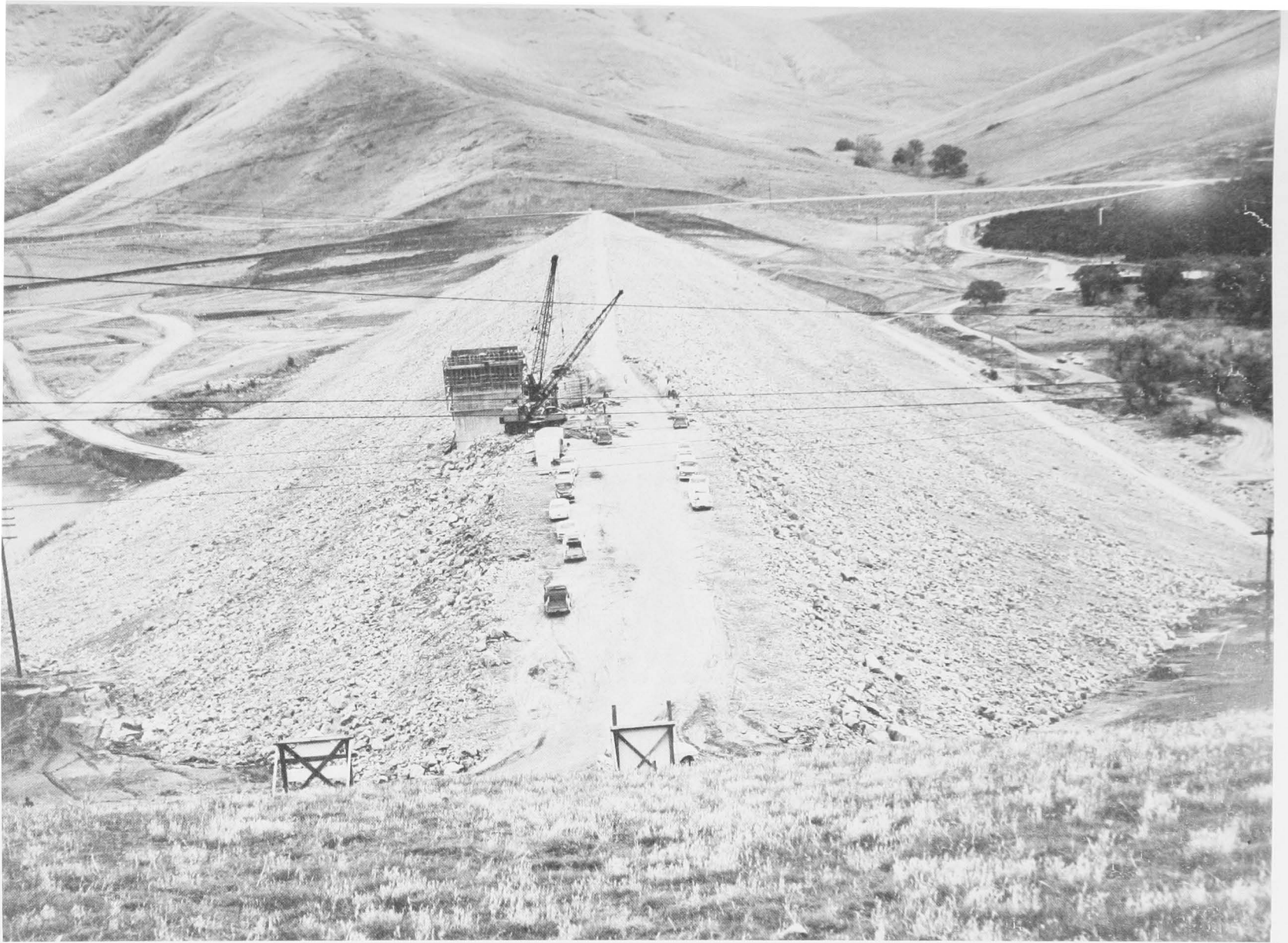
SUCCESS DAM — NEARLY COMPLETE: NOTE THE CONTROL TOWER ON THE LEFT.
