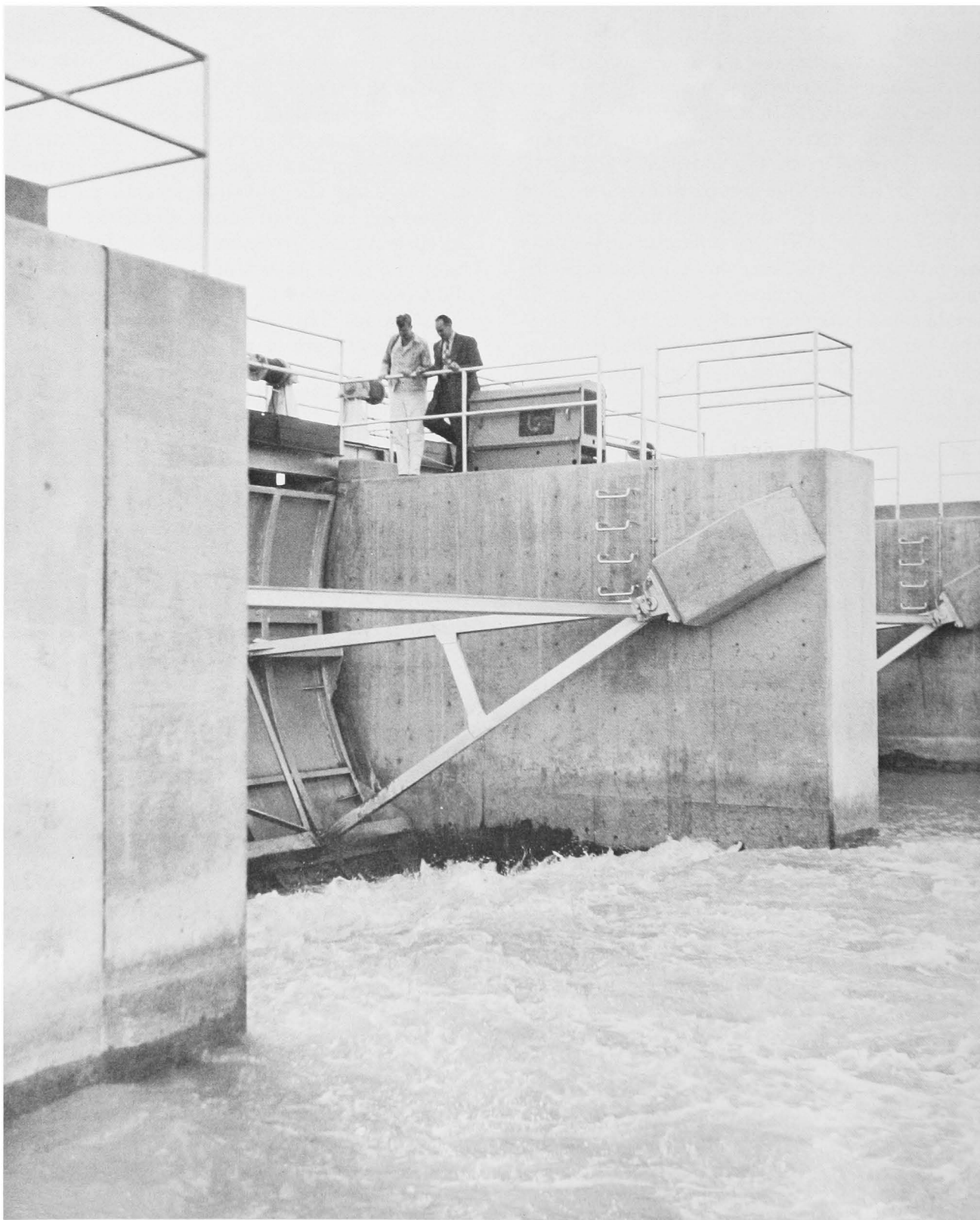
GUNNISON-FAYETTE DIVERSION STRUCTURE, SEVIER RIVER.
