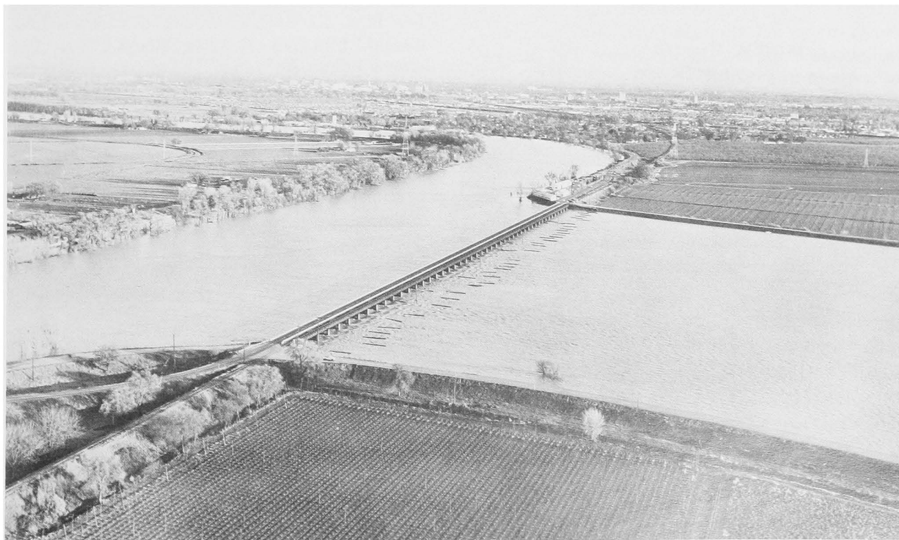
SACRAMENTO WEIR IN OPERATION. THE CITY OF SACRAMENTO IS IN THE BACKGROUND.
