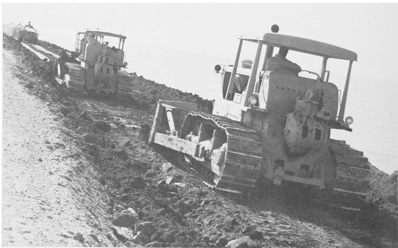
A CONVOY OF DOZERS RAISE A LEVEE IN THE FLOODED TULARE LAKE BASIN TO PROTECT CROPS FROM BEING DESTROYED. THE BASIN RECEIVED BOTH RAINFLOOD AND SNOWMELT WATER FROM ONE OF THE WETTEST SEASONS IN HISTORY IN THE HIGH SIERRA NEVADA. APRIL 1969.
