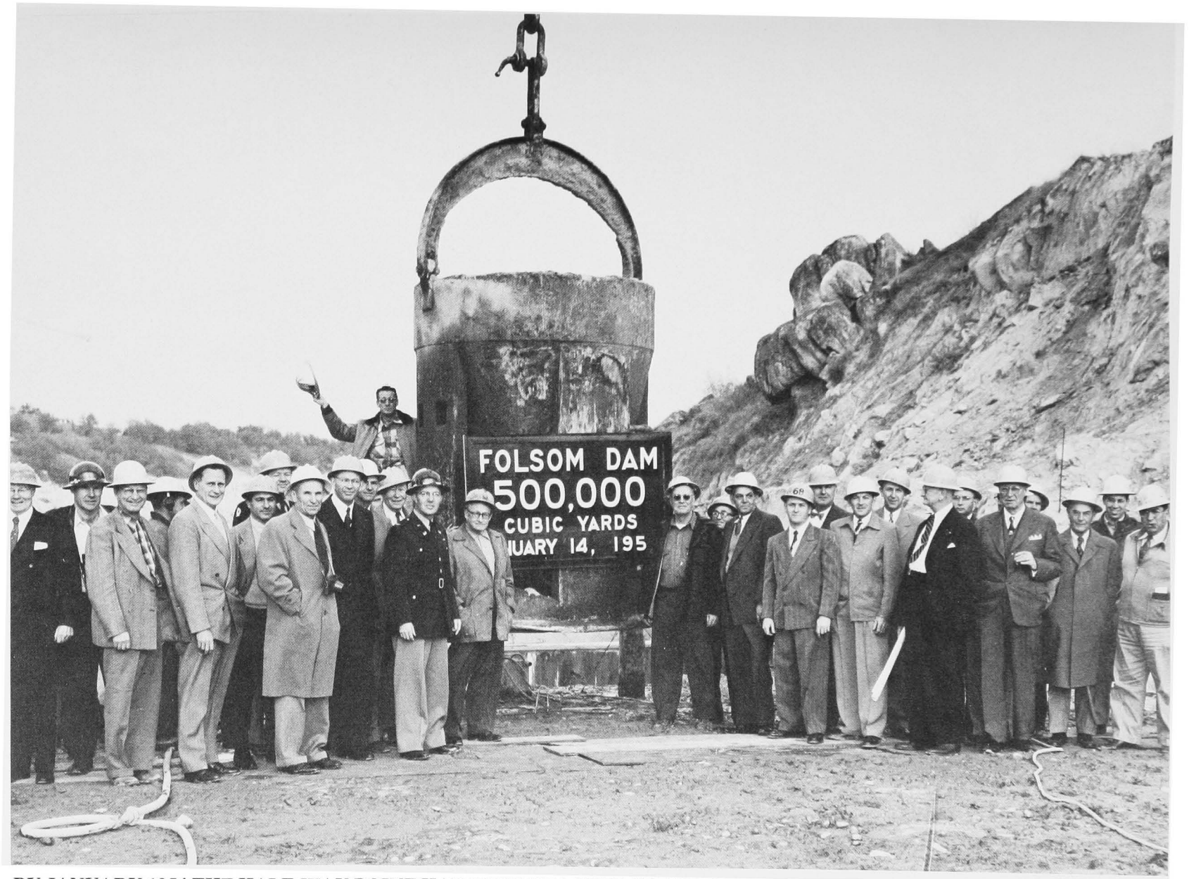
BY JANUARY 1954 THE HALF-WAY POINT HAD BEEN REACHED IN THE PLACING OF CONCRETE. DISTRICT PERSONNEL POSE FOR THE OCCASION.
