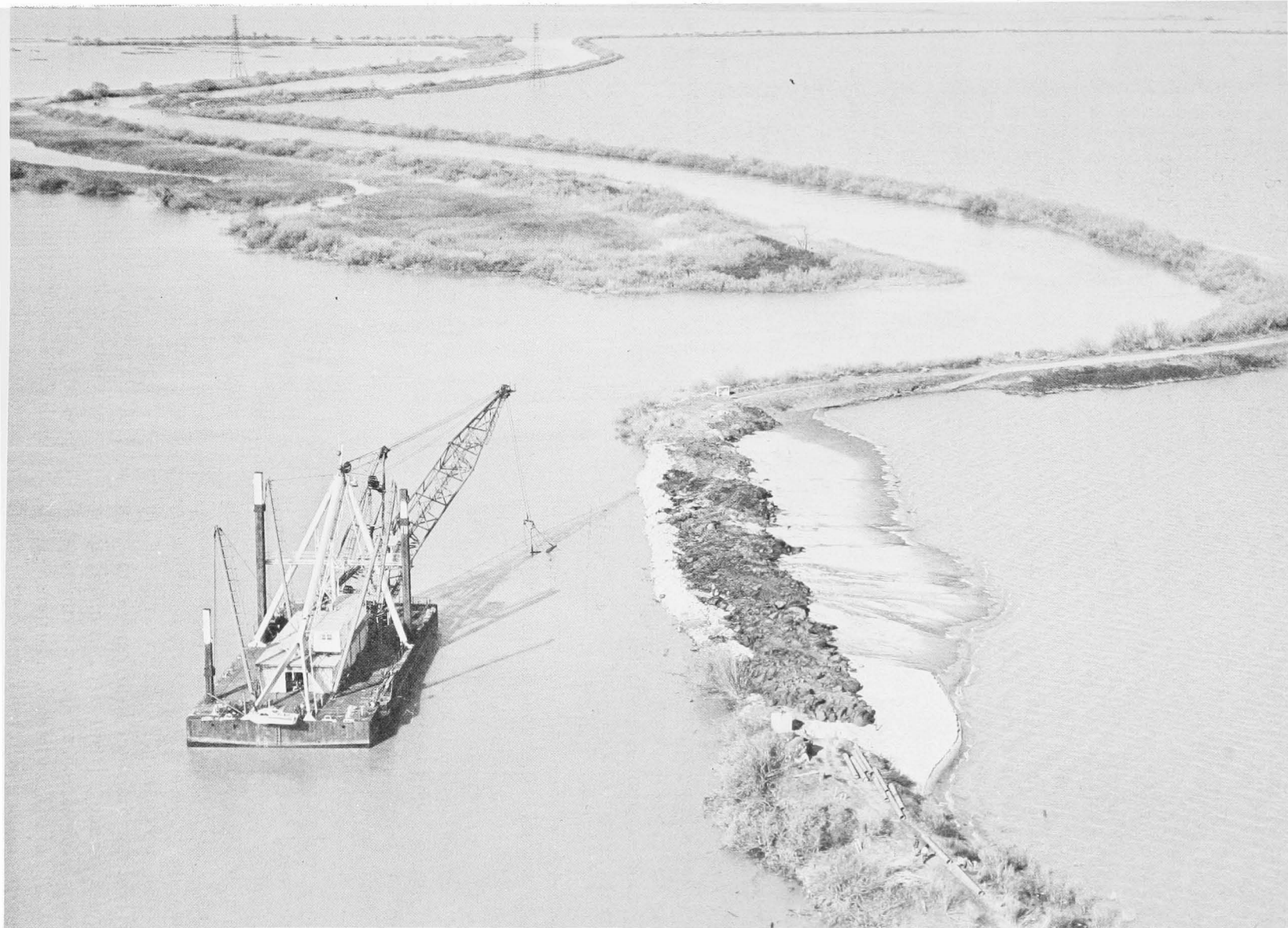
EMERGENCY LEVEE REPAIR WORK — SHERMAN ISLAND IN THE SACRAMENTO-SAN JOAQUIN DELTA — 13 FEBRUARY 1969.
