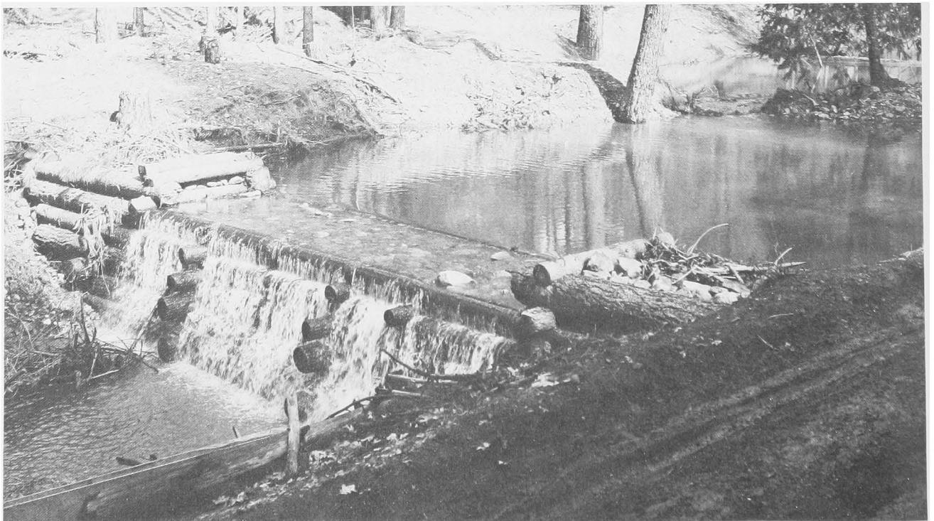
SMALL, PRIVATELY CONSTRUCTED, DEBRIS DAMS SUCH AS THESE PROVED INEFFECTUAL IN THE FIGHT TO HOLD BACK THE FLOOD OF DEBRIS THAT WAS BEING WASHED INTO THE RIVERS OF THE WESTERN SIERRA.
