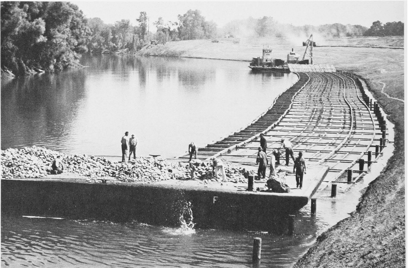
WOVEN LUMBER MATTRESSES, MANUFACTURED AT THE SITE AND HELD IN PLACE BY COBBLES, WERE USED EXTENSIVELY FOR BANK PROTECTION PRIOR TO THE WAR. THIS TYPE OF ACTIVITY WAS GREATLY CURTAILED DURING WORLD WAR II.
