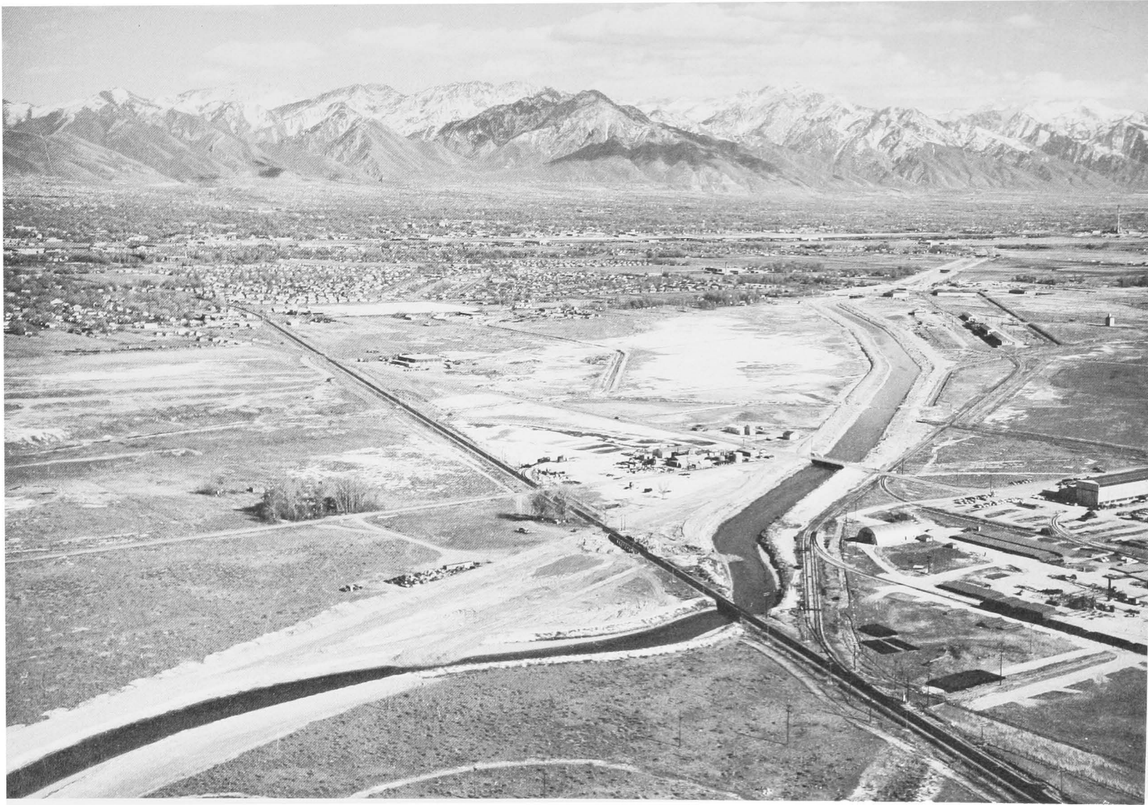
LEVEE CONSTRUCTION AND CHANNEL IMPROVEMENT, JORDAN RIVER, SALT LAKE CITY, UTAH. SURPLUS CANAL REALIGNMENT AND NEW RAILROAD BRIDGE ON U.P. RAILROAD LINE, LOOKING SOUTHEAST. APRIL 1960
