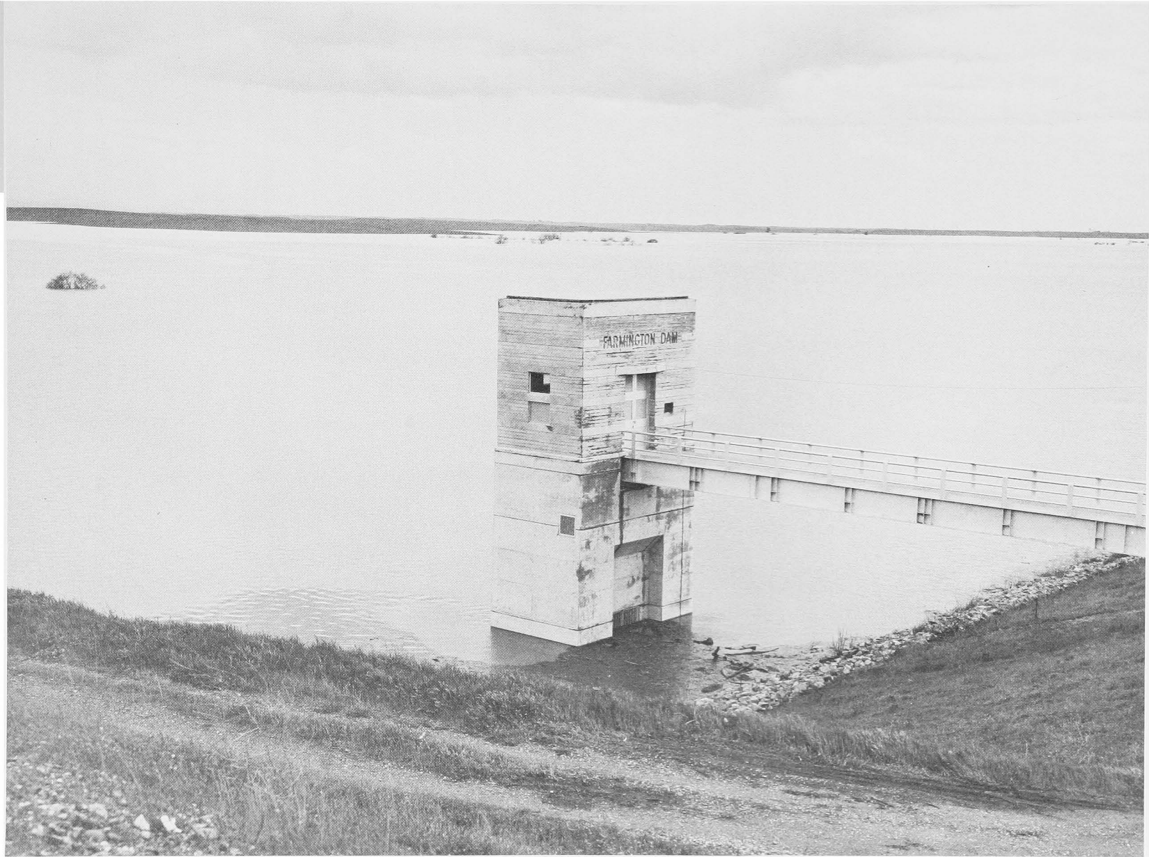
FARMINGTON DAM AND RESERVOIR. (Army Corps of Engineers Photo)
