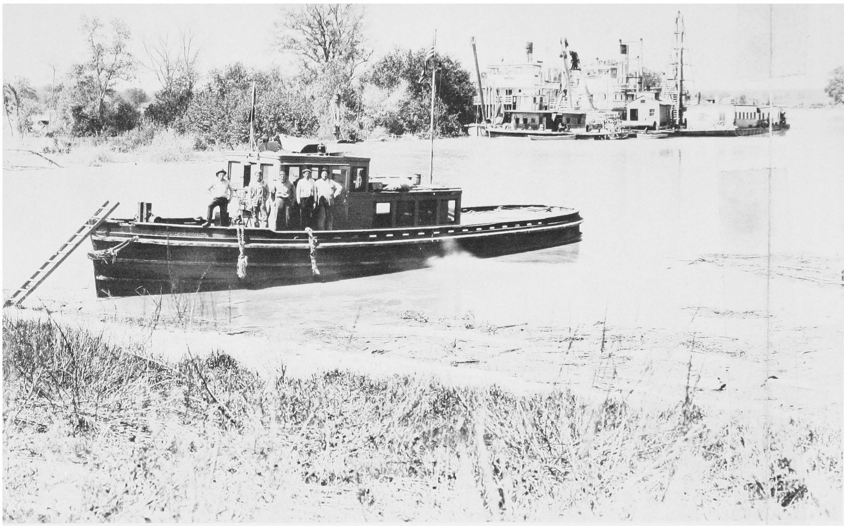
STOCKTON CHANNEL — APRIL 12, 1926 — DREDGE TENDER FALL , FOREGROUND. SNAG BOATS YUBA AND BEAR ALONGSIDE A PILE DRIVER, BACKGROUND. NOTE HOUSEBOATS ALONGSIDE; THIS IS WHERE THE CREWS LIVED.
