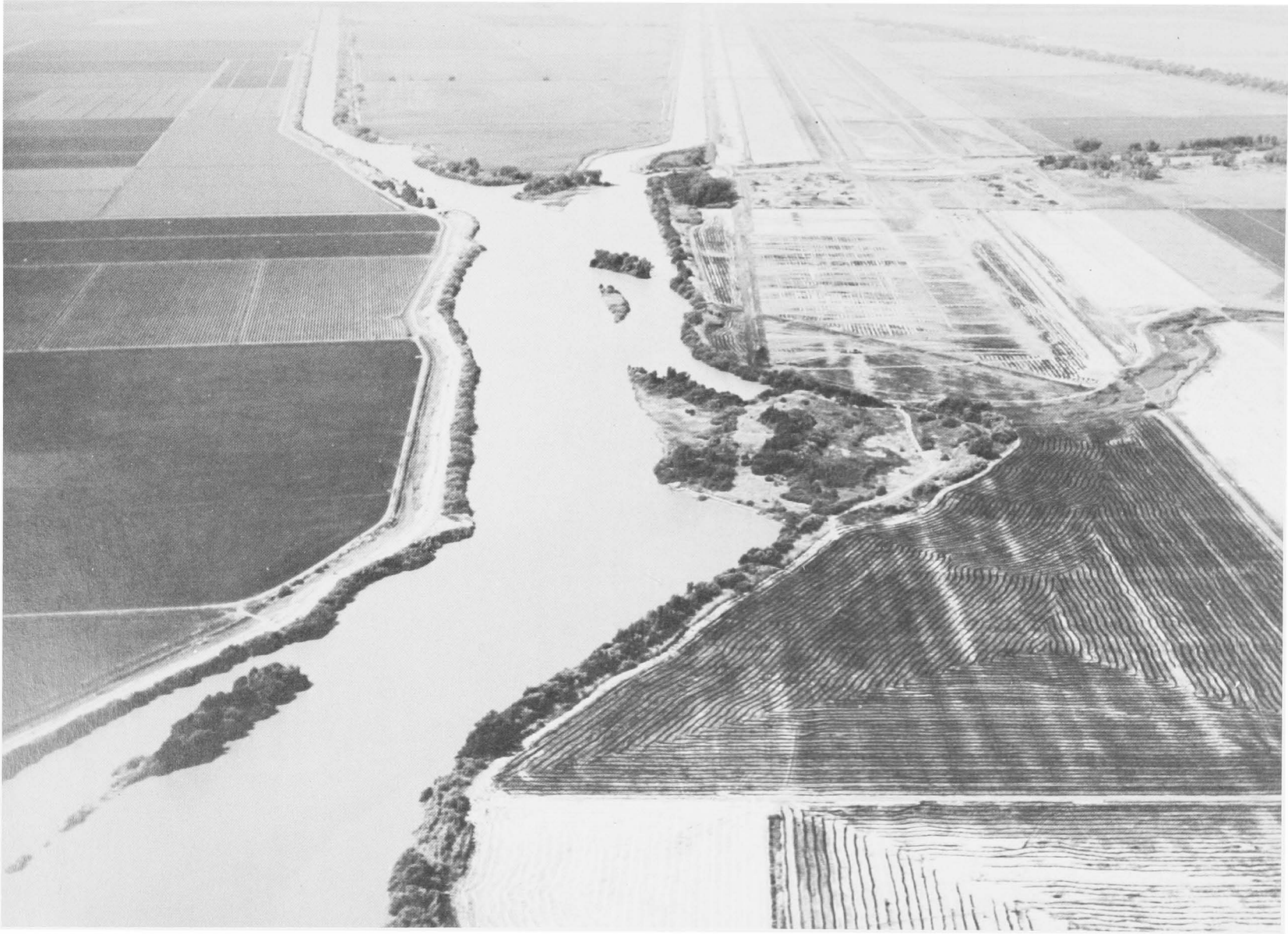
SACRAMENTO DEEP WATER CHANNEL, JULY, 1961 (Army Corps of Engineers Photo)
