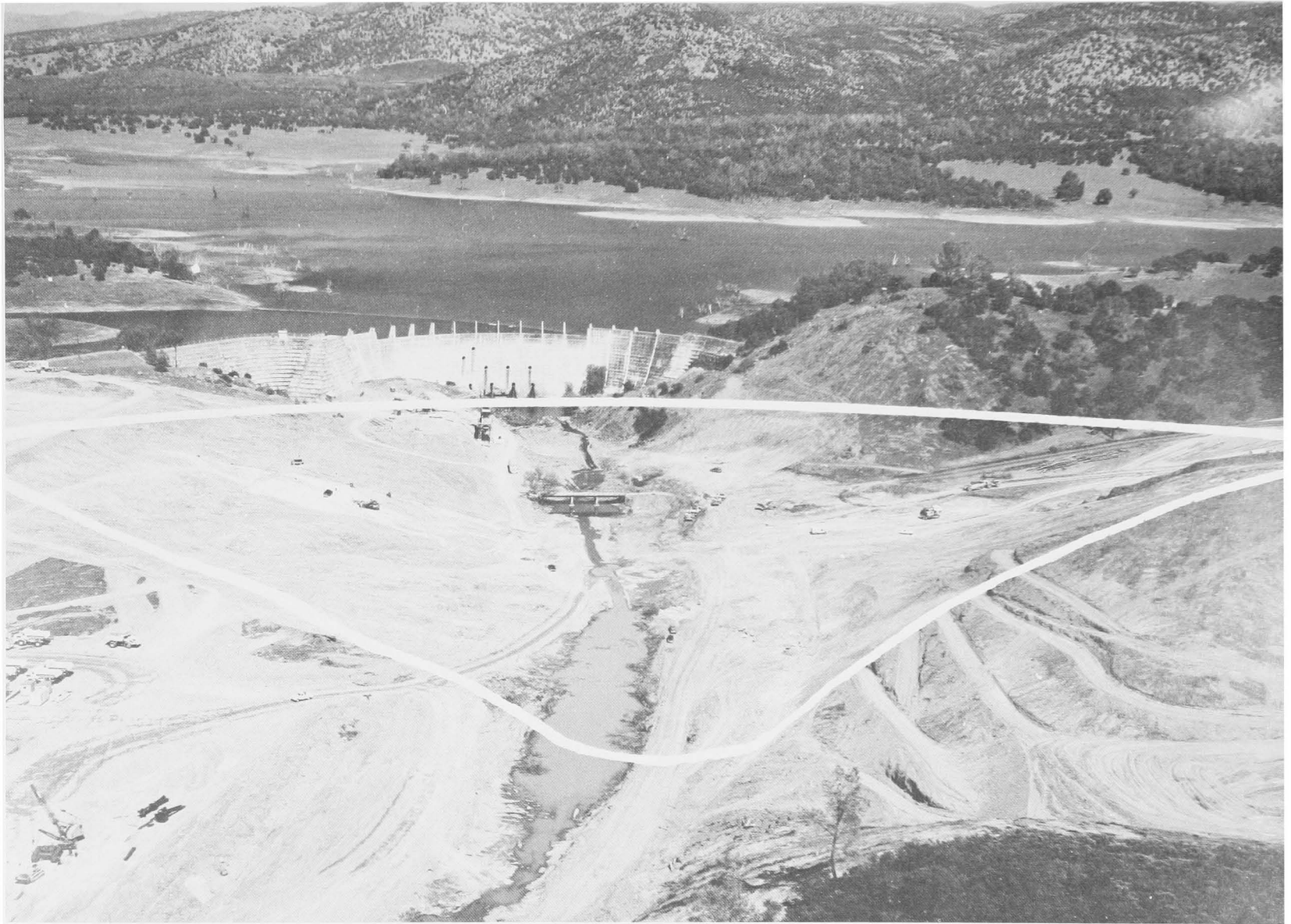
DRAWING SHOWS POSITION OF NEW HOGAN DAM UPON COMPLETION. THE OLD HOGAN DAM IS SEEN IN THE BACKGROUND. APRIL 1961.
