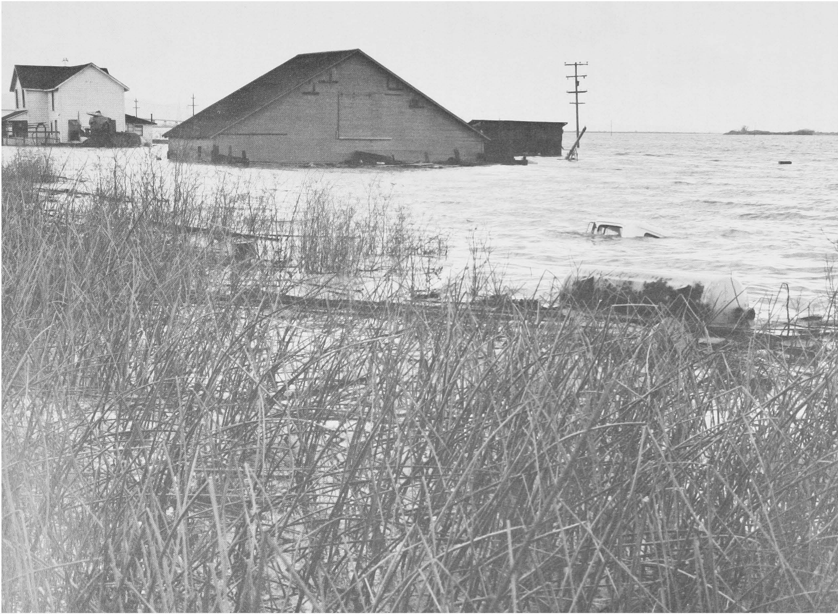
FARM FLOODED AT SHERMAN ISLAND — JANUARY 27, 1969
