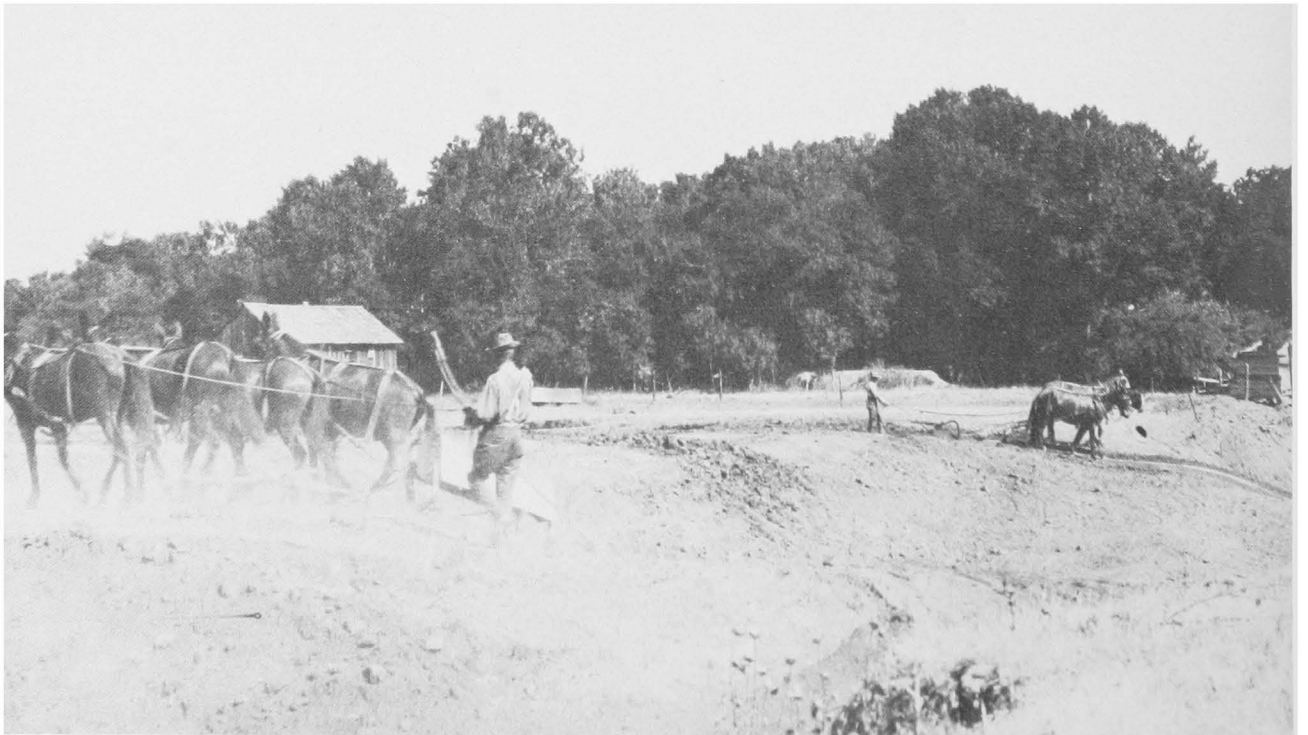
LEVEE CONSTRUCTION DURING THE EARLY DAYS, WITHIN THE SACRAMENTO DISTRICT, MEANT LONG DAYS AND A LOT OF MULE POWER. (National Archives Photos)
