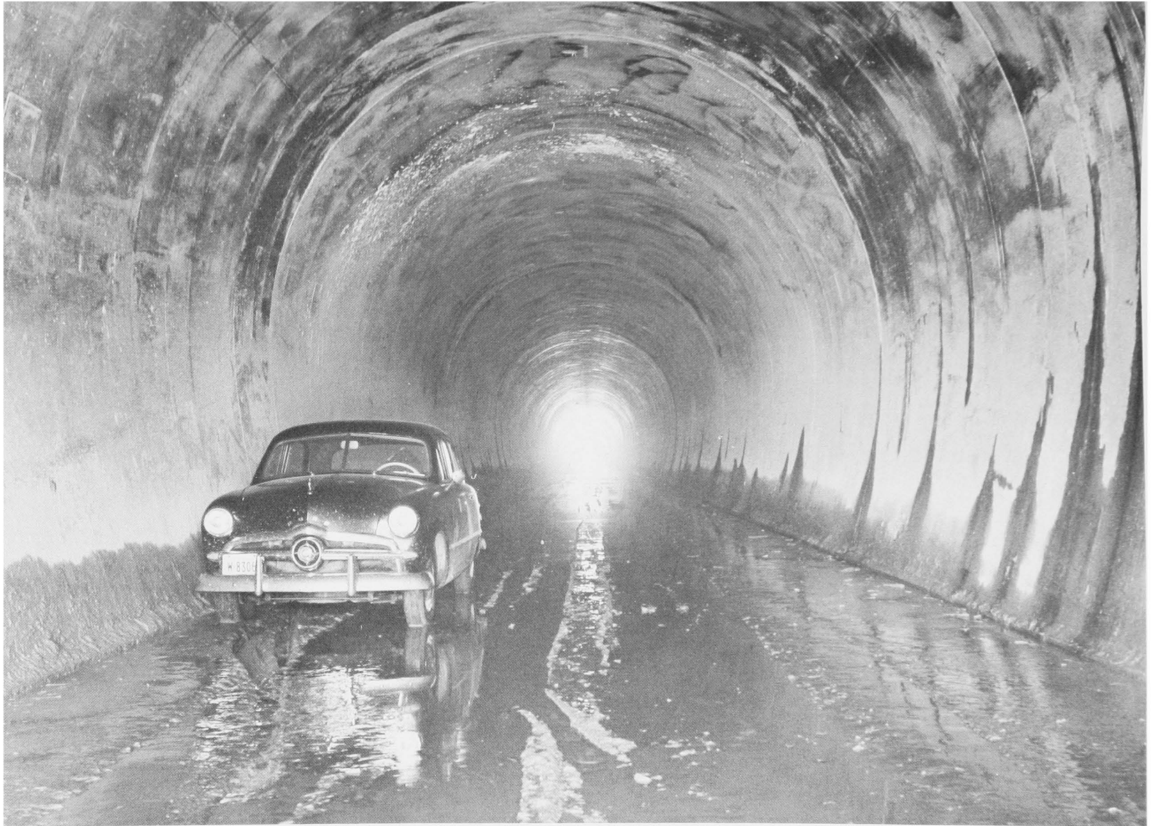
FOLSOM DAM PROJECT NEAR FOLSOM, CALIFORNIA. VIEW OF DIVERSION TUNNEL LOOKING DOWNSTREAM FROM STA. 6+55 ON RIGHT ABUTMENT OF MAIN DAM.
