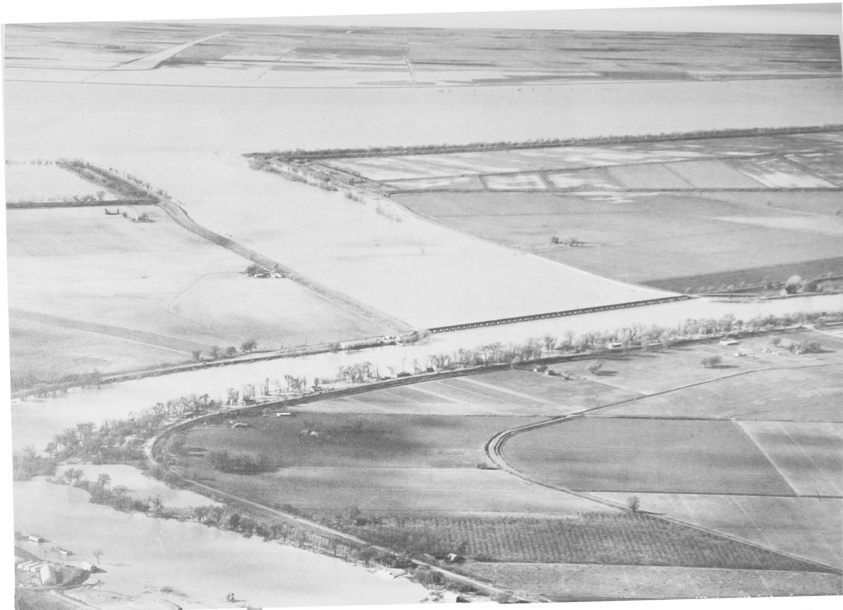
SACRAMENTO WEIR CONNECTING THE SWOLLEN SACRAMENTO RIVER WITH YOLO BYPASS — PHOTO TAKEN DECEMBER 1955. (Army Corps of Engineers Photo)
