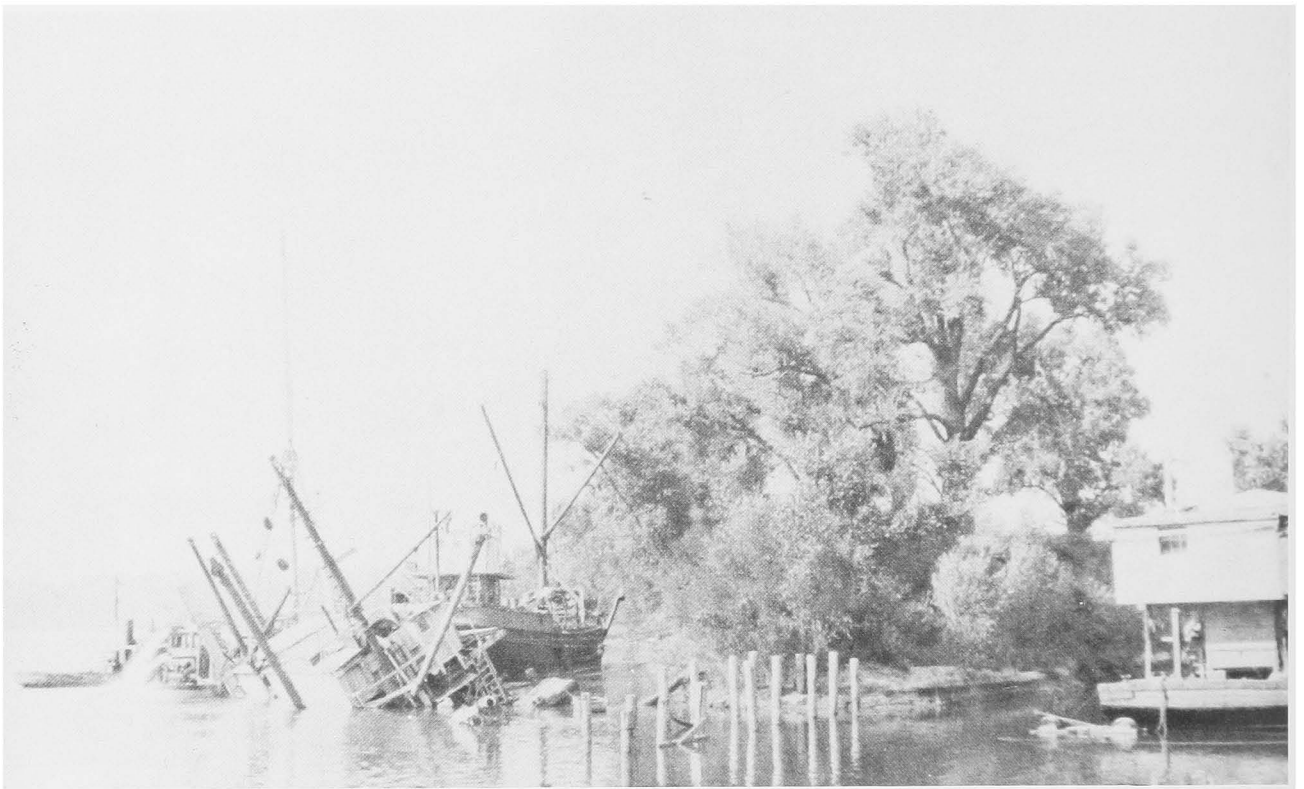
1929 — SAND DREDGER SUNK AT MOUTH OF AMERICAN RIVER.
