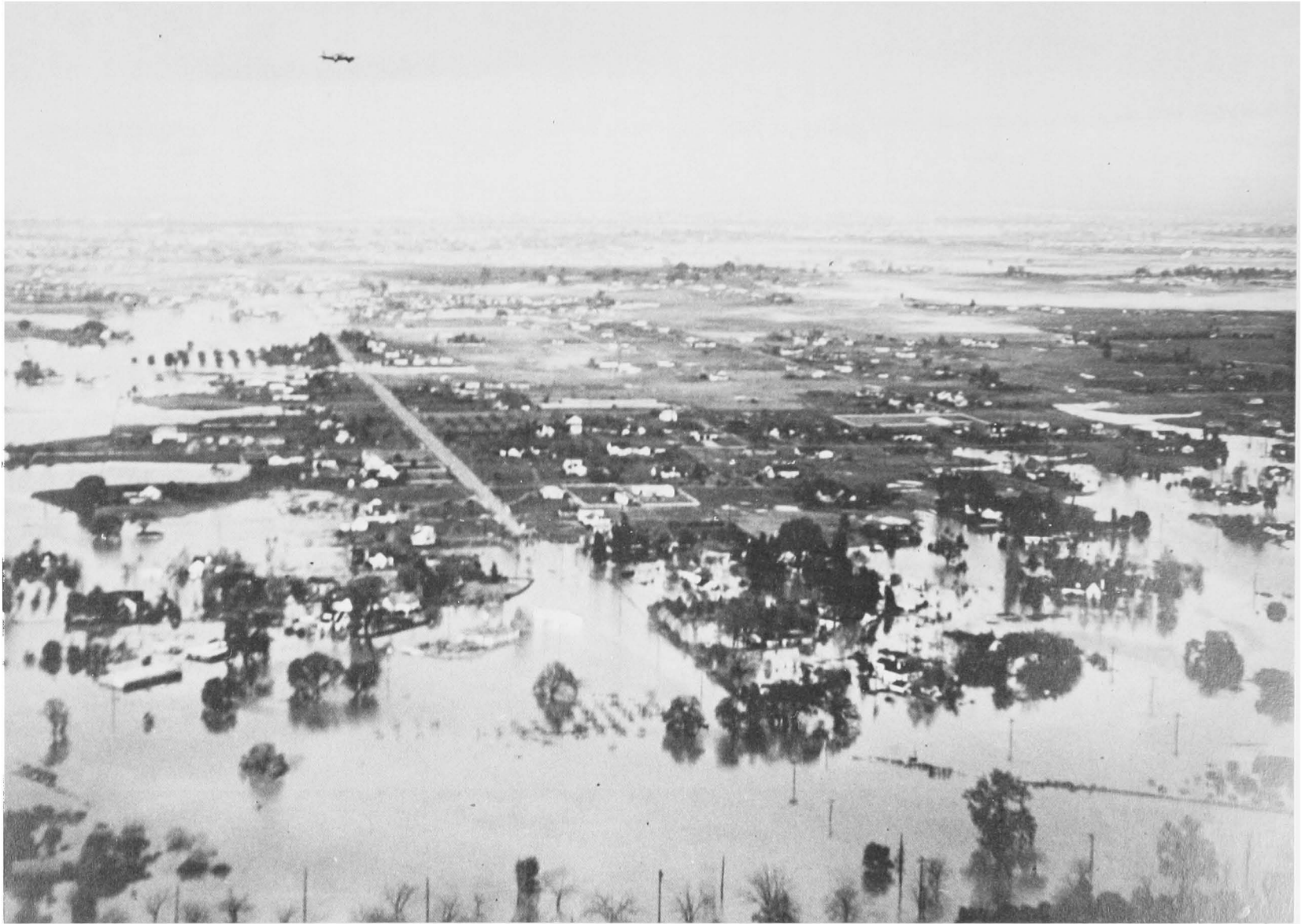
AMERICAN RIVER OVERFLOW. LOOKING NORTH ALONG FULTON AVENUE. NOVEMBER 1950. (Army Corps of Engineers Photo)
