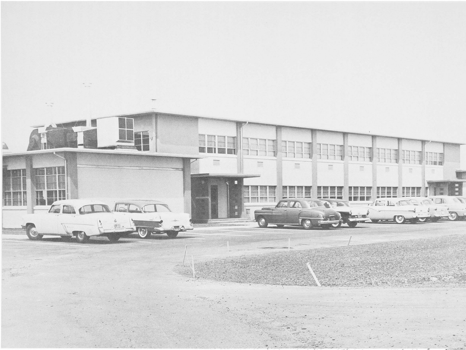
TRANSMITTER STATION NEAR DAVIS, CALIFORNIA (Photo courtesy Jack English)
