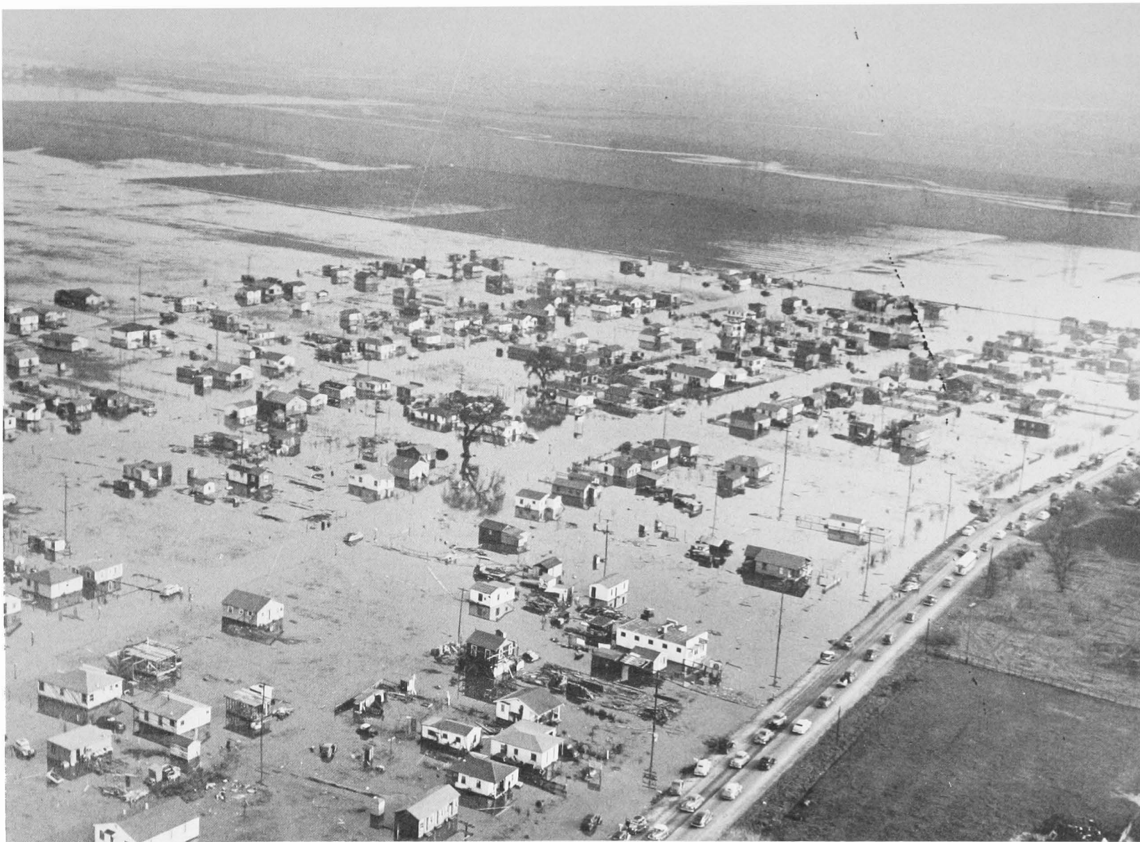
FLOODING BY DUCK CREEK IN VICINITY OF SHARP'S LANE, SOUTH OF STOCKTON. DECEMBER 1950.
