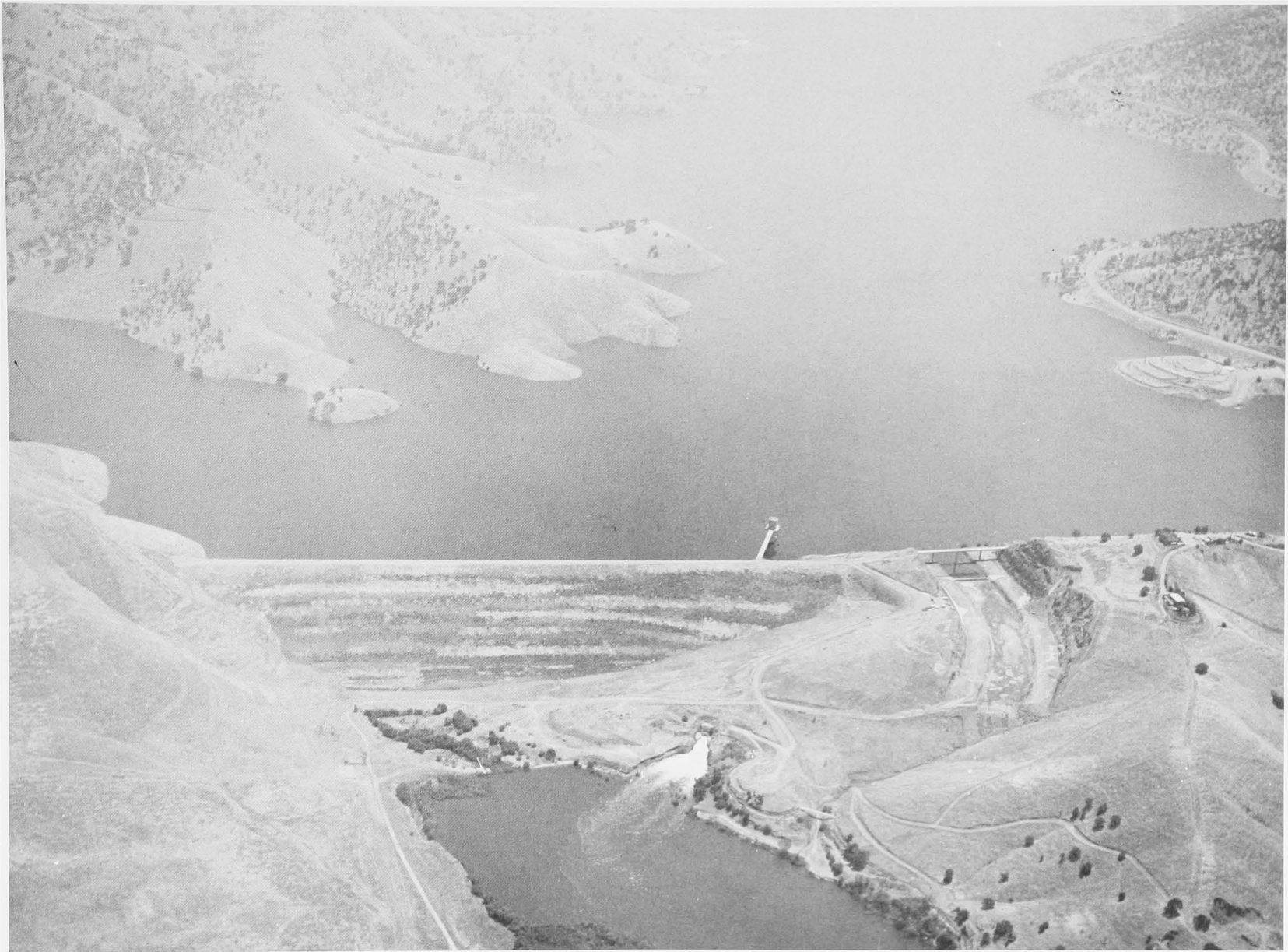
TERMINUS DAM AND LAKE KAWEAH (Army Corps of Engineers Photo)
