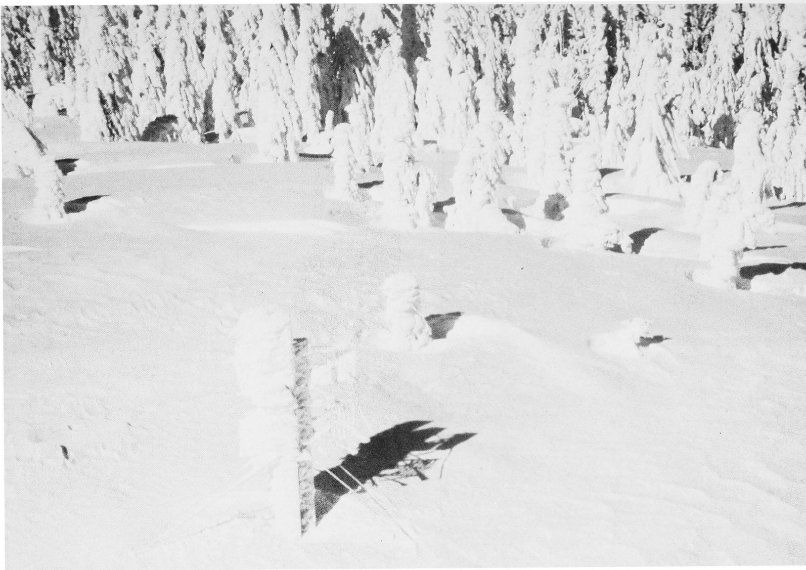
THE SHERMAN MOUNTAIN RADIO RELAY ANTENNA IN THE KERN RIVER BASIN 30 MILES SOUTHWEST OF MOUNT WHITNEY. ELEVATION HERE IS 10,000 FEET. THIS ANTENNA RELAYS SNOW WATER CONTENT INFORMATION GATHERED FROM SNOW PILLOWS TO THE ISABELLA DAM RECEIVING STATION.
