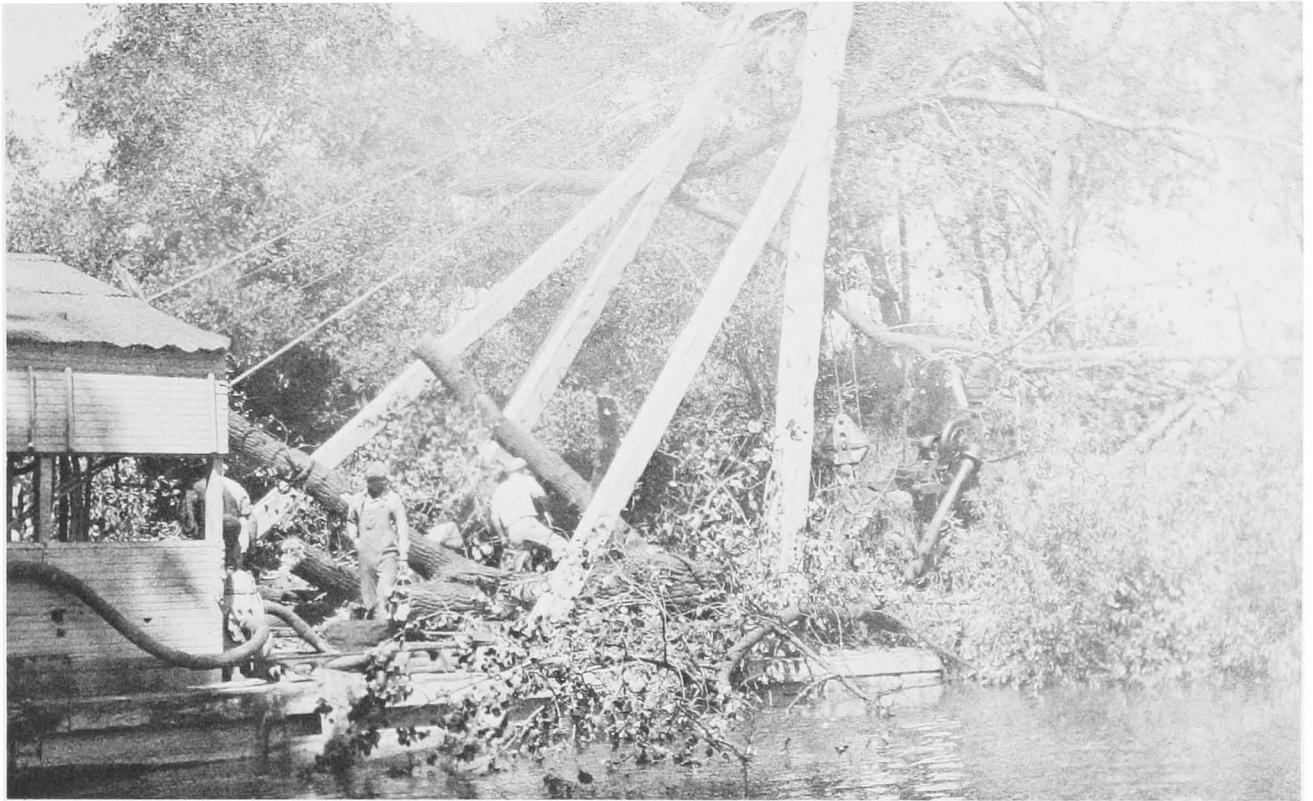
WHILE THE CONTROVERSY RAGED OVER DEBRIS DAMS AND DEEP WATER CHANNELS, SNAGGING OPERATIONS AND OTHER MAINTENANCE CHORES CONTINUED DURING THE 1930s.
