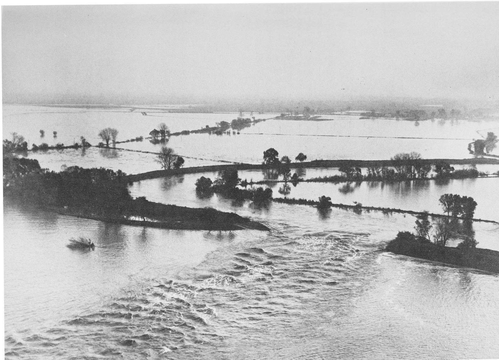
BREAK IN EAST LEVEE OF SAN JOAQUIN RIVER BELOW MOSSDALE. FLOODING OF RECLAMATION DISTRICT NO. 17 — DECEMBER 1950.
