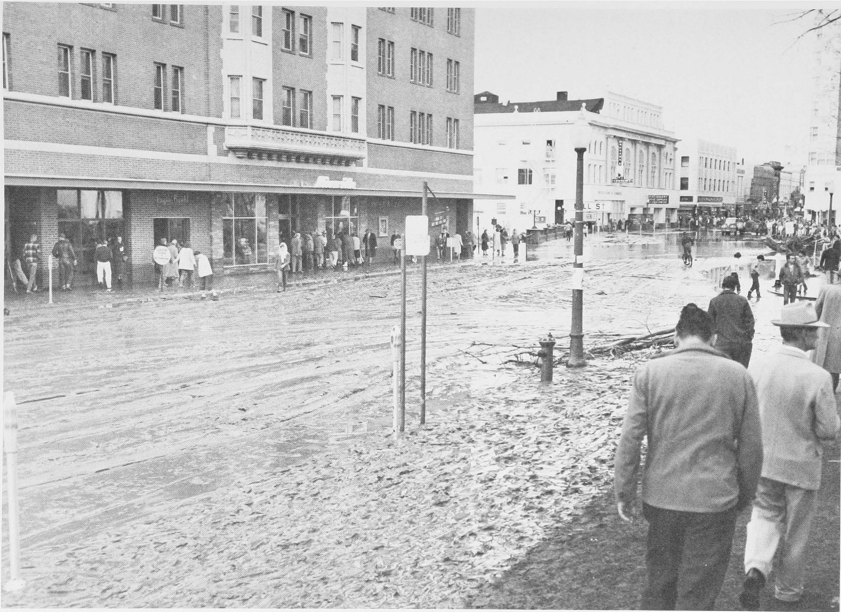
RENO, NEVADA, AFTER RECESSION OF TRUCKEE RIVER FLOODWATER. NOTE HIGH WATER MARK ON THE RIVERSIDE HOTEL. NOVEMBER 1950.
