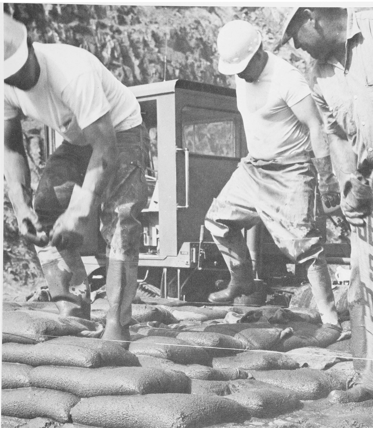
PLACING CONCRETE-FILLED SANDBAGS ACROSS THE LIP OF THE TERMINUS DAM SPILLWAY, THE SACRAMENTO DISTRICT, US ARMY CORPS OF ENGINEERS, GAINED ABOUT 10,000 ACRE-FEET OF ADDITIONAL STORAGE SPACE DURING THE RECORD SNOWPACK SNOWMELT OF JUNE 1969.
