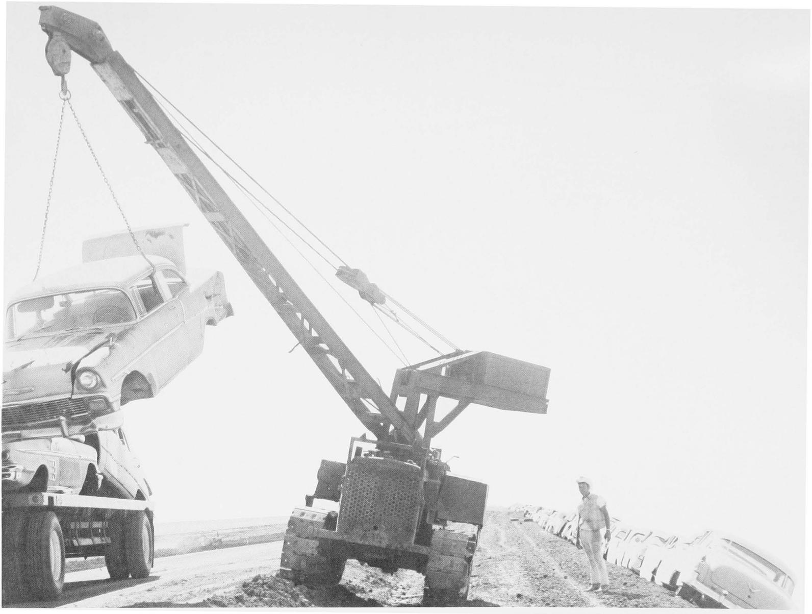
JUNK CARS ON THE LEVEE REDUCE EROSION FROM WINDBLOWN WAVES IN THE TULARE LAKE BASIN WHERE THOUSANDS OF ACRES WERE FLOODED BECAUSE OF THE RECORD SNOWFALL AND RAINFLOODS IN THE REGION. APRIL 1969.
