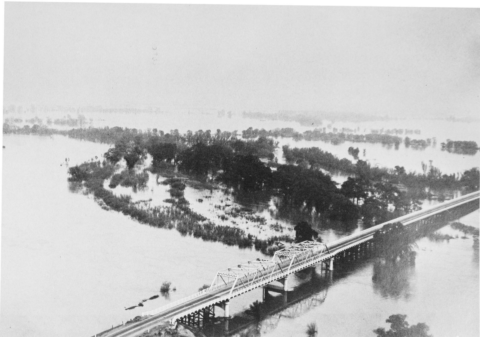
MAZE ROAD BRIDGE OVER SAN JOAQUIN RIVER BETWEEN TUOLUMNE AND STANISLAUS RIVERS. VIEW LOOKING NORTHEAST. DECEMBER — 1950.
